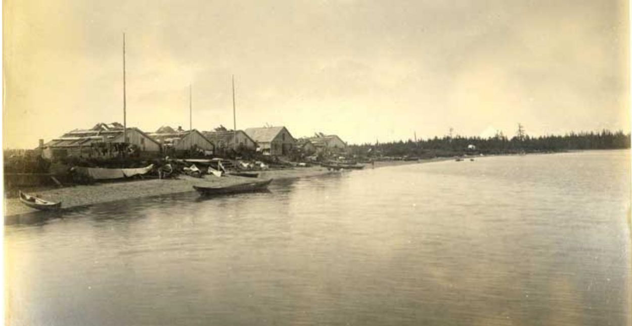
Figure 1 – The village of S'oooska, or Port Mulgrave, across the water from the modern Yakutat shoreline. This village served as the winter settlement for Yaakwdáat Kwáan prior to the consolidation of settlement in the village of Yakutat in the late 19 th and early 20 th centuries. Photo courtesy Yakutat Tlingit Tribe/Bert Adams Sr.
