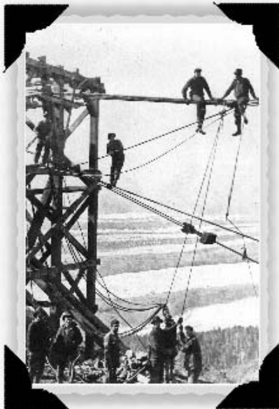
8 Working on the Bonanza tramline.
