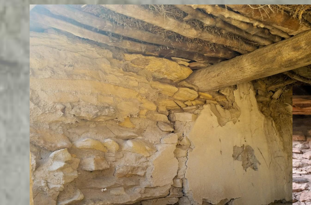
The masonry construction from a room at Hopi.
