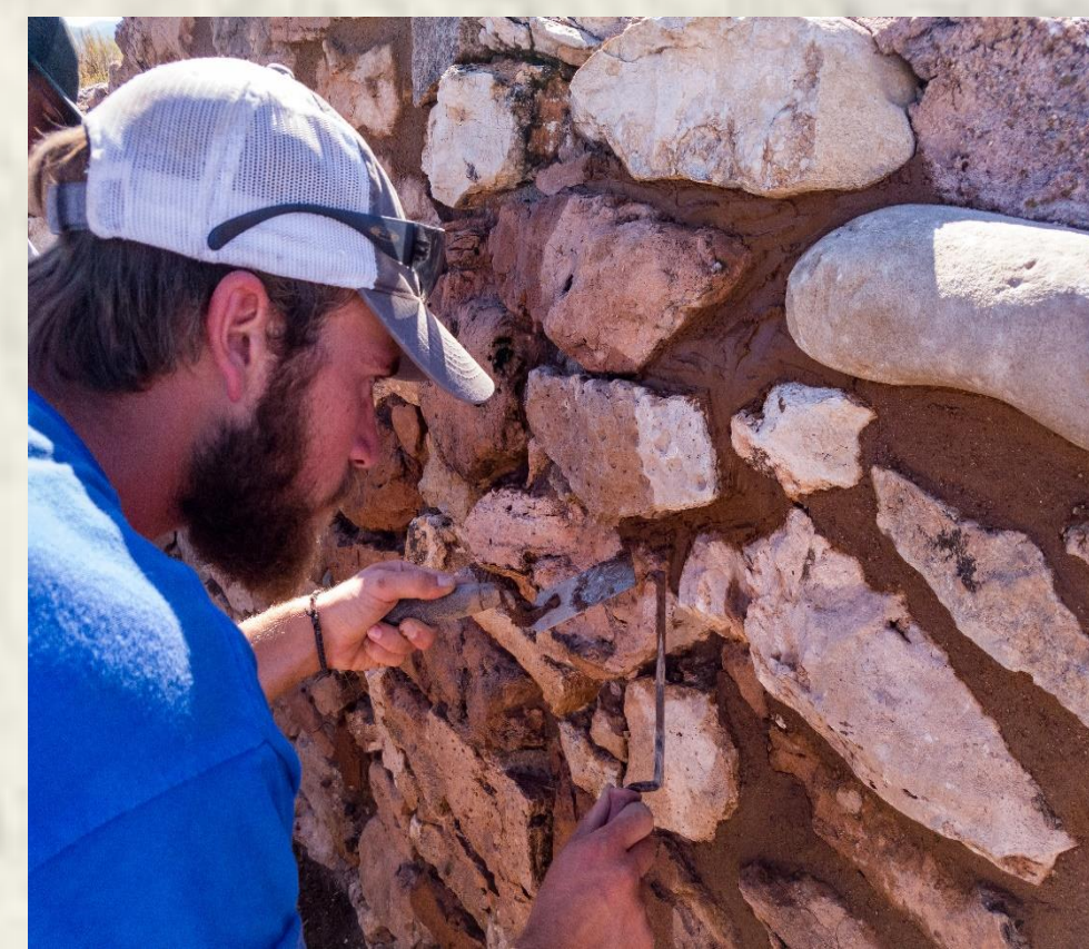
During stabilization using the technique of tuck pointing.
