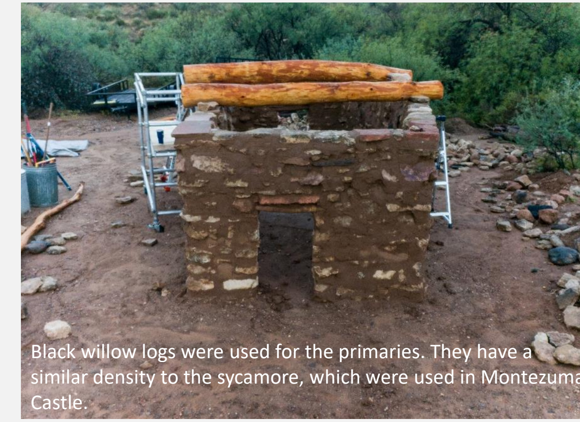
Black willow logs were used for the primaries. They have a similar density to the sycamore, which were used in Montezuma Castle.
