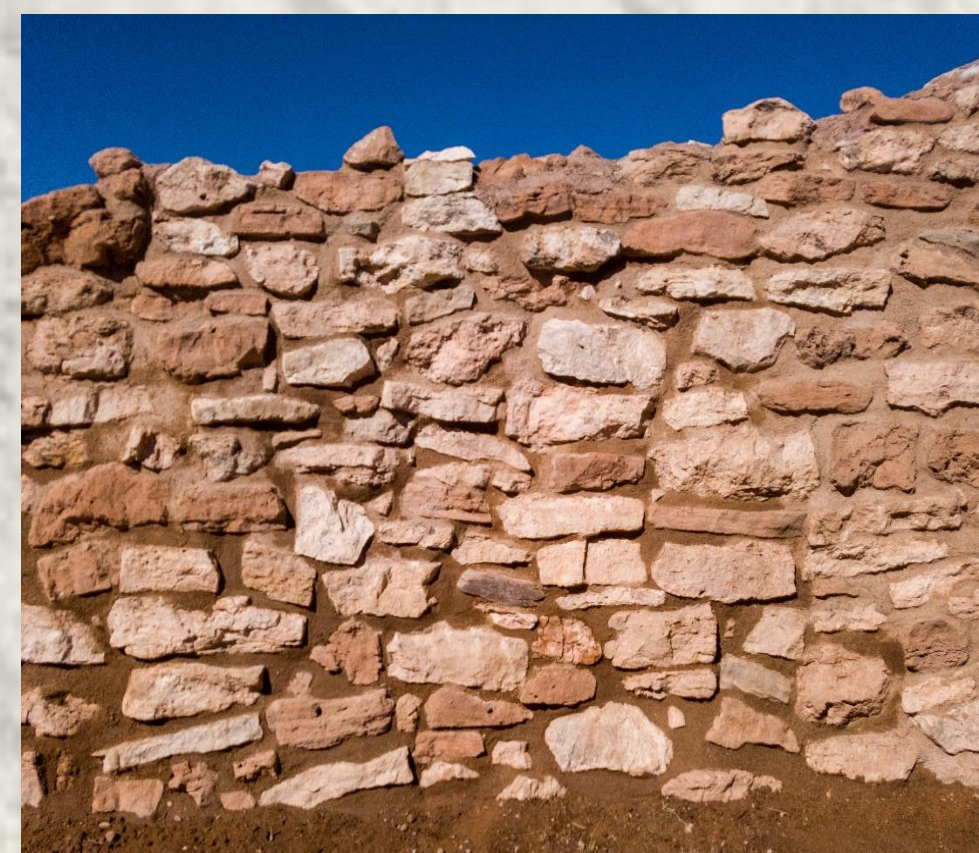
After stabilization using the current mortar mix at Tuzigoot National Monument.
