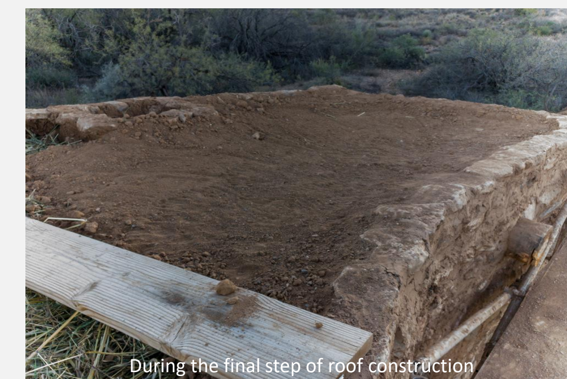
During the final step of roof construction.
