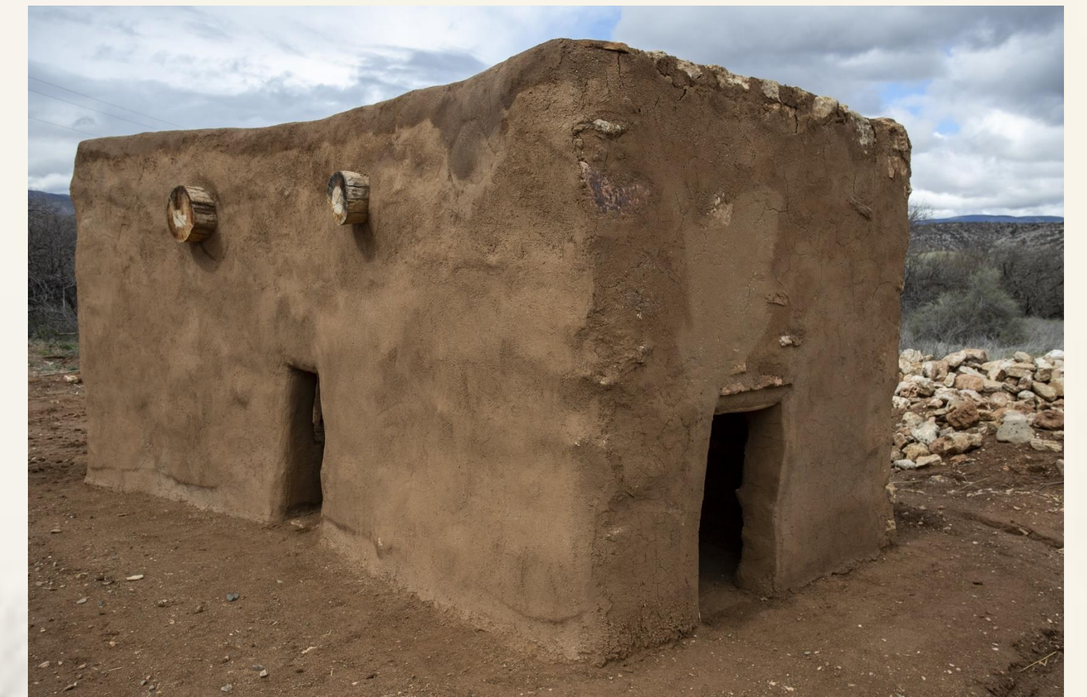
After the final layer of finishing plaster was applied.
