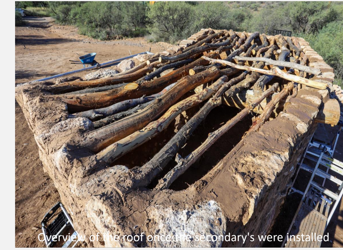
Overview of the roof beams. The secondary's were installed.
