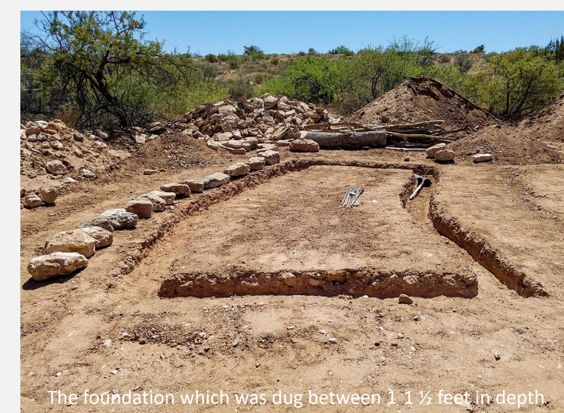
The foundation which was dug between 1-1 1/2 feet in depth.
