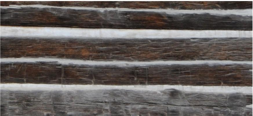
**Problem:** Large-scale Failure of Chinking and Daubing. Advanced deterioration has made the chinking and daubing unattractive and unable to repel wind and water.
