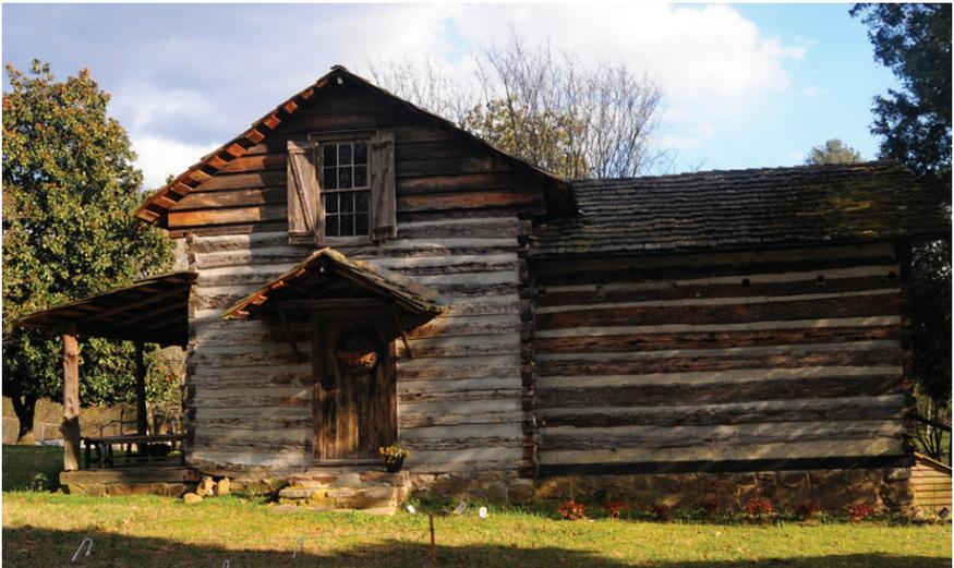
Log structures in warm climates were set on piers in order to allow air to circulate underneath. This air circulation kept the house cooler and helped keep wooden components (particularly sills and joists) from rotting. If infill was added between the piers air circulation decreased, making deterioration of the sills, joists, and lower logs more likely.
