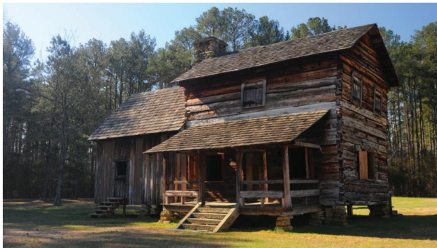
*Cherokee James Vann built this two-story hand-hewn log tavern around 1805. It has a single room on the first floor and three rooms on the second floor accessible by an external staircase at the rear. A one-story board-and-batten room was added to the east side at a later date. The tavern was moved to the New Echota State Historic Site in Gordon County, Georgia, in 1955.*
