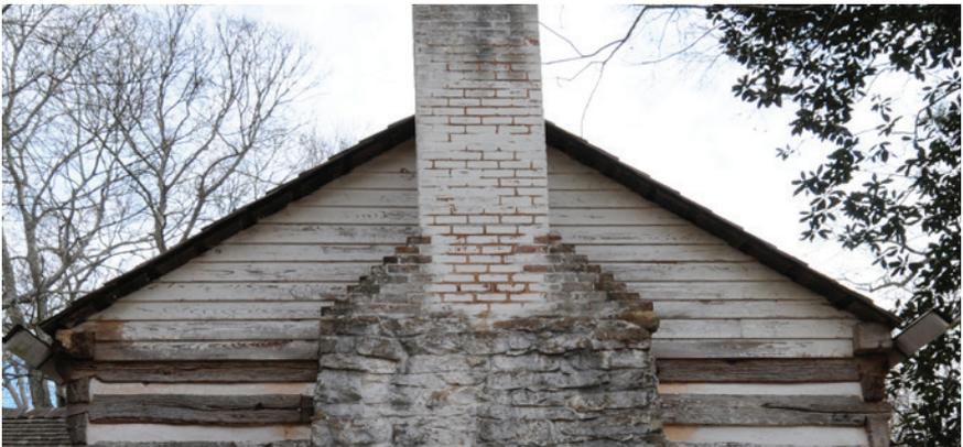
**Problem:** Removal of Siding to Expose Logs. The majority of the structure's historic siding is removed for an "old-timey" appearance. This all-too-common practice can be extremely deleterious to the logs themselves and other historic building materials. Because the purpose of the siding was to protect the logs, chinking, and daubing, its removal allows deterioration to begin and continue.
