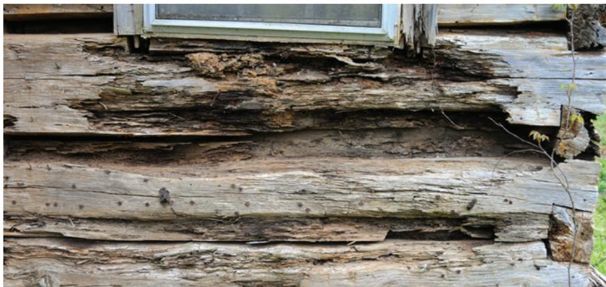
**Problem:** Minor Deterioration of Log. Deterioration of wall logs, particularly lower logs and logs near fireplaces, is not unusual. Although some species of wood, such as red cedar and yellow poplar, are highly resistant to decay, all wood will rot eventually.
