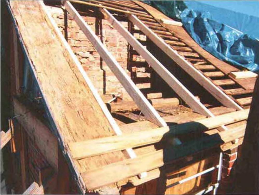
*Replacement rafters and two new sheathing boards installed at the southwest corner of the ell roof.*
