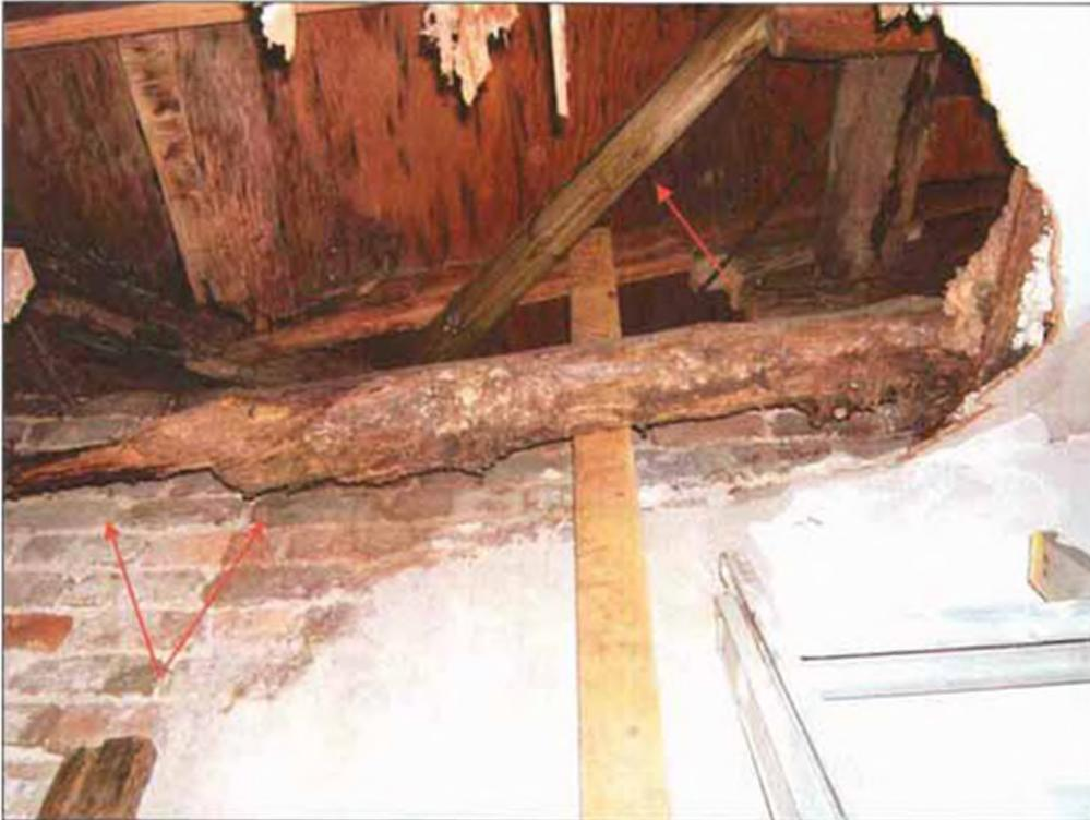
*Once lifted back into position, the temporary rafter was braced with a 4x4 cross beam as shown in this photograph. Note the extent of the deterioration to the original log rafter that once supported the rear porch of the house.*
