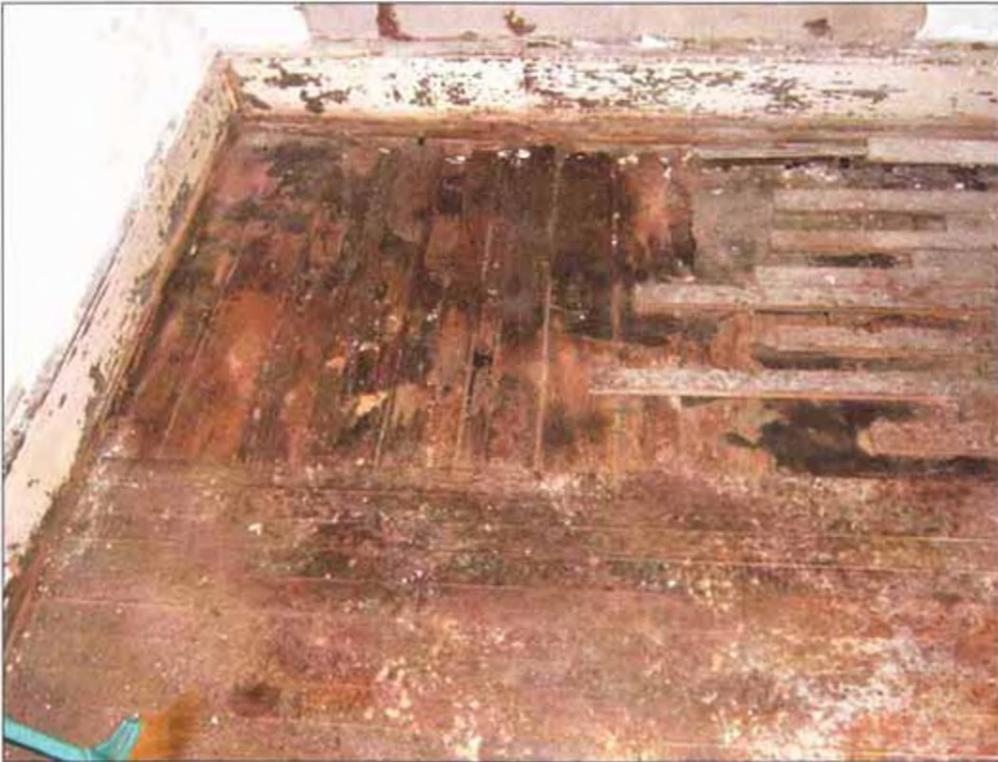
*Southeast corner of room 103 where water intrusion into this area of the James Brown House has deteriorated the floor to the point of collapse. This photograph shows the original floor boards of the room beneath the removed modern hardwood flooring.*
