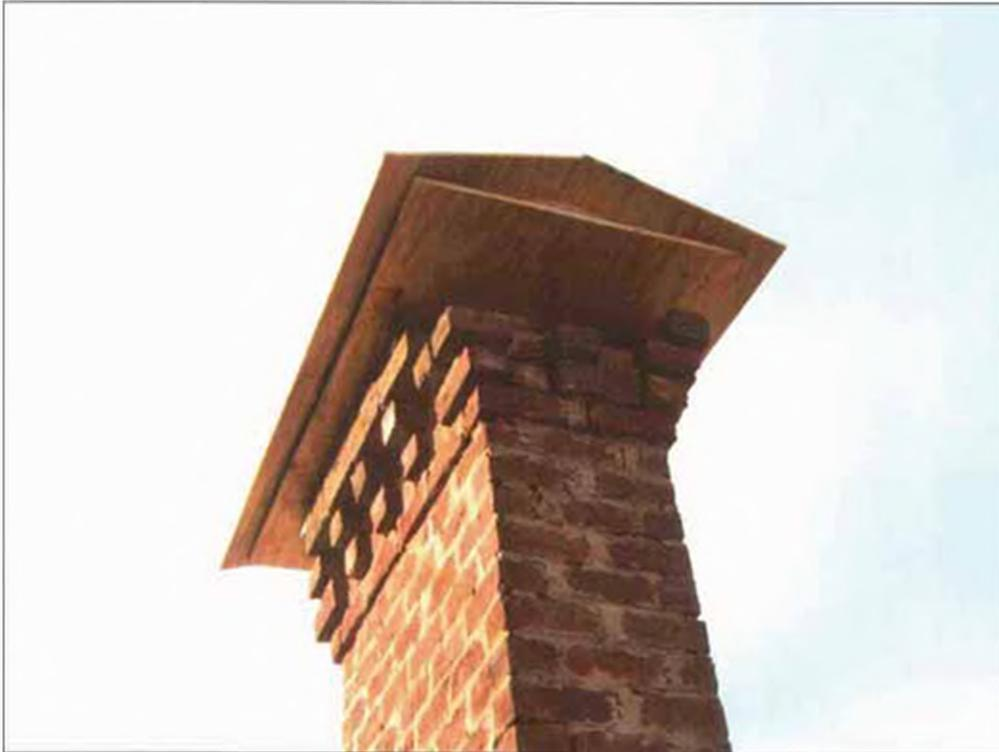
*Detail of temporary wood chimney cap which sits down partially within the flue of the chimney.*
