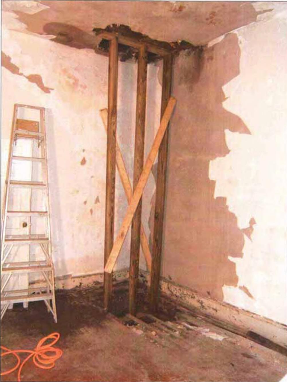
*Temporary support wall constructed to carry the load from the broken ceiling beam down to grade. No attempt was made to lift the beam back into position as this no doubt would have transferred undue stresses to other members of the house. Instead by stabilizing the detached beam, the mechanisms of deterioration in this area of the structure can be more fully assessed and a comprehensive repair of the failed elements can be undertaken when funding permits.*
