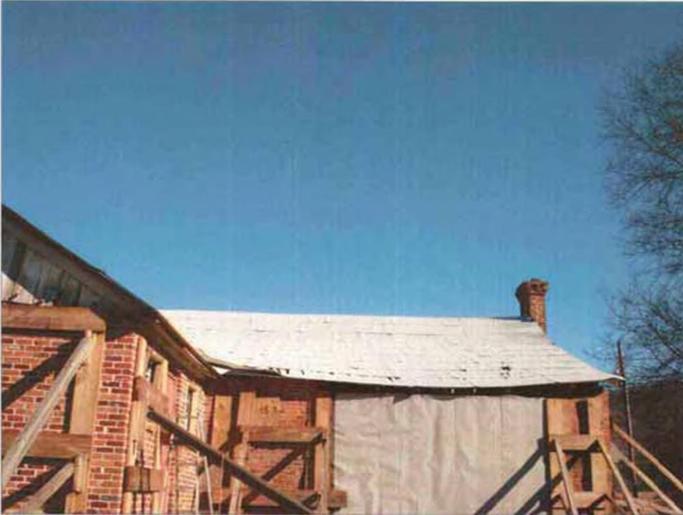
*Detail of roll roofing installed at west side of house. The buckling of the roll roofing, which could not be avoided, is due to the application of the material over the underlying roof deck, which though stabilized remains uneven. Photo courtesy of Scott Smith.*
