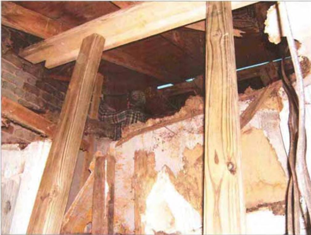
*Volunteer carpenter Richard Bond make repairs to the rafters from within the house prior to repairing sheathing in the lower valley area of the roof at the west side of the James Brown House. Note 4x4 posts and 2x6 brace( in foreground of photograph) installed beneath 2x6 rafters which had become dislodged and where lifting up roof sheathing at the back of the house.*
