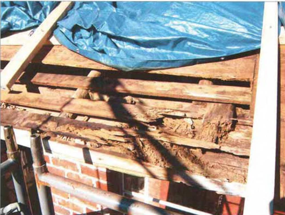
*Detail of extensive termite damage and rot found at the eaves on the south side of the ell roof.*
