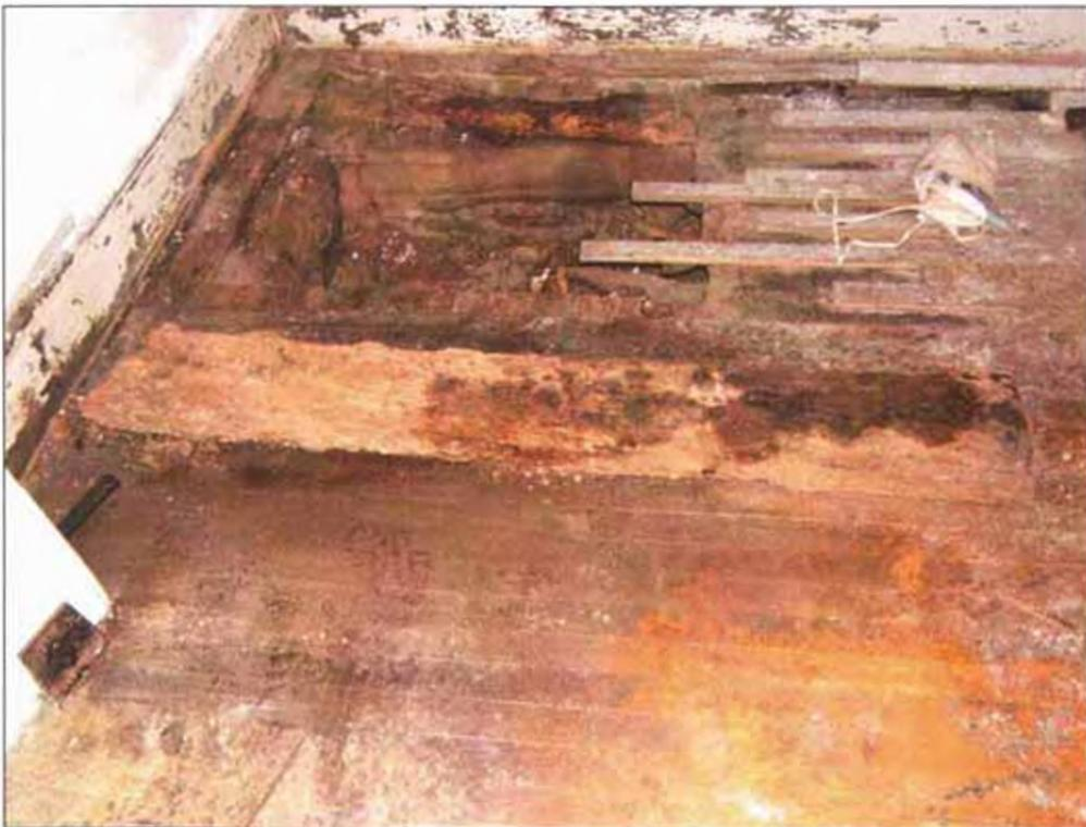
*Southeast corner of room 103 showing removed broken log joist in foreground of photograph. Note the wet condition of the joist as well as the joist still intact along the foundation of the south wall of the room.*
