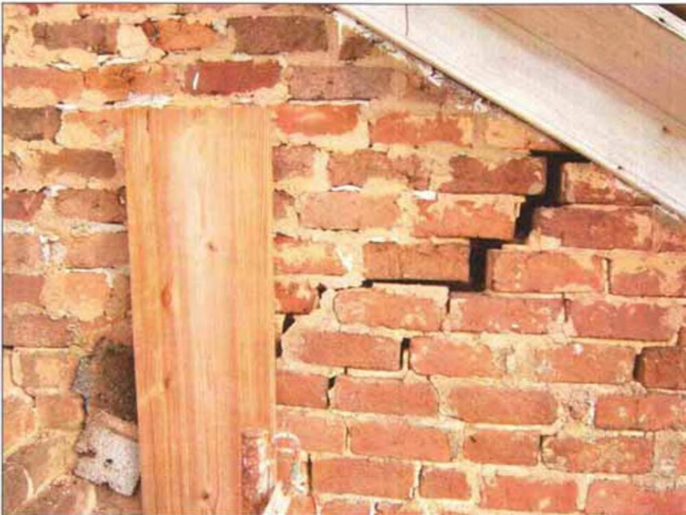
*Detail of gable wall east of south chimney in need of repointing to temporarily keep water and insects from entering the structure.*
