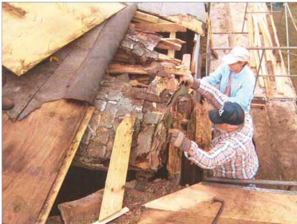
*Volunteers installing edge flashing at eave of ell roof after repairs to deteriorated sections of roof sheathing and underlying materials.*
