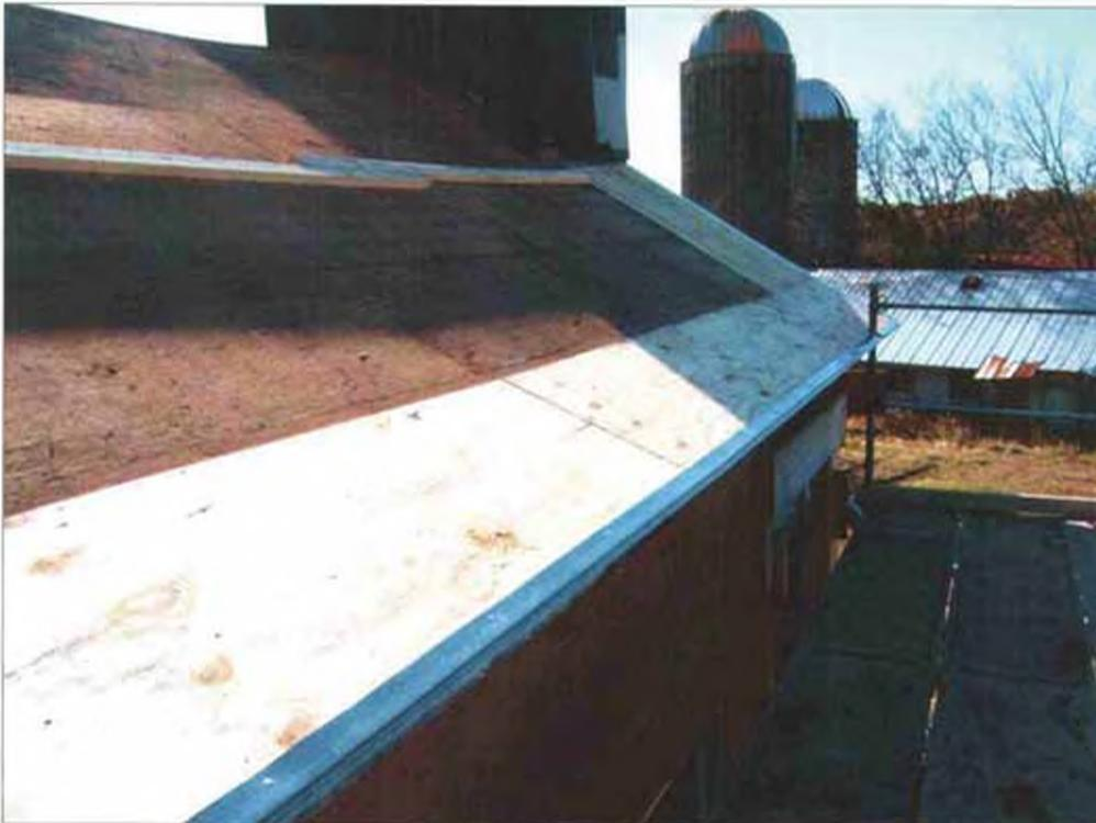
*Repairs to sheathing at eave and rake on north side of ell prior to reproofing with 90# roll roofing and 15# felt.*
