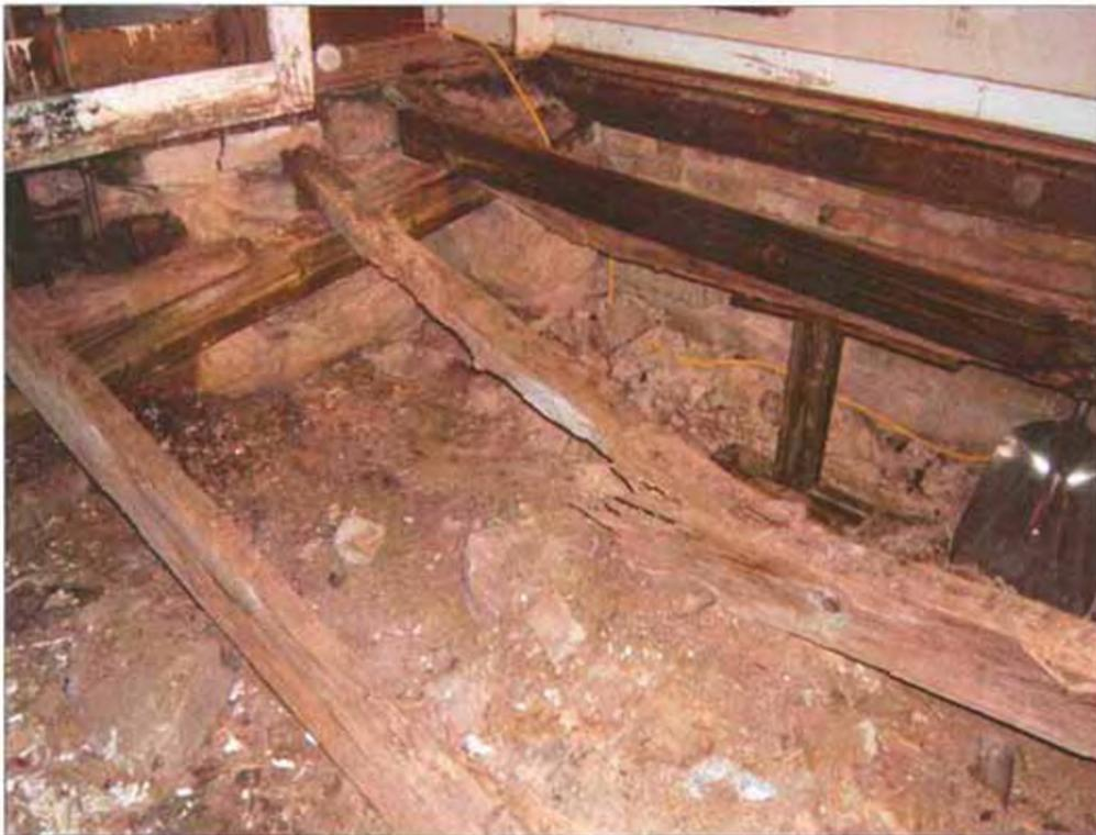
*Stabilized original rear porch floor joists and girder located in room 105 of the James Brown House to allow for future architectural investigation of the structure. It should be noted that an archeological investigation of the space should also be undertaken in the future.*
