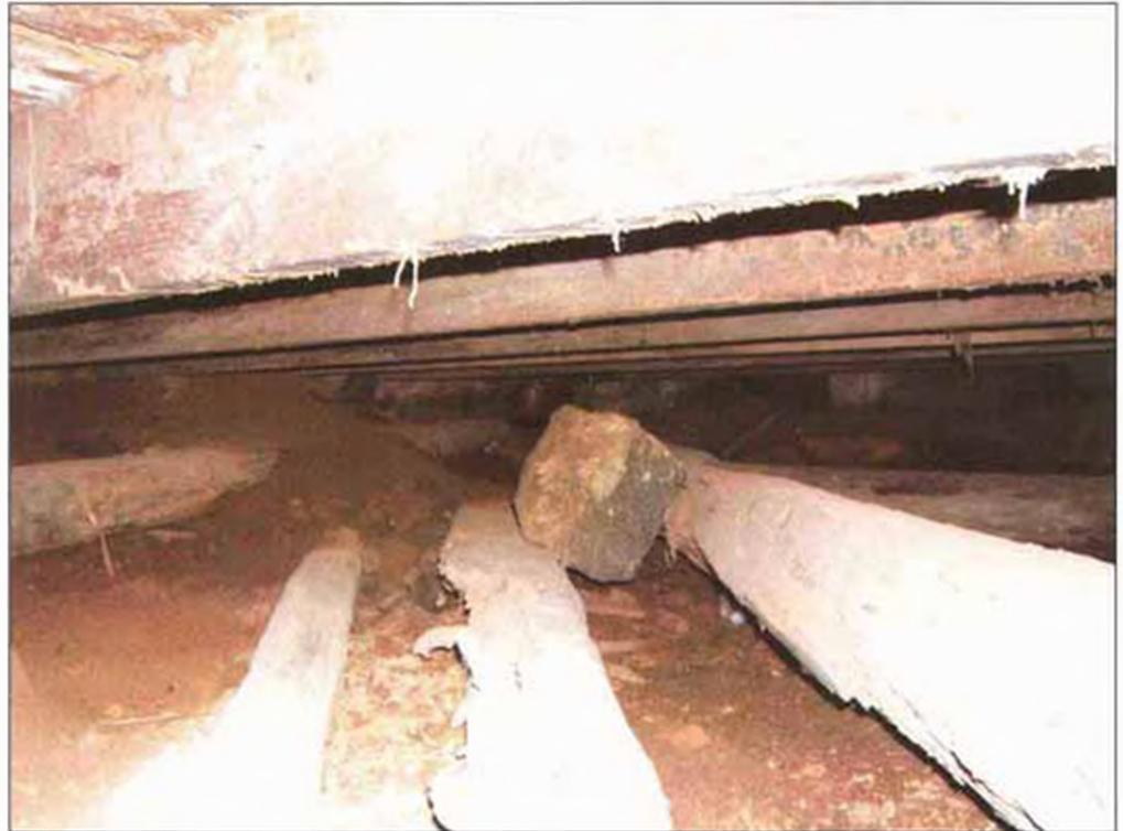
*Detail of crawl space beneath room 103 showing hewn logs sitting on grade, which may be remnants from earlier log structure located on the site.*
