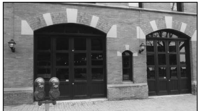
The design of the replacement doors is articulated with multi-paned units, maintaining the historic character of the building.
