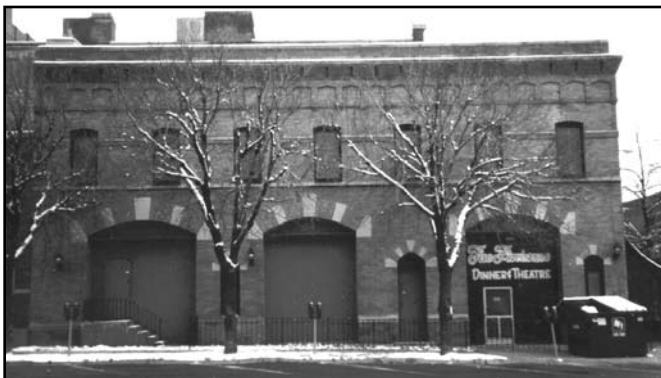
The south elevation of the 1903 firehouse is dominated by three large garage door openings. This photo was taken just prior to rehab and shows the existing infill treatments.
