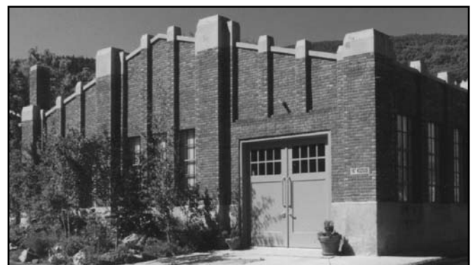
The owner chose to duplicate the original garage doors. The new doors preserved the industrial character of the historic building.
