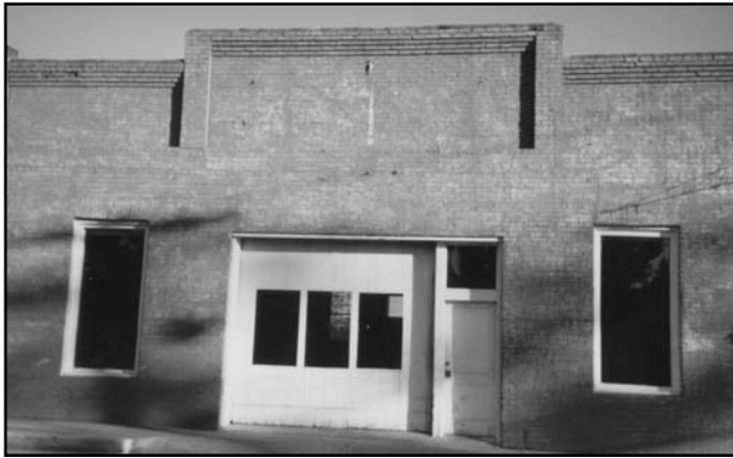
Before the work began, the original 1930 garage door opening had an operable garage door and a pedestrian door surmounted by a glazed transom installed as infill.
