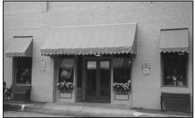
During rehabilitation the owner infilled the garage door opening with a storefront reminiscent of those used in the early-20 th century, which is not in keeping with the historic character of the building.
