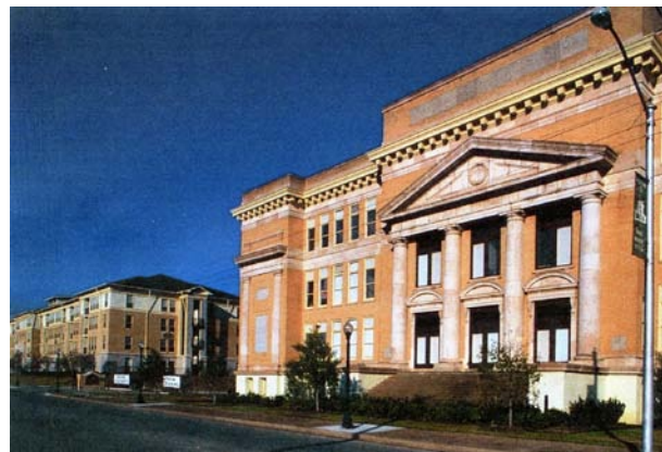
Historic school buildings are commonly rehabilitated for multi-family housing. This often requires more space and, consequently, new construction, such as the building shown here, which is compatible with the historic school and its site
