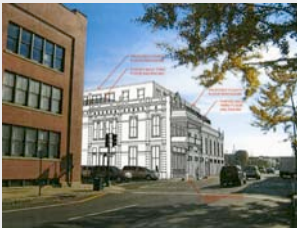
The rehabilitation proposal is to recreate the historic appearance, while adding a two-story rooftop penthouse. This did not meet Standards 3 & 9. It would have given the building a false sense of history and adding a two-story rooftop addition to a low-rise building is generally not a compatible treatment.
