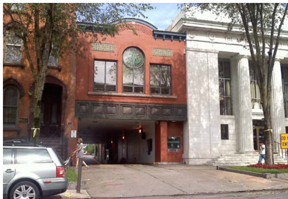
This new addition, which features a drive-through teller window, to a historic Classical Revival-style bank was designed to appear as a compatible infill structure, rather than an addition to the bank.
