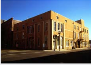
The building as it appeared prior to the proposed rehabilitation: Originally constructed in the 19th century, it housed an undertaker's establishment, livery stables and, most recently, a coffee warehouse.
