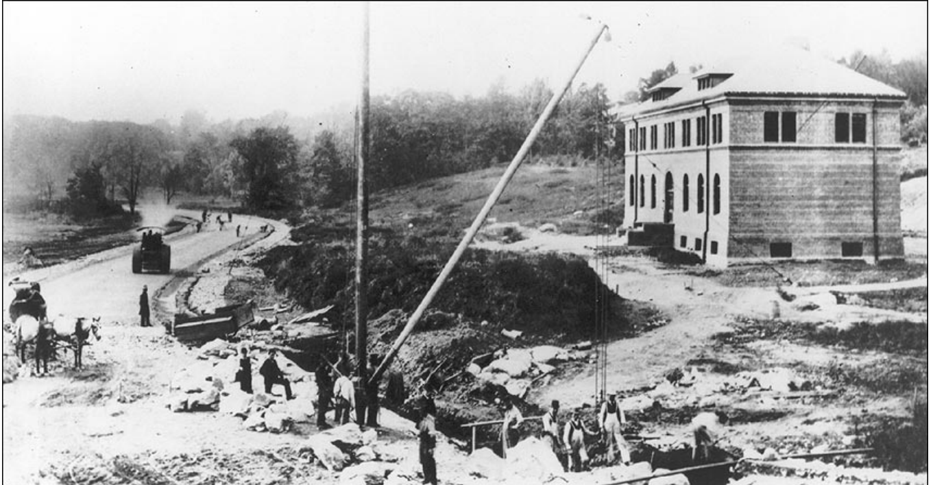
Photo 1: Construction near main entrance on Meadow Road, c. 1892
