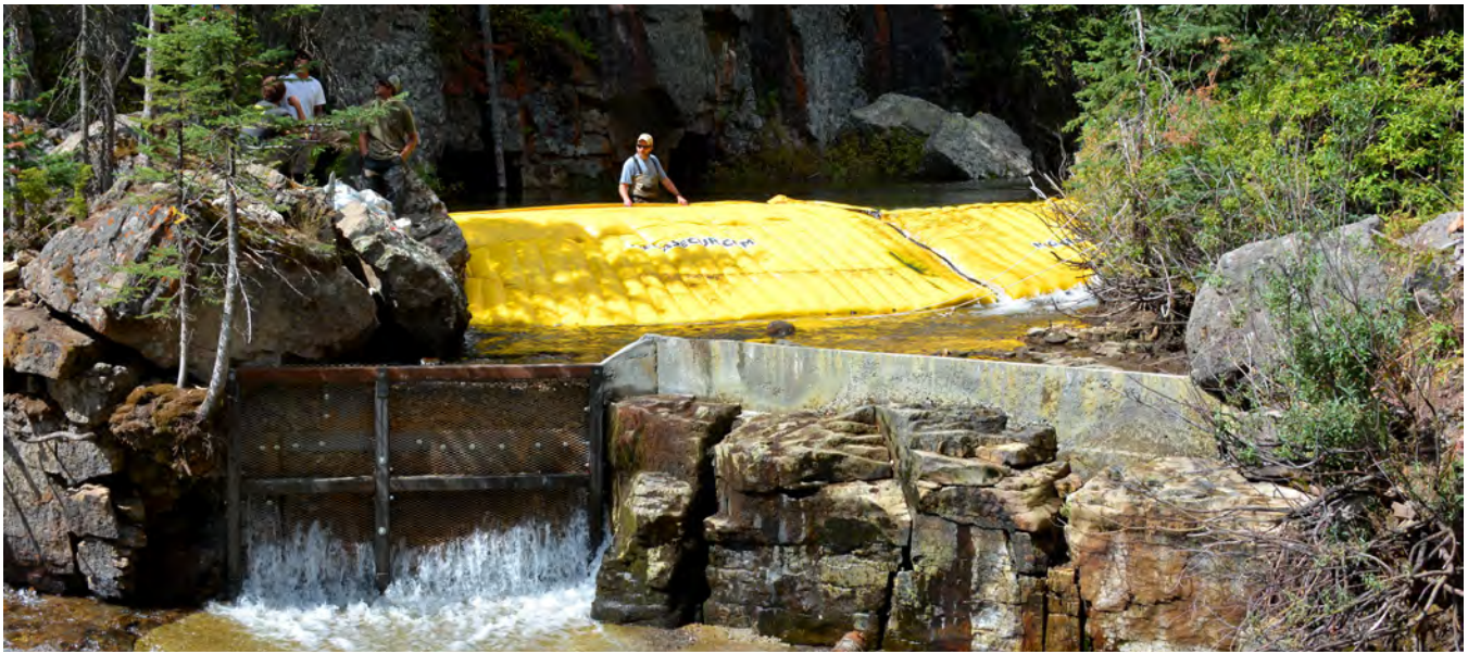
An existing waterfall was modified on lower Grayling Creek watershed to provide a complete barrier to upstream fish movement. The large yellow structure temporarily diverted the stream and was removed after construction was completed.
