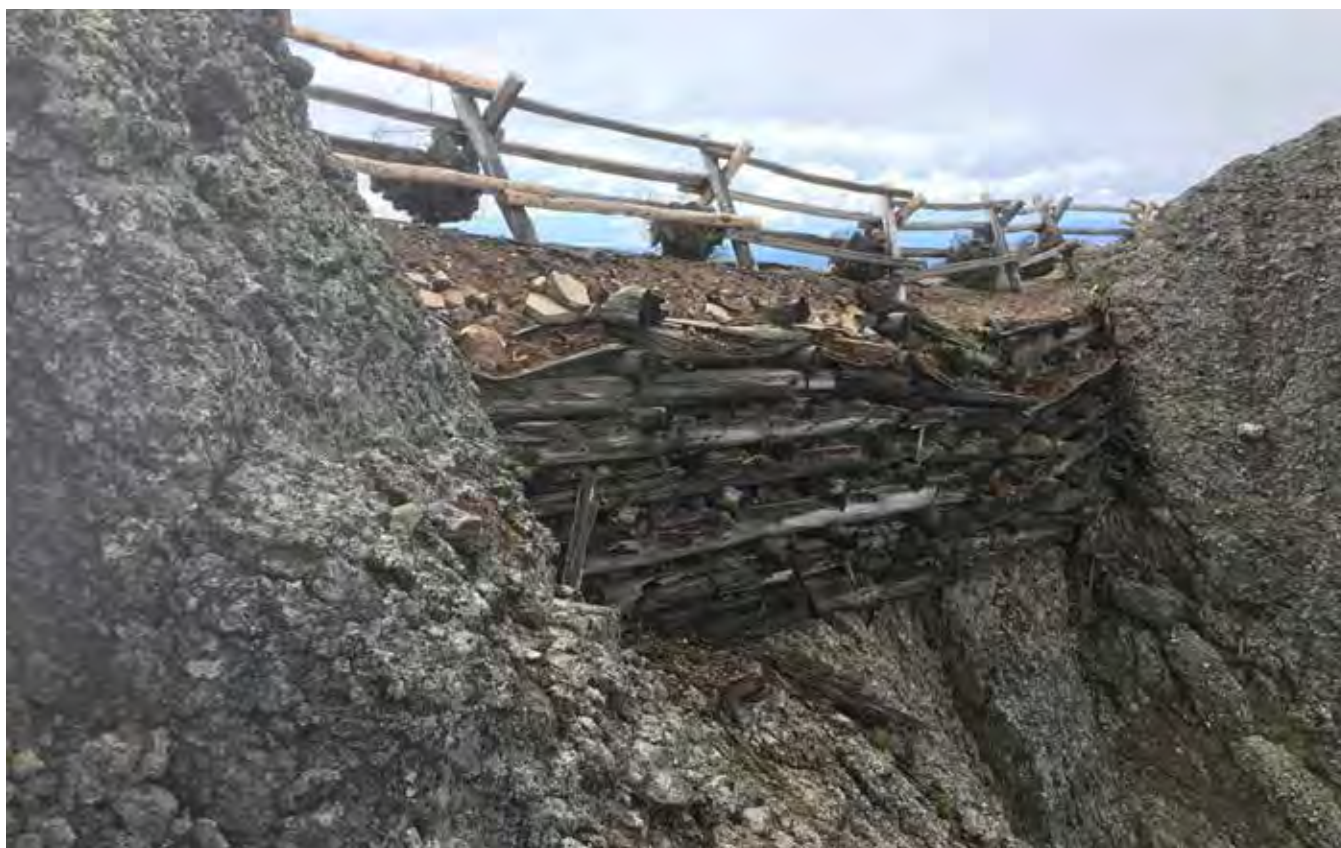
Log cribbing on the Old Chittenden Road near the top of Mount Washburn. This structure was built to bridge a ravine along the Old Chittenden Road between Tower Junction and Canyon Junction, which was completed in 1904 and used until 1931, when the current road alignment was completed.
