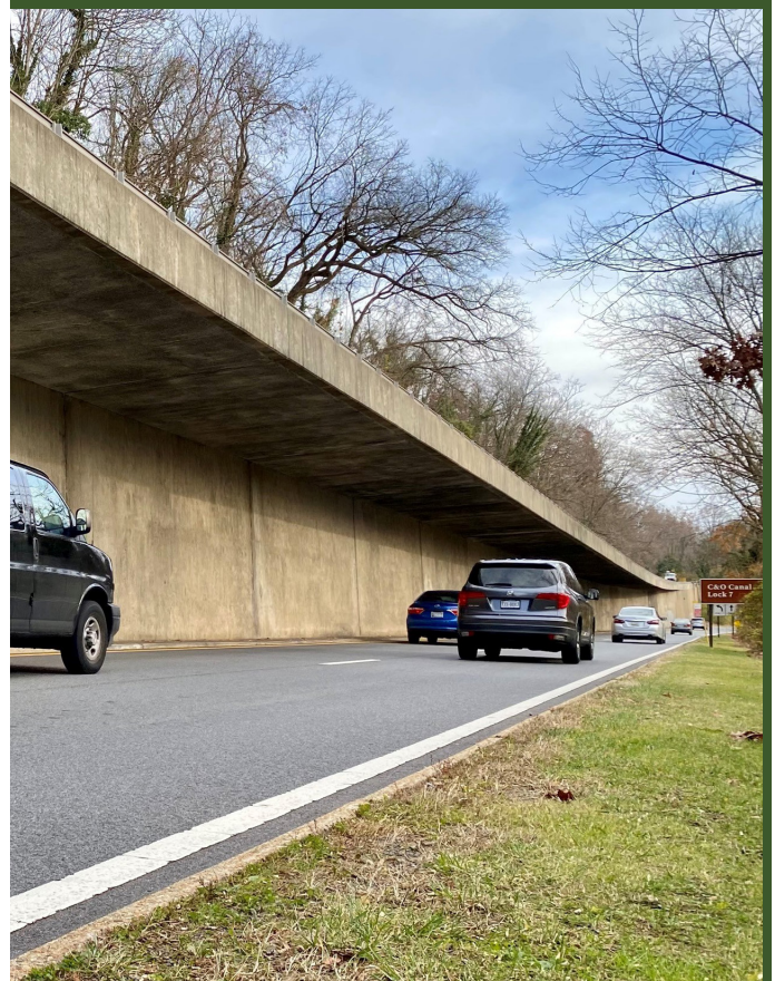
View of the Clara Barton Parkway travel lanes below the cantilever.
