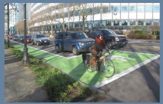
Figure 3-18: (left) Intersection crossing marking in Denver, Colorado. (Source: Ashley Haire, Toole Design Group); (right) Bicycle Box in Portland, Oregon. (Source: NACTO Urban Bikeway Design Guide)
