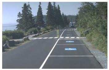
Figure 4-6: Improved visibility at a marked crossing location in a rural park setting. (Source: NPS)
