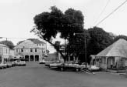
Illustration 12: A northwest view of Market Street shows hipped roof houses in the foreground and the background in Christiansted Historic District, St. Croix, Virgin Islands, circa 1976.
