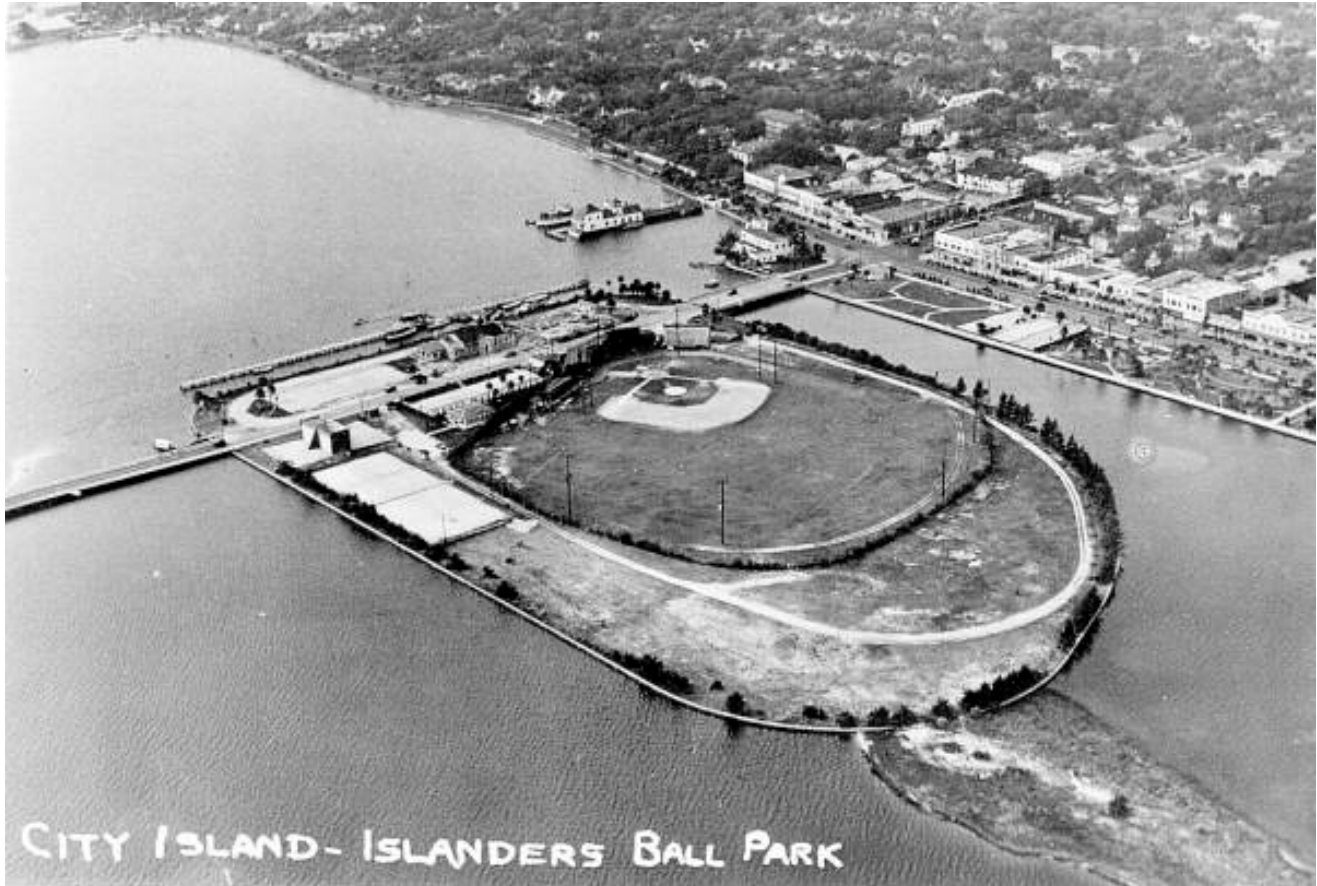
Photo 1: Aerial view of City Island Ballpark, circa 1930s.
