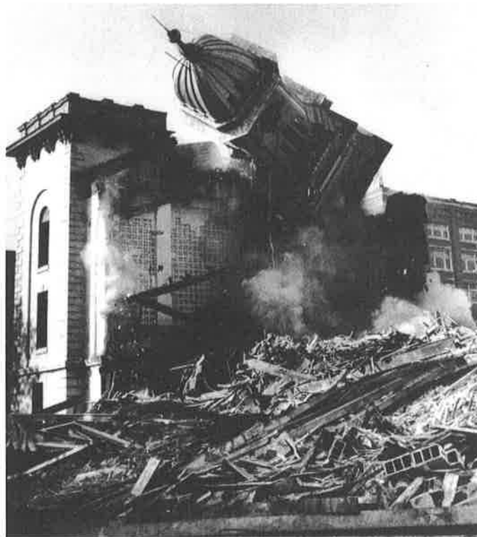
The 125-foot tower of the Lycoming County Courthouse in Williamsport, PA, falls during the 1969 demolition of the 109-year-old landmark. AP Wirephoto, RGW 51430rgw.
