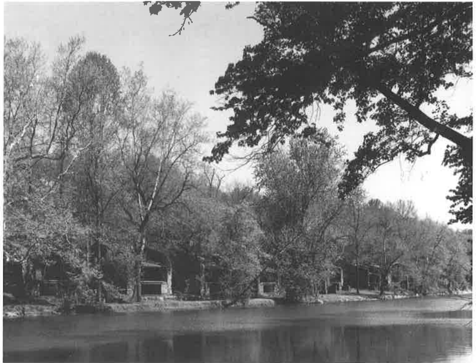
The shells of 17 of the original 21 roll mills survive along Brandywine Creek; buildings open to the water and tree density were safety features in case of explosions. Photo courtesy The Hagley Museum.
