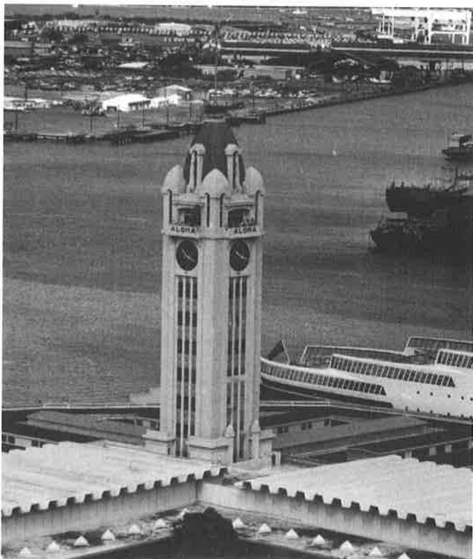
Once the tallest building in Honolulu, the 1925 Aloha Tower symbolizes the importance of both sea transportation and tourism in Hawaii's history. Photo by Gary T. Cummins
