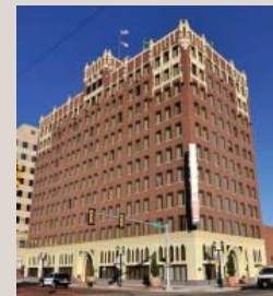
Fisk Medical Arts Building, Amarillo, TX (photo: Chirage Patel, Amarillo Hospitality LLC)
