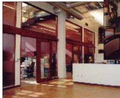
W. P. Fuller Paint Building, Salt Lake City, Utah-- interior and exterior views following rehabilitation.
