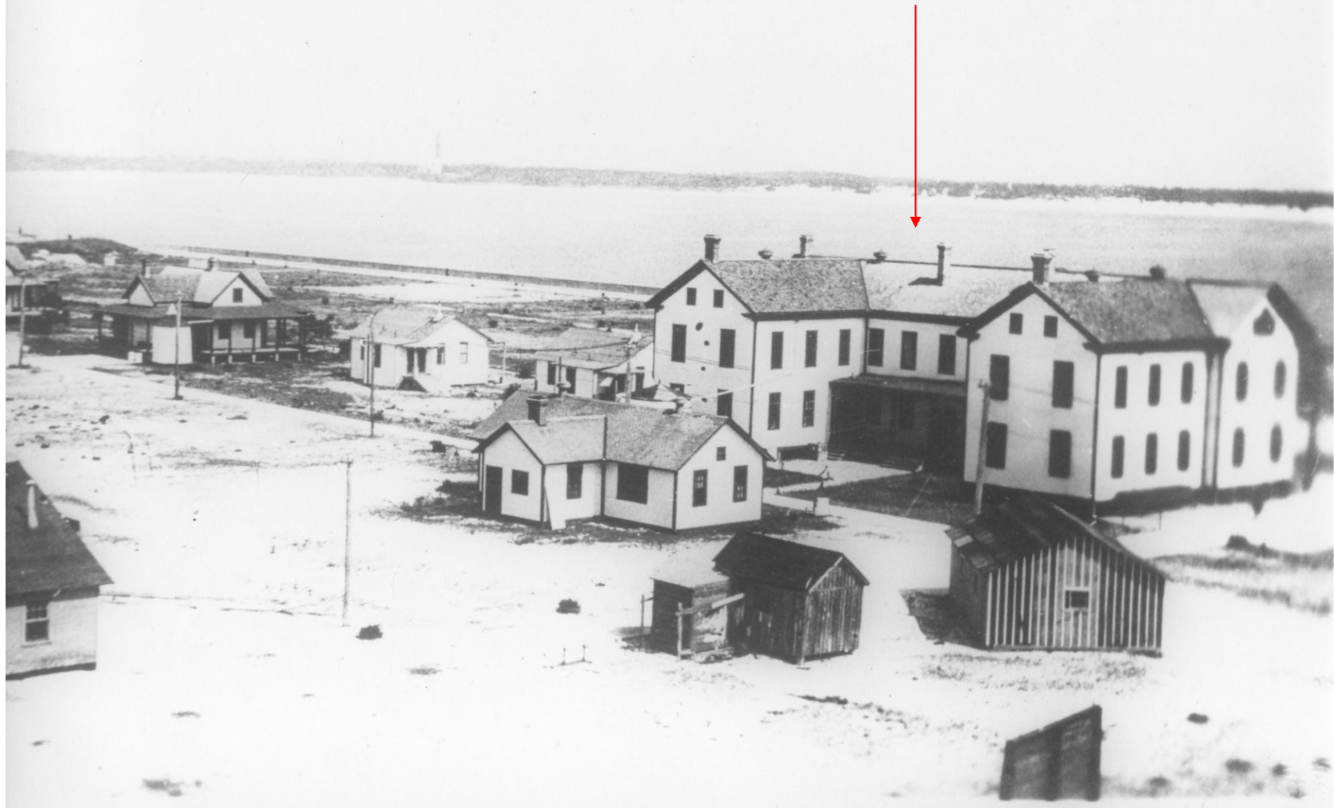
Enlisted Men's Barracks, 1900-1940
