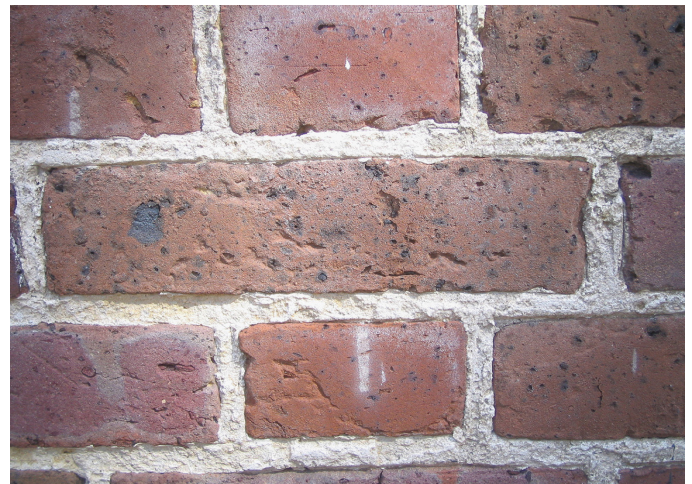
Detail of Handmade Bricks, Pompion Hill Chapel after Pointing
