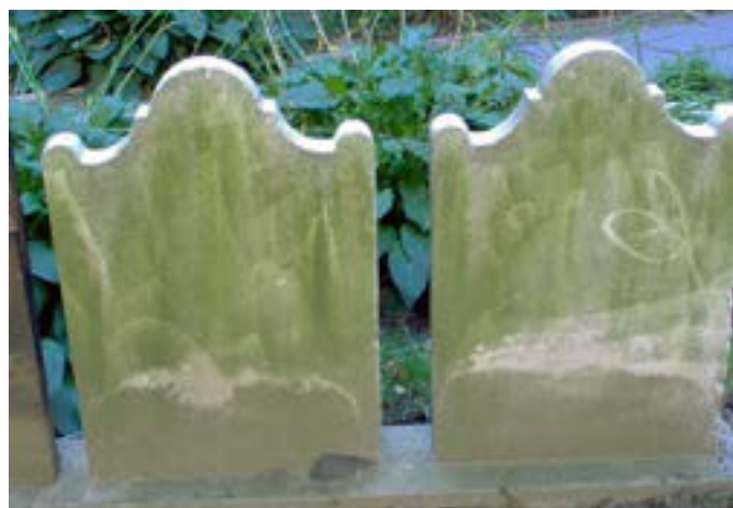
Figure 14. High-pressure water washing can damage grave markers. The photograph shows "wand marks" on the headstones produced by inappropriate pressure washing. Photo: Jason Church.
