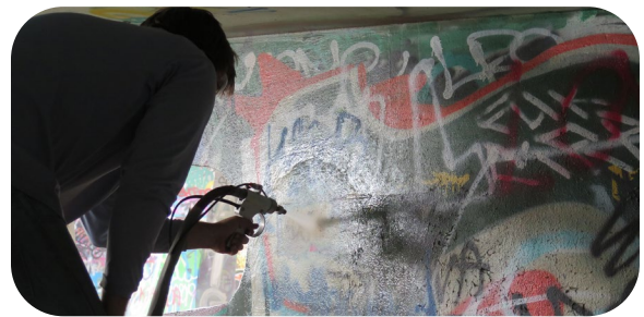
A preservationist tests the Ibix® Abrasive system to remove graffiti from a concrete surface. Photo courtesy of RLA Conservation, Inc.
