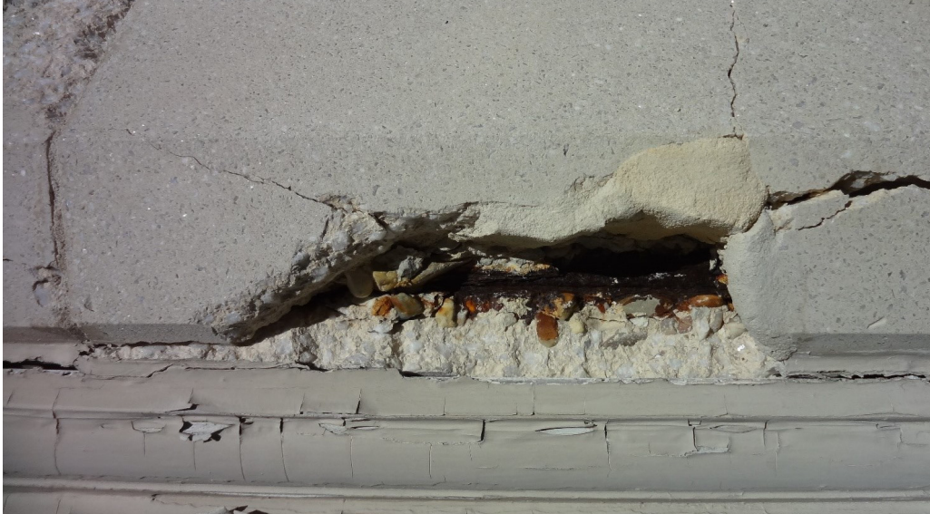
Examine stone frames for loose fragments and missing mortar. Source: Jason Church.
