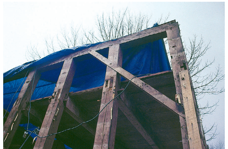
In Dutch houses, where wall posts are closely spaced, builders might use passing braces to achieve a long (and so more effective) brace length. In this Alford, Massachusetts, house, undergoing renovations, the brace passes one post where it is lapped its full thickness and secured with a pin. Below, in lieu of normal braces, some German carpenters would angle a stud to serve as both brace and stud, as in this structure in Ephrata, Pennsylvania.
