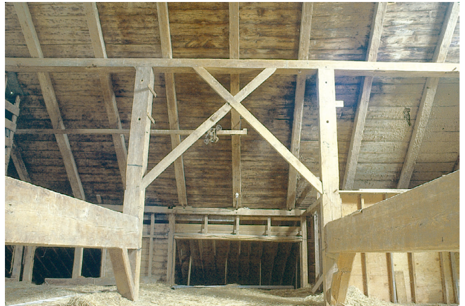
Dutch barns often had extremely long braces. In this upstate New York example, they are half-lapped where they cross.
