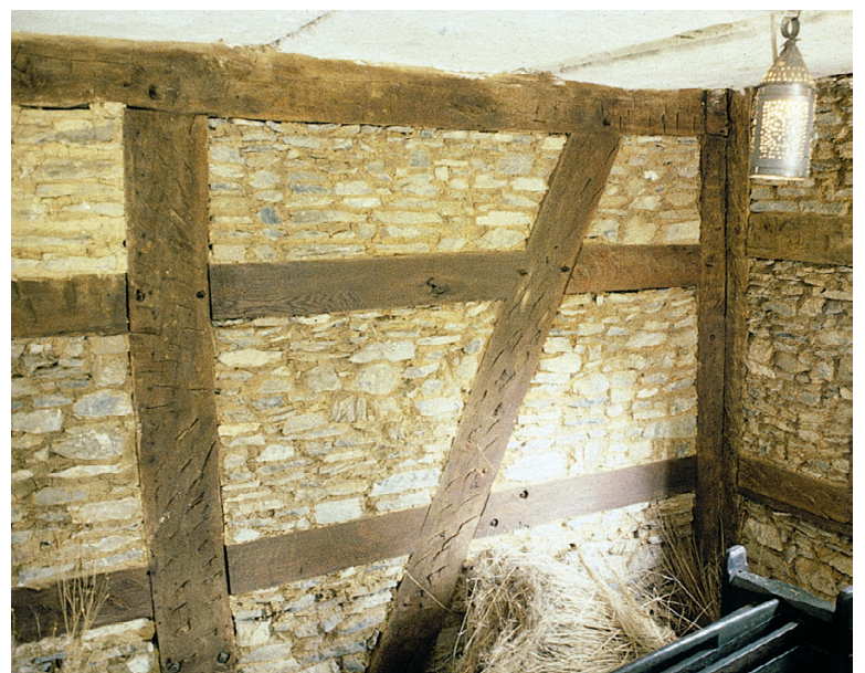
In Dutch houses, where wall posts are closely spaced, builders might use passing braces to achieve a long (and so more effective) brace length. In this Alford, Massachusetts, house, undergoing renovations, the brace passes one post where it is lapped its full thickness and secured with a pin. Below, in lieu of normal braces, some German carpenters would angle a stud to serve as both brace and stud, as in this structure in Ephrata, Pennsylvania.
