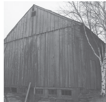
Boarding lapped at tie beam.
