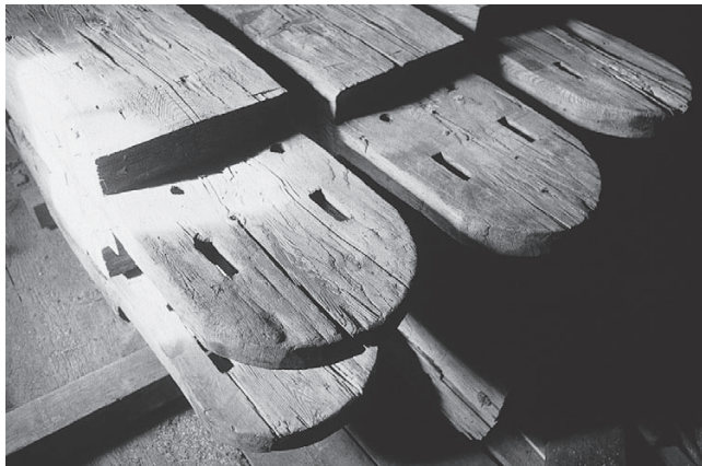
Anchorbeam tenon ends from a pre-1820 Dutch barn taken down in Altamont, New York.
