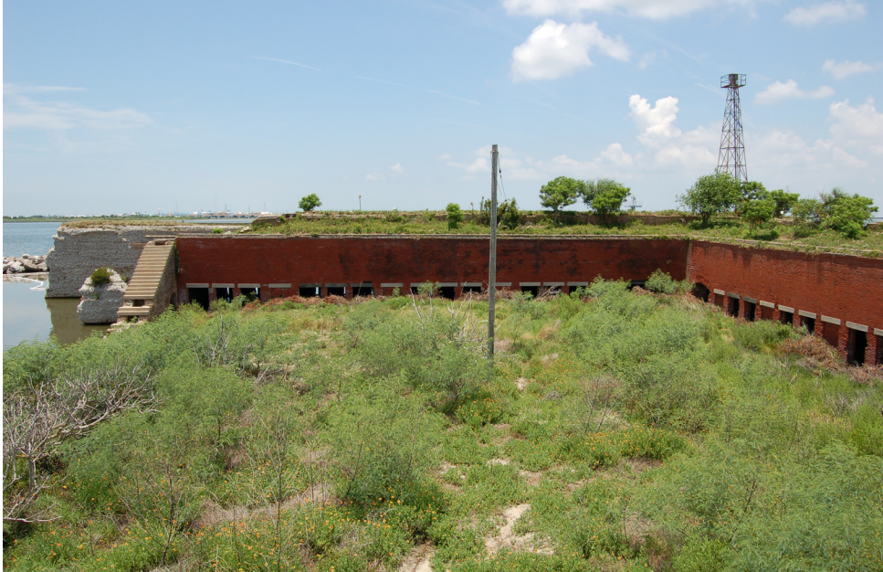
View across the courtyard looking southwest from the terreplein on the east side of the fort. Note the buildup of sand in the foreground, the light colored granite steps (left) and lintels over the openings in the brick walls, and the exposed tabby in the broken outer wall in the background, left of center. Barataria Pass and Grand Isle are visible beyond the fort. (Photo: NCPTT, Jason Church.)
