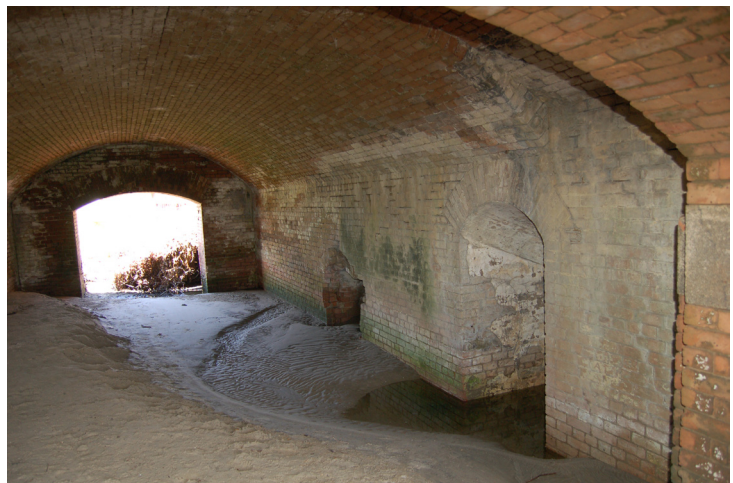
Barrel-vaulted passageway between the courtyard and the moat on the northwest side of the fort. Photo taken looking southeast toward the courtyard. Note the sand that has covered the floor and partially filled the space. Water has intruded as well, as seen on to the right in the photo, and evident from the flow channels in the sand. Oil has not contaminated this space. (Photo: NCPTT, Jason Church.)
