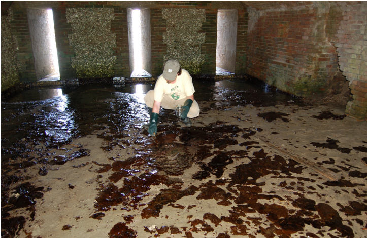
Location 2, inside the southernmost casemate. The cooler temperatures inside the casemate allow the oil to become more viscous so that it remains on top of the wet sand. Note the tabby walls with brick quoining in the background. (Photo: NCPTT, Carol Chin.)
