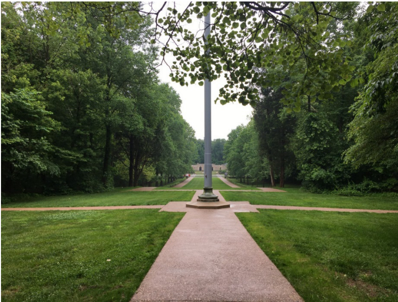
Figure 15. The new colored concrete-aggregate is poured and pretty surrounded by the lawn of the formal landscape of the Allee. (NPS/Rhonda Schier)
