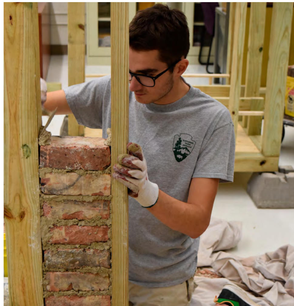
Gregory Lefebvre, Student FFB-CPB 4.0 Intern, adds brick masonry to the framed model houses in the laboratory.
