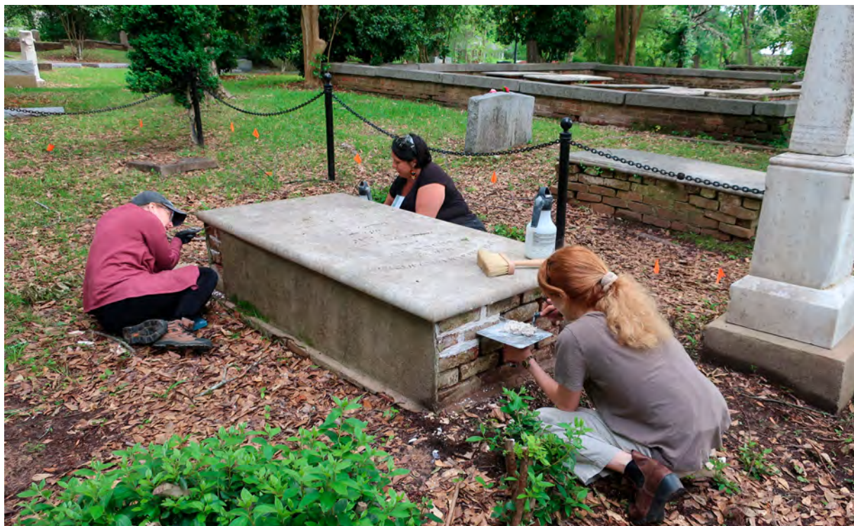
Mortar workshop participants repoint a brick box tomb using mortar mixed from lime putty.
