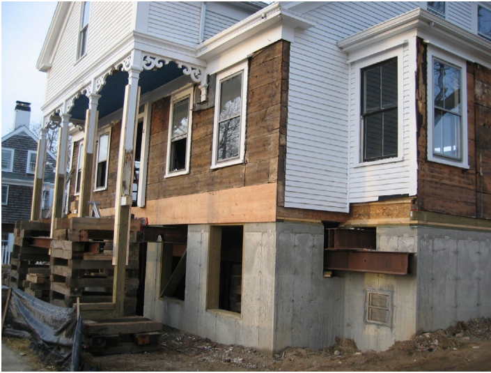
A home is elevated on extended poured concrete foundation walls.
