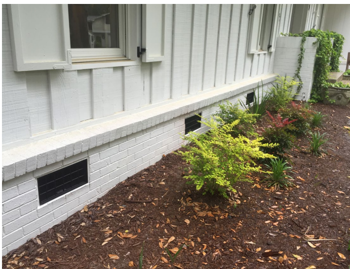
Flood vents allow water to enter the basement, preventing excessive pressure from developing on the basement walls.
