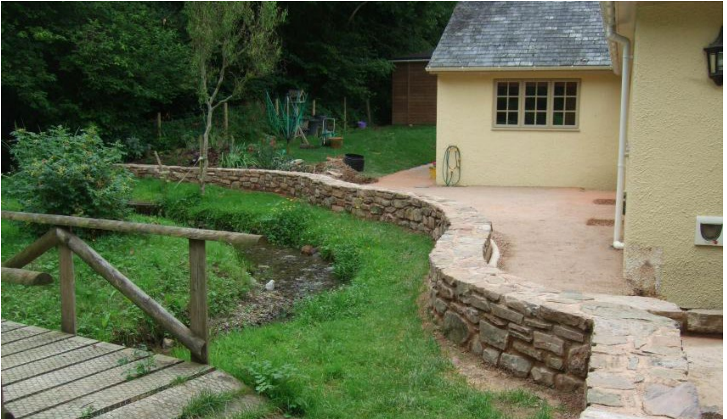
A small stone floodwall that protects the house from a local creek.
