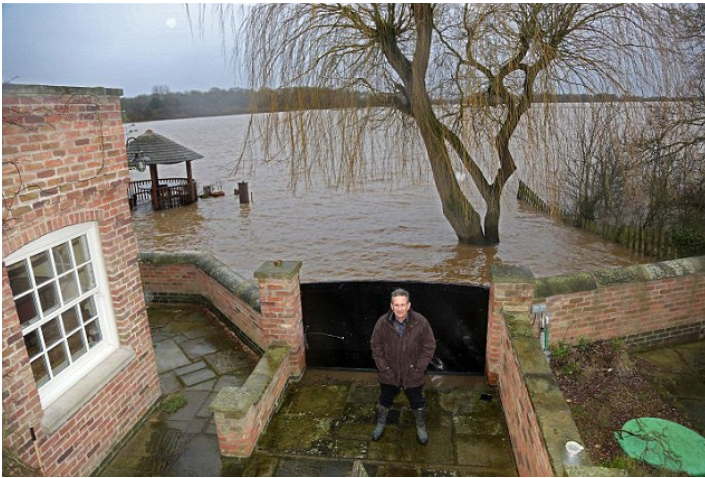
An example of a permanent brick floodwall designed and constructed by Carl Canty at his home in Bubwith, England, along the River Derwent.
