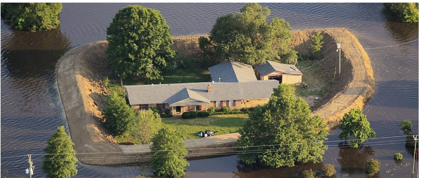
A levee constructed of soil and sand protects a single home in Vicksburg, Mississippi along the Yazoo River.
