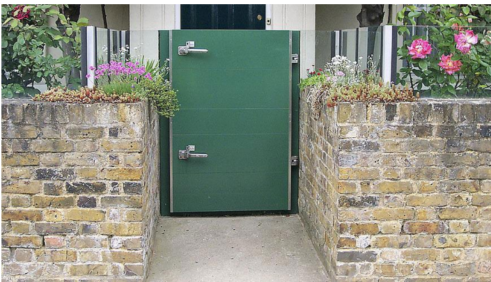
A swing-hinged flood gate provides access along this permanent brick floodwall.
