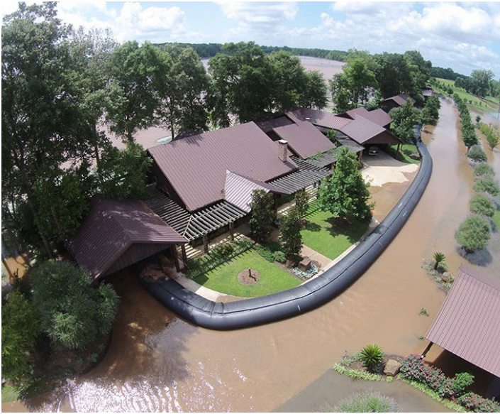
An example of a water-filled temporary barrier system by Aqua Dam.
