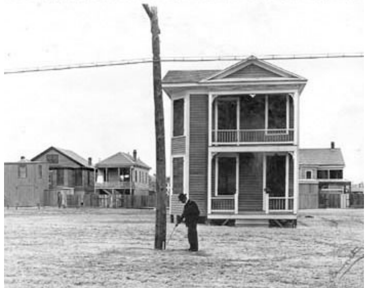
Almost the entire town of Galveston, Texas, was elevated after the 1900 Galveston Hurricane devastated the town and caused severe damage.
