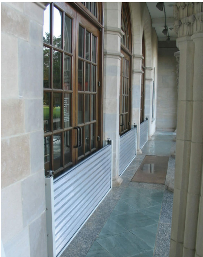
Flood shields in front of doors and windows should be placed before a flood event to prevent water from entering the building.
