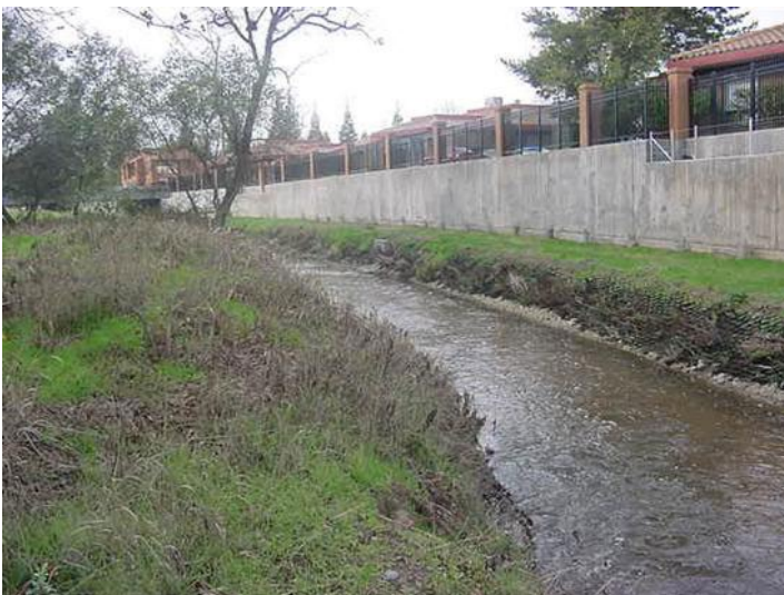
A concrete floodwall permanently protects the community of East Park in the City of Rosevill, California, from flooding along the Dry Creek.
