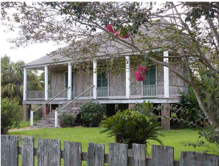
In Louisiana, there has been a long tradition of building houses on open brick pier foundations, as seen here at this French Louisiana Cottage from the early 1800s in Gramercy, Louisiana.
