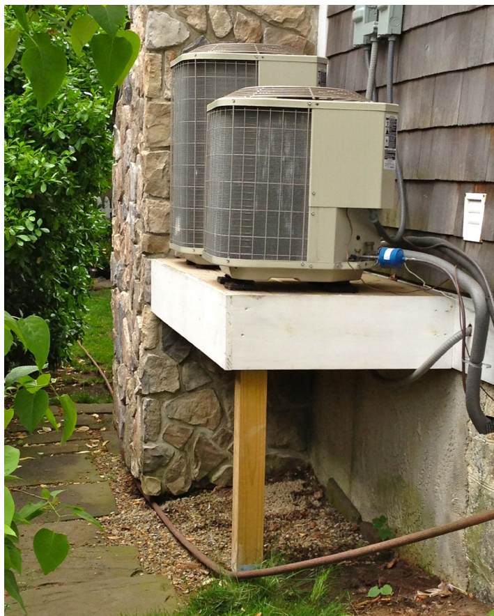
To protect outdoor utilities, such as air conditioning units, they should be elevated above the flood level.
