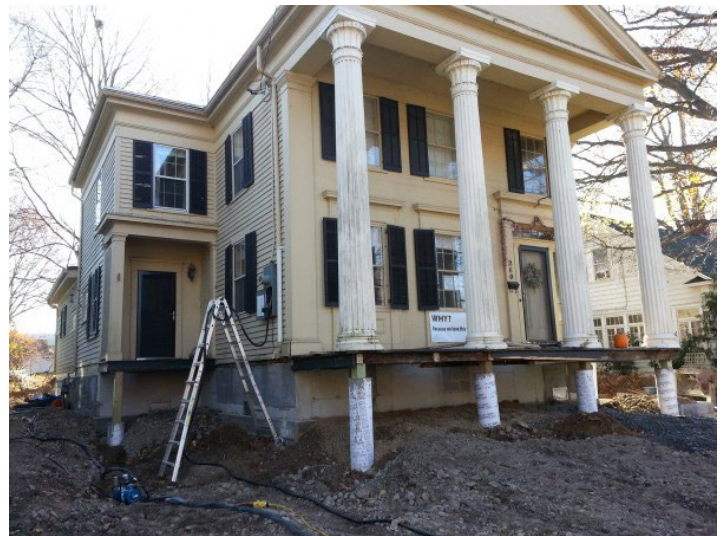
The same home after being elevated onto an extended poured concrete foundation.
