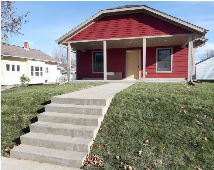
In La Crosse, fill was added on Charles Street to elevate new homes above the floodplain.
