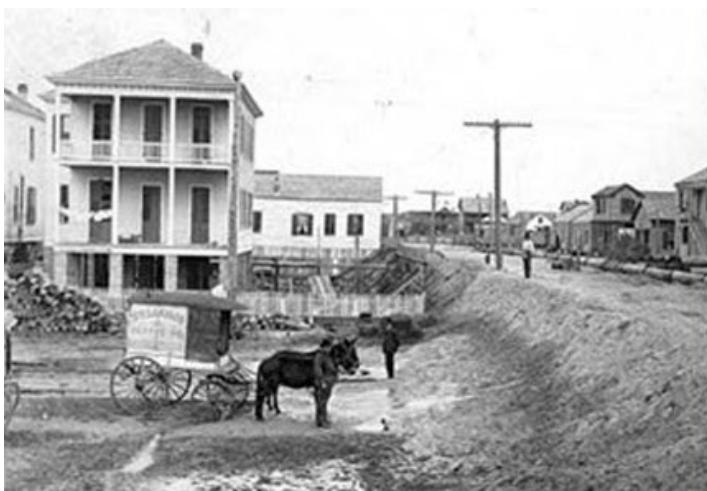
After the 1900 Galveston Hurricane hit Galveston, Texas, much of the town was elevated on new fill. In this image, part of the town has been covered in fill, while the rest of the town is only elevated by posts.
