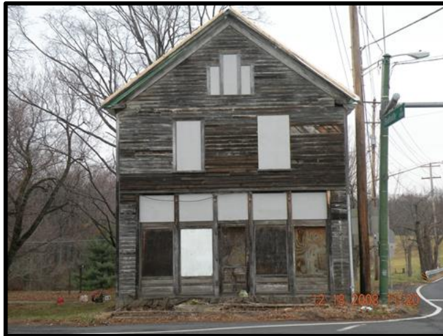
Figure 5.1 Weathered cladding from a naturally durable wood species that results in an appearance quite different than if it was painted.
