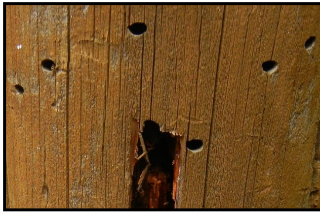
Figure 4.10. Bore holes in a stained column (also with deterioration by wood-decay fungi).
