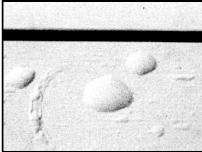
Figure 4.13. Moisture blisters in paint. Image from Cassens and Feist 1988.
