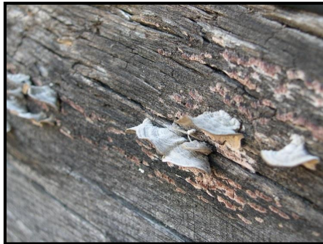
Figure 4.9. Fungal fruiting bodies growing out of a wood substrate.
