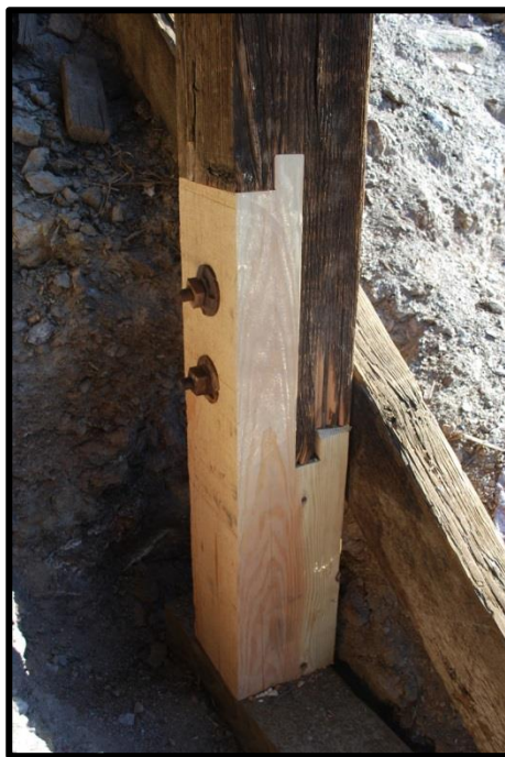
Figure 5.6. A Dutchman repair on an exterior column that had deteriorated in ground contact (courtesy of Douglas Porter, Conservation Associates).
