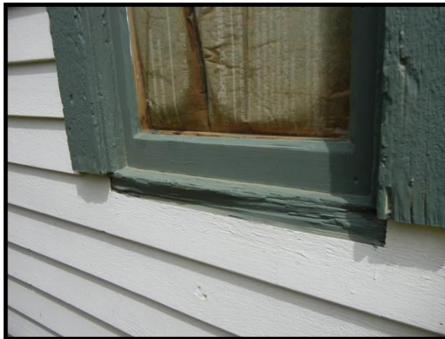
Figure 4.17. Missing window sill.
