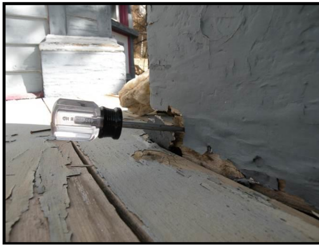
Figure 4.18. Probing at the base of a porch column with an awl reveals some deterioration.
