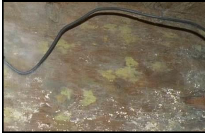
Figure 4.4. Yellow and white mold growth on an uncoated wood surface.
