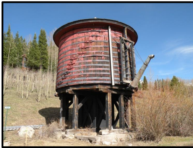
Figure 5.2. Deterioration of the staves of this water tank has resulted in friable wood surfaces that are delaminating. Given the fragile surface condition of many of the staves, repainting is not advised due to the potential damage that could result from removing the existing paint and properly preparing the surface for repainting; instead, replacement material can be painted to match the existing color, and the existing paint allowed to continue weathering.
