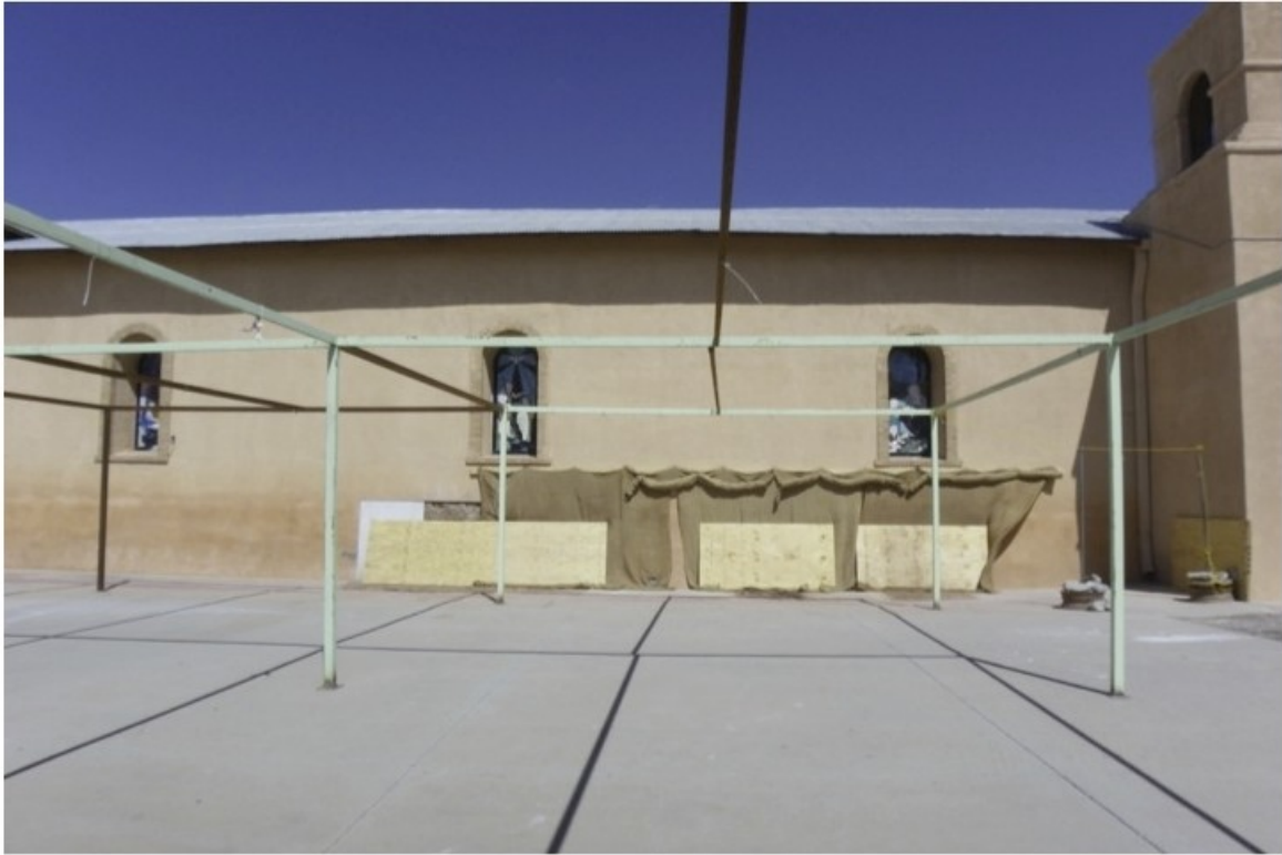
La Mesa Church work area
