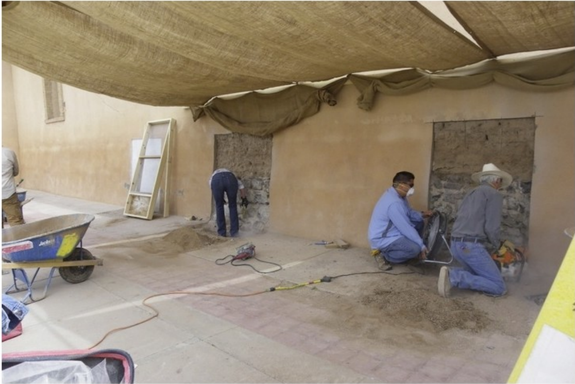
La Mesa Adobe Preservation Pilot Course – Wall preparatio
