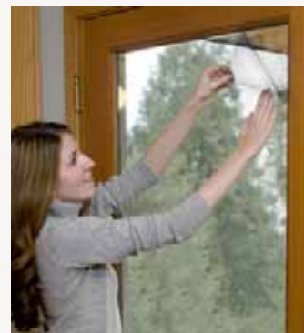
Homeowner installation of low-e interior surface film.
