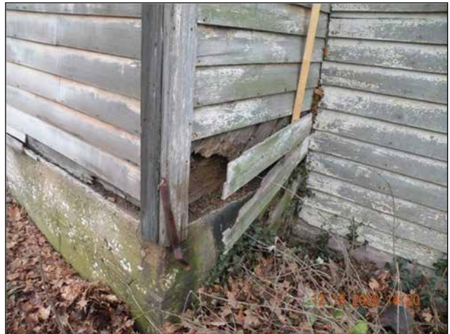
Figure 19—Deteriorated wall sheathing behind clapboard siding. Photograph courtesy of Anthony & Associates, Inc.
