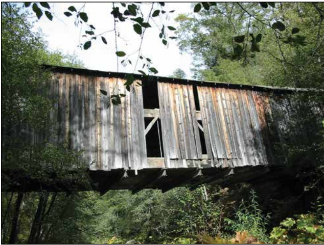
Figure 27—Vandals removed cladding from this covered bridge, exposing the large support beams to moisture.
