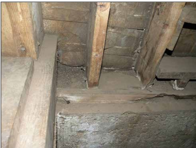
Figure 22—A sill plate resting on a concrete foundation below grade with evidence of deterioration. Photograph courtesy of Anthony & Associates, Inc.
