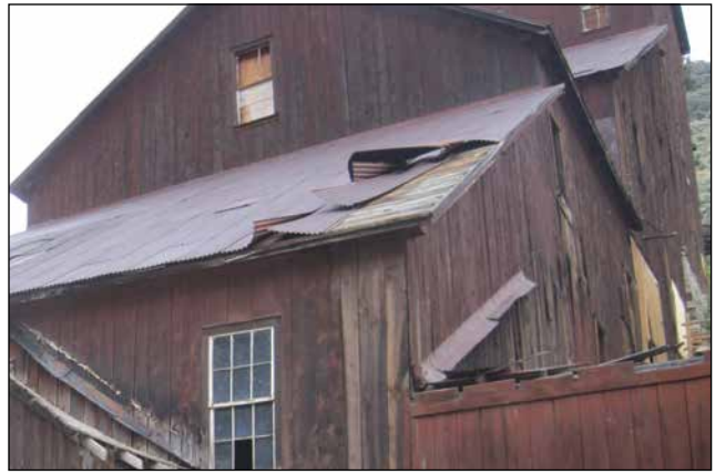
Figure 24—Repairing missing or damaged roofing material is a priority in preventing deterioration.
