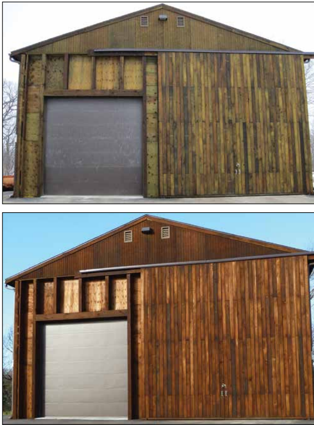
Figure 33—The green color of copper naphthenate tends to weather to brown over time. The photograph on the top is soon after construction and that on the bottom was taken one year later. This wood was pressure treated with oil-borne copper naphthenate.
