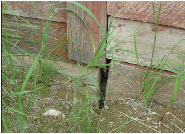
Figure 29—Over time, soil has accumulated against the wall of this house, virtually guaranteeing severe decay.
