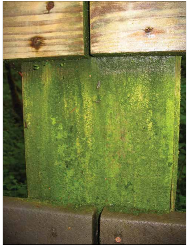
Figure 6—Green algae are commonly found on wood surfaces in moist, shady locations.
