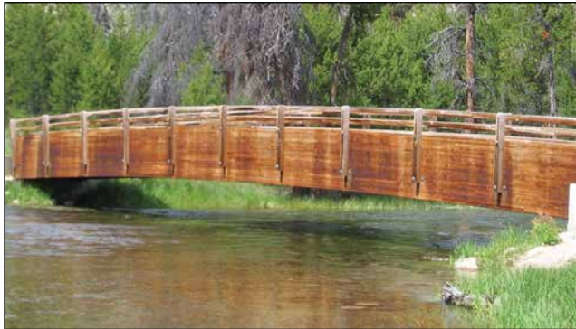
Figure B10—Glued-laminated beam treated with pentachlorophenol in heavy oil.
