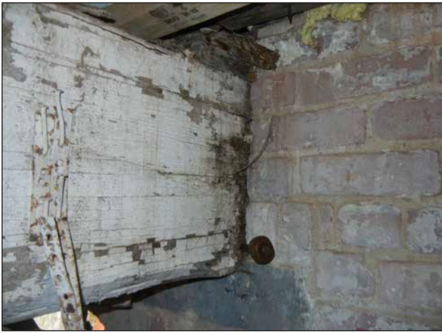
Figure 20—A structural beam with decay within the beam pocket. Photograph courtesy of Anthony & Associates, Inc.
