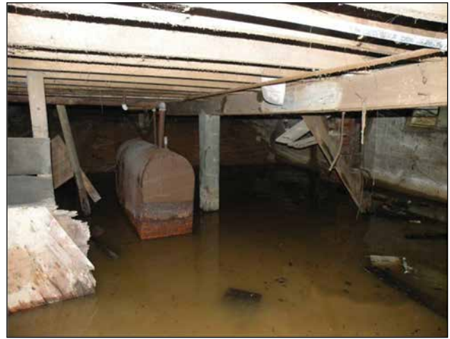
Figure 23—Wood girder and joists in a flooded crawl space; the evaporation of the water into the air and lack of air circulation greatly increases the likelihood of deterioration of these members. Photograph courtesy of Anthony & Associates, Inc.
