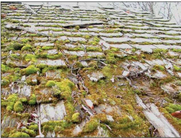
Figure 5—Moss on a cedar shake roof. Photograph courtesy of Anthony & Associates, Inc.
