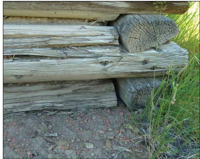
Figure 12—Ground contact greatly increases the risk of biodeterioration.
