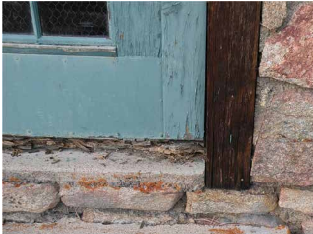
Figure 17—A severely deteriorated door threshold. Photograph courtesy of Anthony & Associates, Inc.
