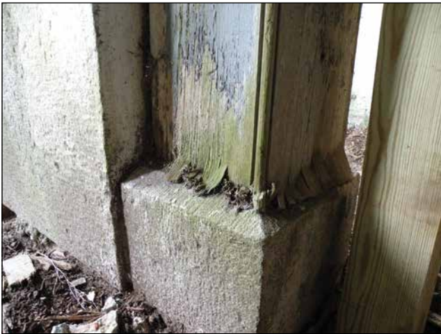
Figure 21—High moisture content and decay led to the crushing failure of this large timber column under design loads. Photograph courtesy of Anthony & Associates, Inc.
