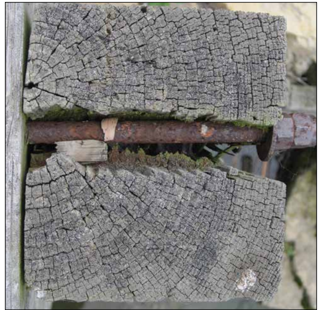
Figure 46—Metal fasteners are sometimes associated with decay pockets if holes are drilled after treatment and expose untreated wood.
