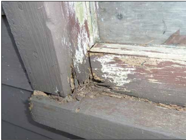
Figure 16—Windows and other millwork that can trap moisture can be vulnerable to decay.
