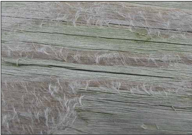
Figure 1—Weathering has caused cracking and loosened the fibers on the upper surface of this deck board.
