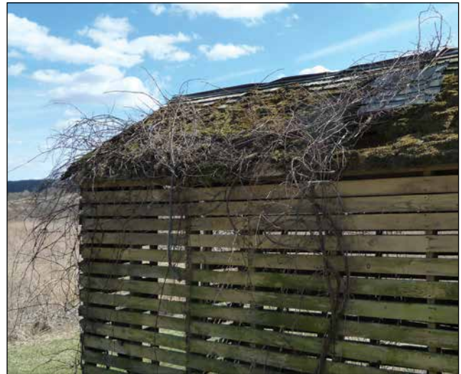
Figure 28—In addition to possible mechanical damage, vines create shading and trap moisture.
