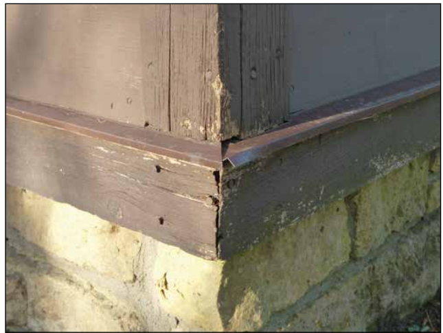
Figure 25—Improperly installed or damaged flashing can direct water into the structure and promote decay.
