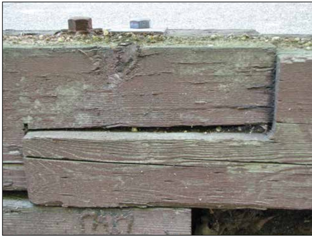
Figure 45—Unless it was pressure treated after fabrication, this type of connection creates a favorable environment for decay. It exposes untreated wood and creates an area that traps and holds moisture.
