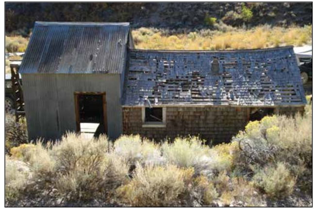
Figure 14—The lack of shingles allows moisture penetration into the roof and wall framing members of this mine building. Photograph courtesy of Anthony & Associates, Inc.
