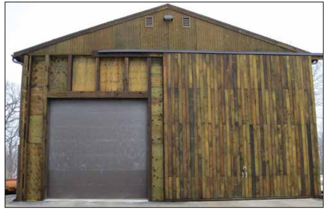
Figure B11—Salt storage shed treated with copper naphthenate in heavy oil.
