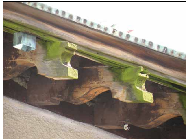
Figure 15—These rafter tails exhibit discoloration and green mold growth indicative of a high-moisture environment. Photograph courtesy of Anthony & Associates, Inc.
