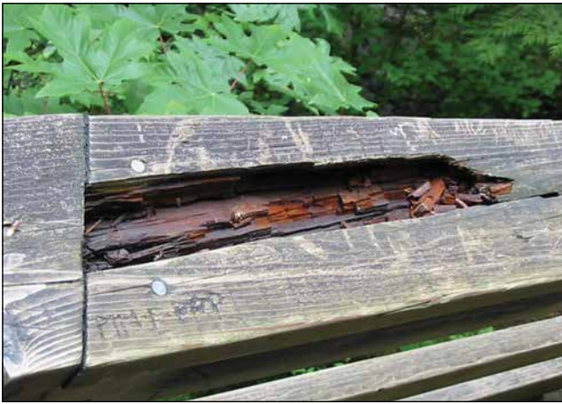
Figure 7—Typical brown-rot decay.
