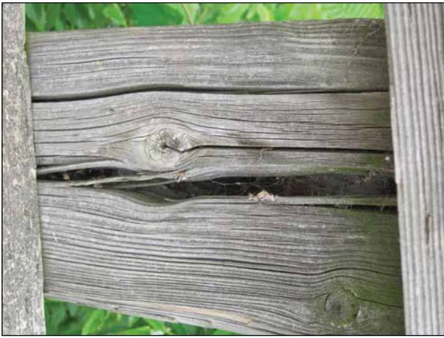
Figure 43—Deep seasoning checks can be an indication of potential problem areas unless the checks formed prior to pressure treatment.
