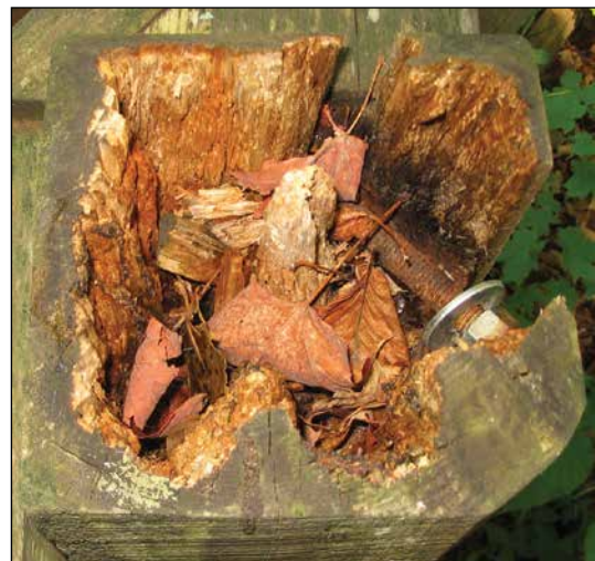
Figure 44—Examples of internal decay in vertical members that were cut to height after installation. Only the preservative-treated zone remains sound. In some sawn members with heartwood faces, the treated zone may not be complete (see photograph on bottom). Fortunately, most pressure-treated members have greater penetration than shown in these examples.
