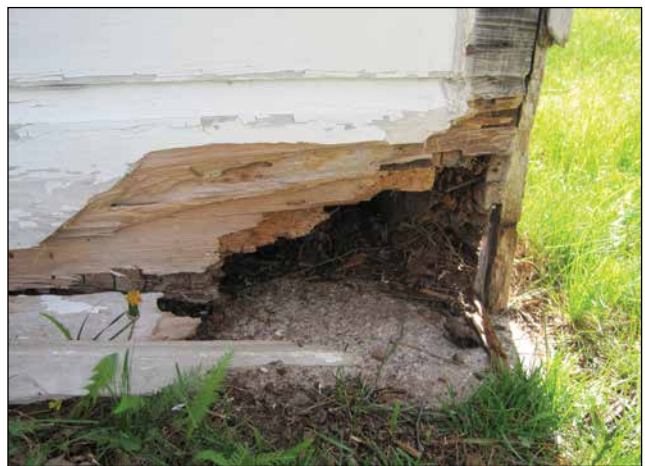
Figure 26—A leaking downspout led to decay in the corner of this historic cabin.
