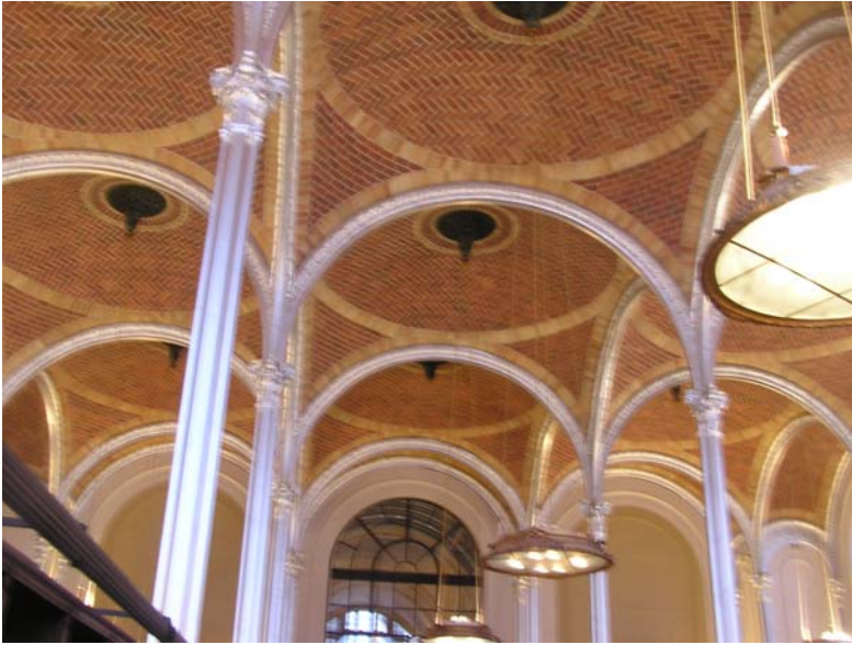
Figure 56: The view of rib and dome construction.
