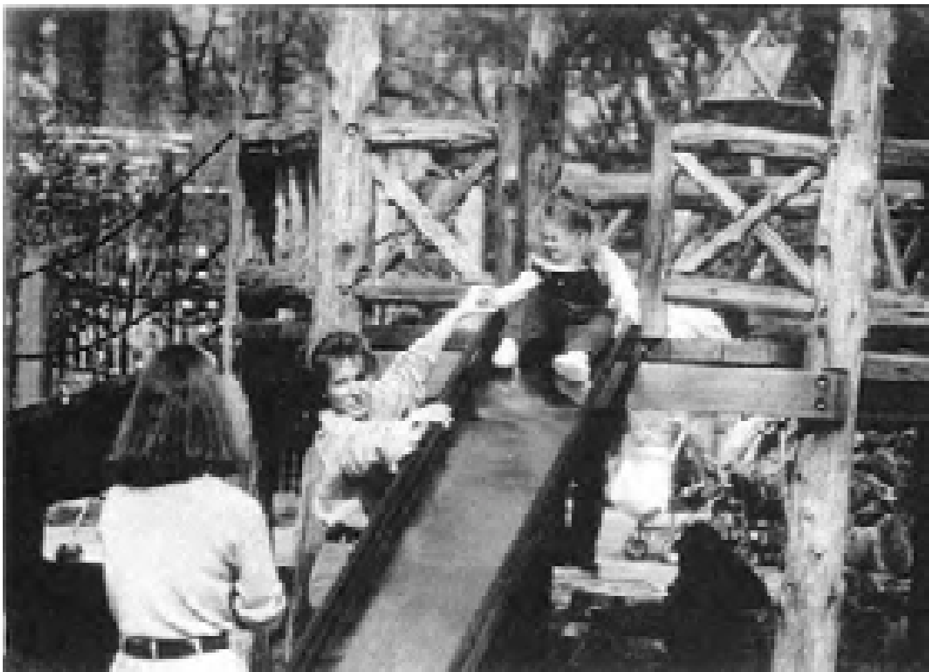
This Central Park playground had become deteriorated over time. Rather than replace the structures with standard apparatus from a catalog, the new play structures—made of traditional materials—are compatible with the park's historic character. (Central Park Conservancy)
