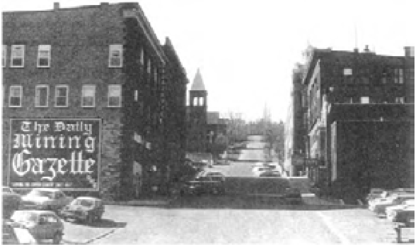
Many of the mining communities that prospered during the late 19th and early 20th centuries often possess a rich legacy of historic architecture, as demonstrated in this 1983 view of downtown Houghton in the “Copper Country” of Michigan’s Keweenaw Peninsula. Photograph by Richard Francaviglia.
