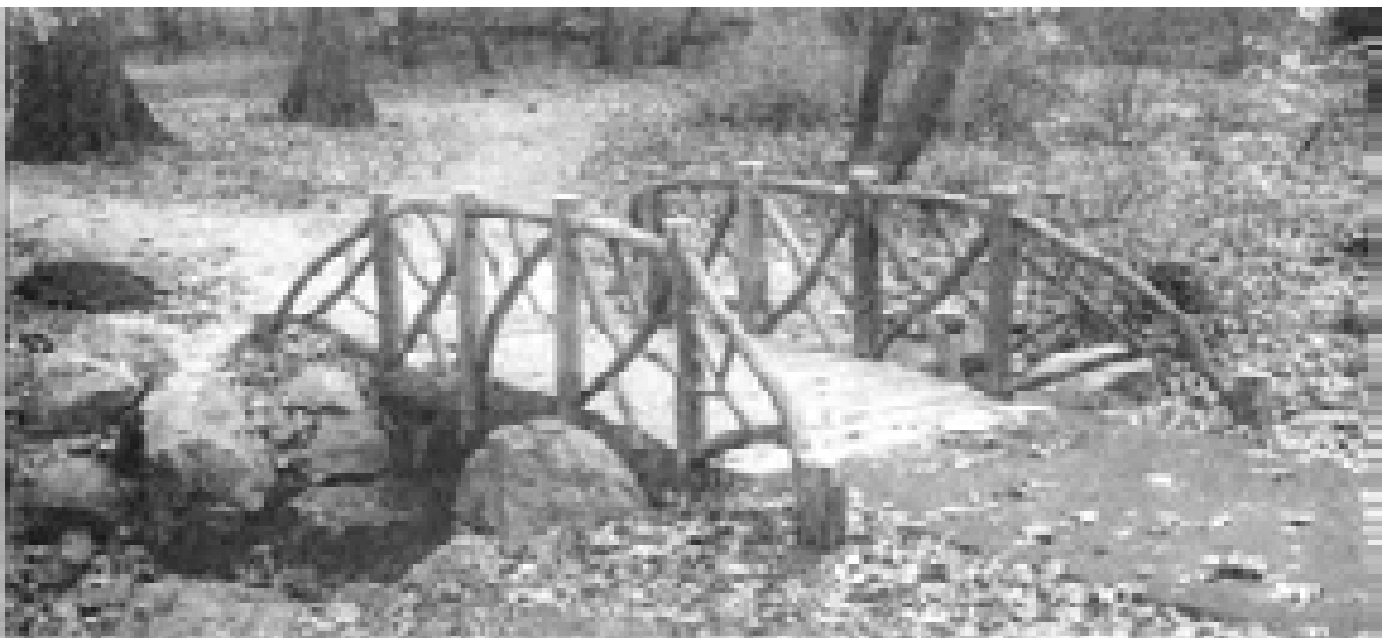
This small footbridge in Central Park's Ramble [above] has been re-created on the basis of historic documentation. The new bridge meets current code requirements, yet replicates the historic appearance, while utilizing compatible substitute materials. (Central Park Conservancy) The selected treatment for the landscape at the J. L. Bush Storehouse Property, Greenwich, Connecticut, [top] is restoration to the impressionist painters' period. Here, sensitive grading preserved historic landscape features while providing access on the alignment of the original path. For example, grade relationships to the historic building and hedge have been retained. (LANDSCAPES)
