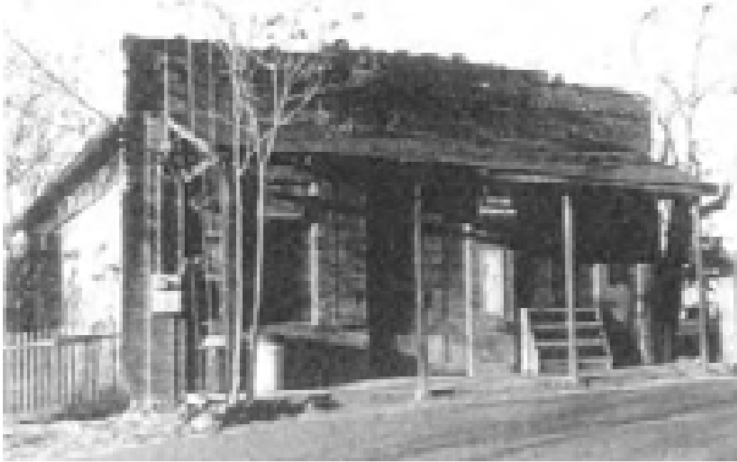
Mining communities such as Chinese Camp, California, often make good use of older buildings. This historic store, dating from about 1860, serves as a visitors' information center and makes a tangible connection with the past. Photograph by Richard Francaviglia.
