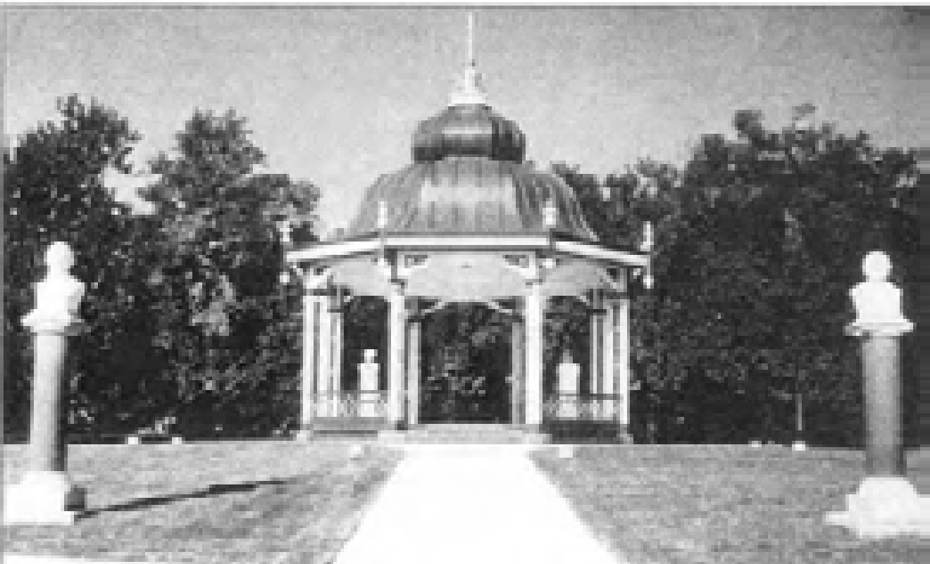
The area known as the music pavilion at Tower Grove Park in St. Louis, Missouri, had been badly deteriorated including its central marble busts, radiating walks, lawn areas and curbing. Utilizing photographic documentation, [top] the pavilion [opposite top right] and its associated landscape were restored to portray the pavilion as it would have appeared at a certain time. For example, the marble busts of eminent composers were replaced with pre-cast concrete replicas of the originals [bottom, foreground]. (Tower Grove Park)
