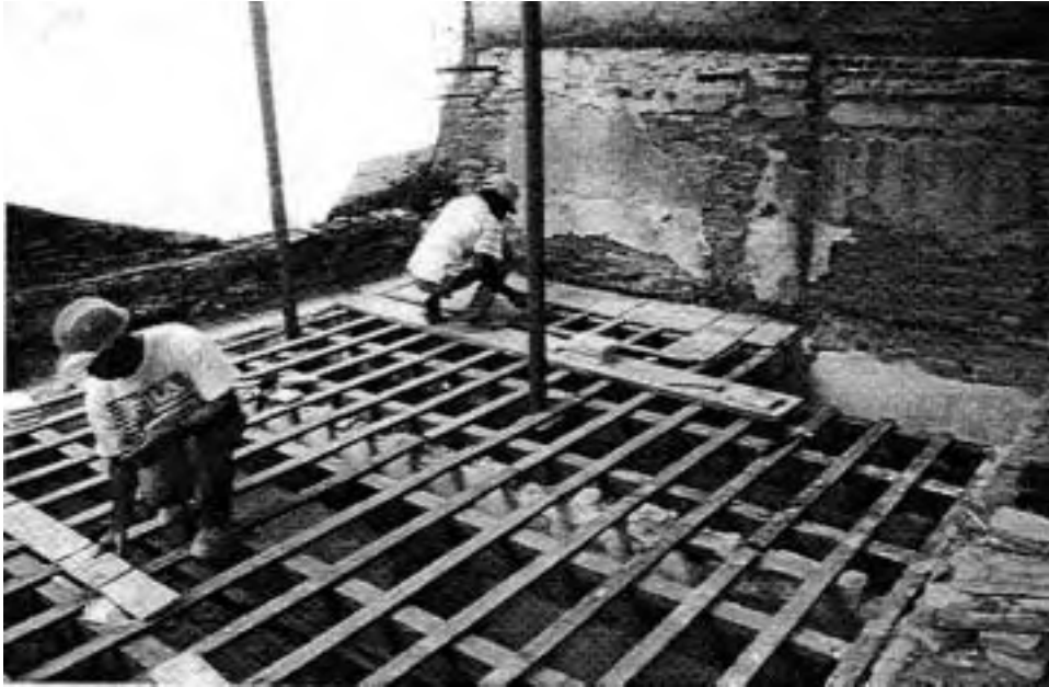
The reconstruction of the flat ceiling and roof utilizing recycled historic ausubo (bullet wood) roof beams, slats and brick in the Casa Ramón Power y Girth Restoration Project Old San Juan, PR (1994).
