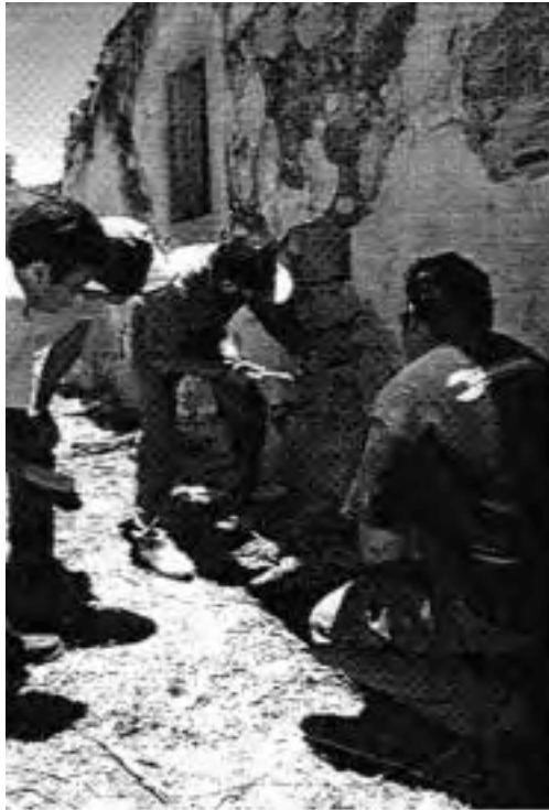
Repointing and replastering exercise, on the Casa de Caminero at Juana Diaz, being directed by Conservation Architect John Fiddler (left). Architectural Conservator Jeanne Marie Teutonico explains issue of “material compatibility”(right). Design 203 Architectural students during fieldwork exercises from the Polytechnic University of Puerto Rico (1997).
