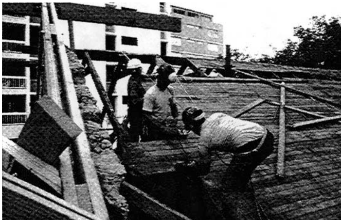
Cutting wood boards before dismantling original roof truss during Colegio de Arquitectos Headquarters restoration in Santurce, PR (19931).
