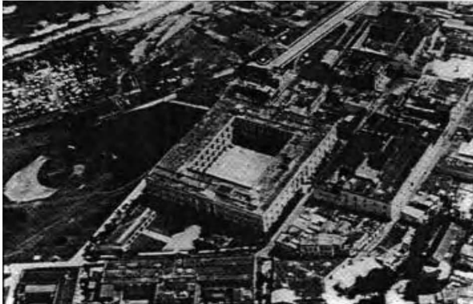
Aerial view of El Morro grounds in Old San Juan, PR. with Ballajá Military Barracks in the center of the photo (U.S. Corps of Engineers. 1924).
