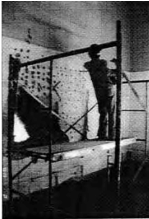
Drilling reinforced concrete wall before removal from adjacent historic fabric in Ballajá Military Barracks in Old San Juan, PR (1988).
