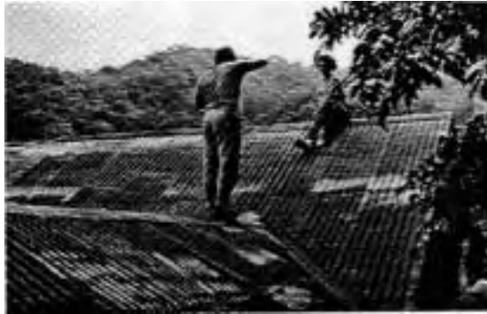
Main House roof documentation at Hacienda Buena Vista in Ponce, PR (1986).
