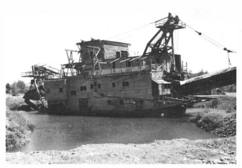
Placer gold mines were once numerous in the West. Some employed floating dredges, such as the Sumpter Valley Gold Dredge in Baker County, Oregon, to dredge up gravel and wash gold dust and nuggets from the waste. Dredges typically deposited large tailings piles along stream beds. (Oregon State Historic Preservation Office)
