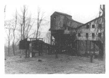
A coal tipple consists of the tracks, trestles, and screens where coal is processed and loaded. Coal tipples are good examples of Mine Development and Exploitation property types. Pictured is the Kay Moor tipple located along the New River in Kay Moor, West Virginia. (National Park Service)
