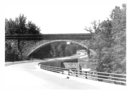
Cabin John Aqueduct, Montgomery County, Maryland. This stone arch was built in 1869 and was the world's longest until 1903. It was designed by Montgomery Meigs, U.S. Army Corps of Engineers. The aqueduct provided the principal source of water to Washington, D.C. throughout the late 19th century. (Michael Bourne, 1969)
