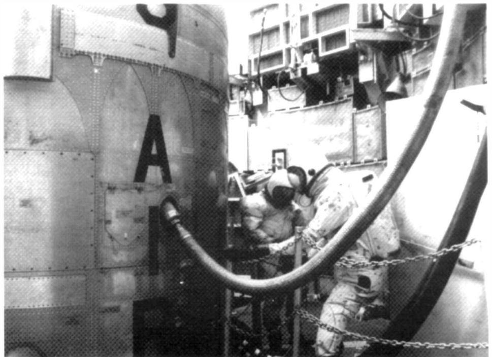
*The Titan II ICBM Missile Site 8 (571- 7) in Pima County, Arizona, was listed in the National Register in 1992. This view shows a simulated vapor detection check by propellant transfer technicians. (David K. Stumpf, 1992)*
