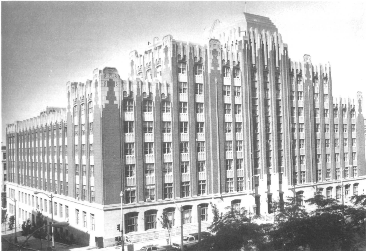
Federal Office Building, Seattle, Washington, 1932-33. In addition to being the city's first building designed especially for Federal offices, this was one of the first Modernistic-styled buildings designed by the Office of the Supervising Architect of the Treasury Department. The innovative use of cast aluminum spandrel panels beneath the windows was the first extensive use of aluminum on the West Coast. Much of the interior Art Deco ornamentation remains intact. (John Krapil)
