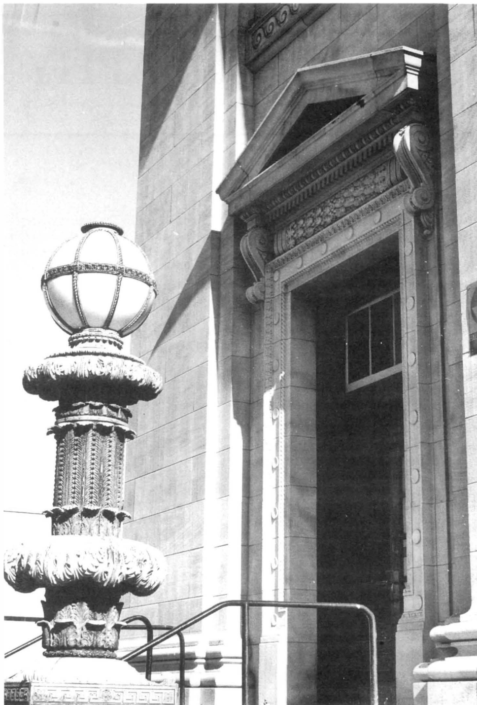
United States Post Office, Des Moines, Iowa, ca. 1908-12. The architectural significance of a building is often illustrated through a collection of rich detailing. This doorway and acanthus leaf lantern are part of a post office that is one of the best examples of classical architecture in central Iowa. (John H. Wetherell)
