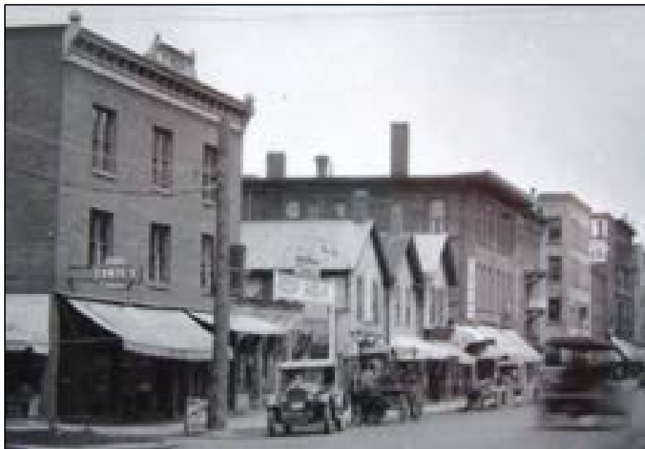
Figure 10. A c. 1915 view of South Main, looking northwest with three first-generation style, gable-fronted, frame commercial buildings, built c. 1865 (now expanded as HD #s 50-53) second from left.
