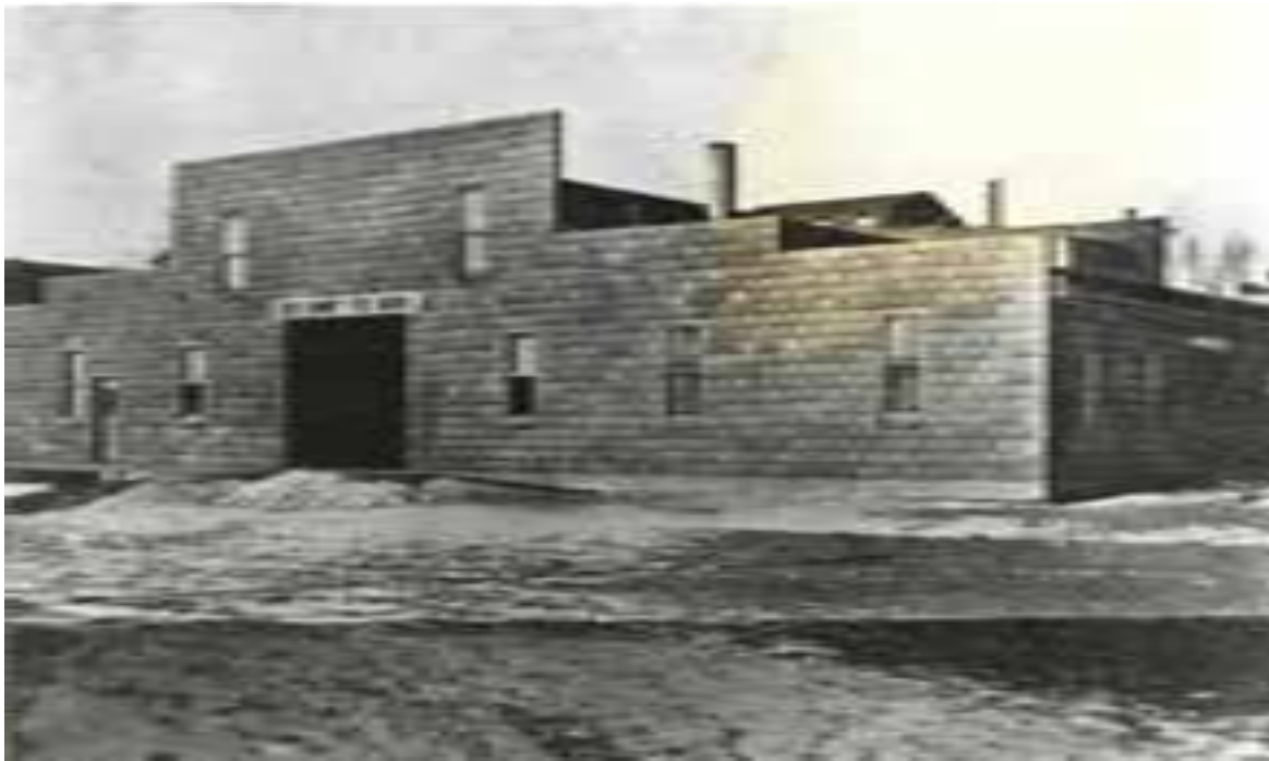
Bailey Tie Barn provided the raw materials for the Inavale Gymnasium. Photo Courtesy, Webster County Historical Society. Reverse of photo notes the building was torn down and materials used for Inavale Gymnasium.
