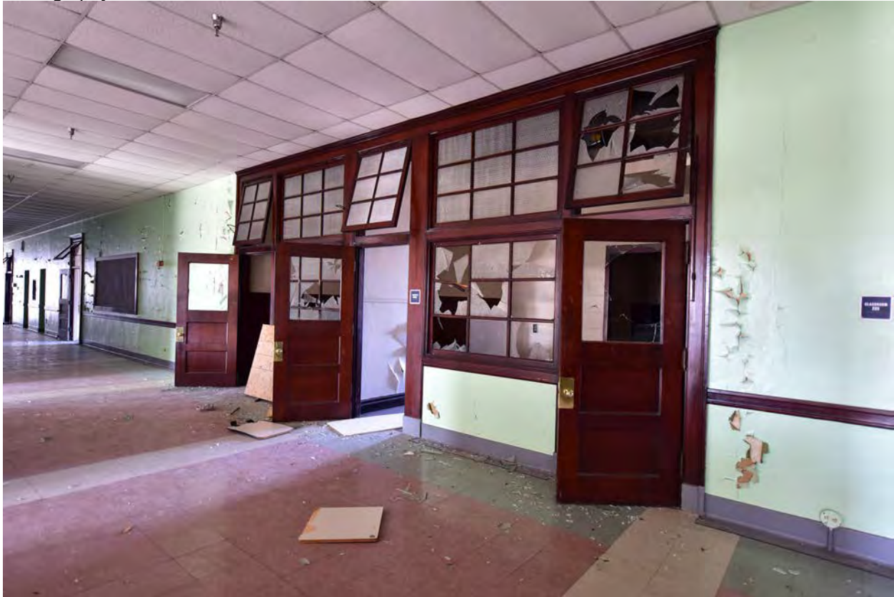
Figure 20. Photo of historic window wall on north side of second-floor corridor. Source: f-stop Photography, December 2020.
