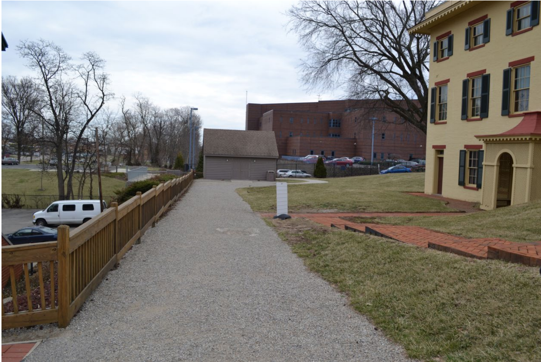
WILLIAM HOWARD TAFT HOME, Cincinnati, Ohio View east along Carriageway. Noncontributing carriage shed is at end of carriageway Photo by Liz Sargent, March 2014
