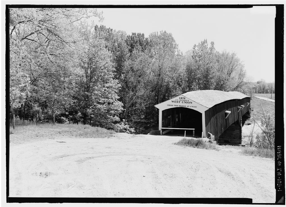
WEST UNION BRIDGE. General view from northwest. Photograph by James Rosenthal, 2004 [HAER No. IN-105-1].
