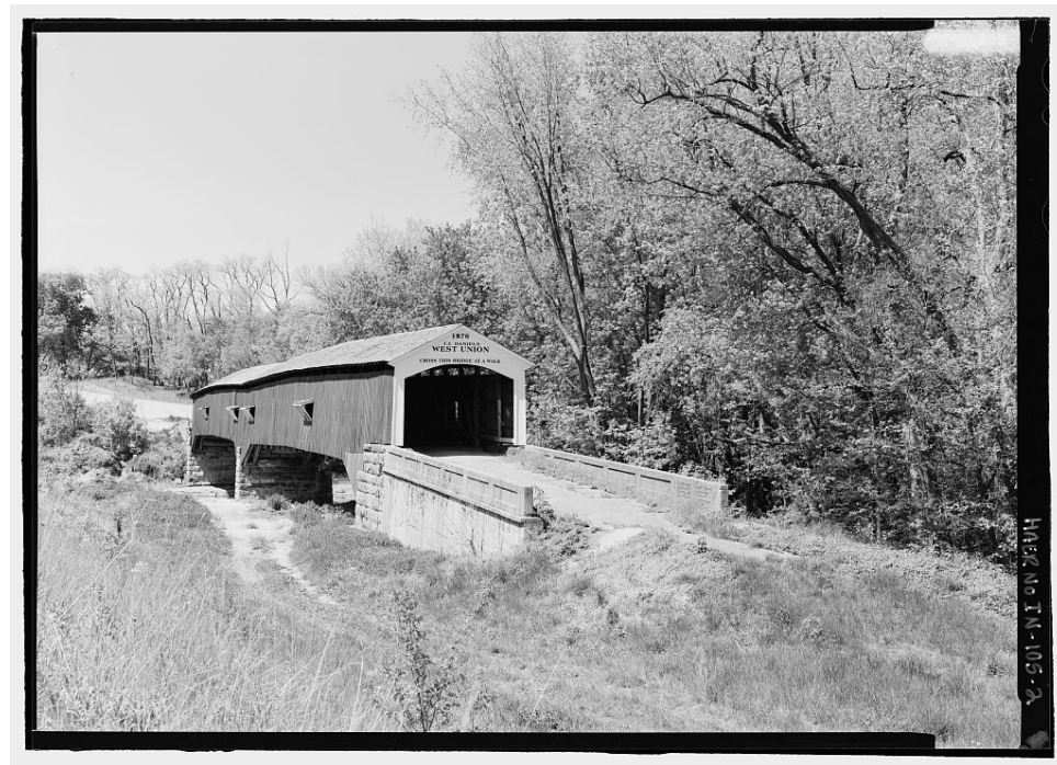
WEST UNION BRIDGE. General view from south. Photograph by James Rosenthal, 2004 [HAER No. IN-105-2].
