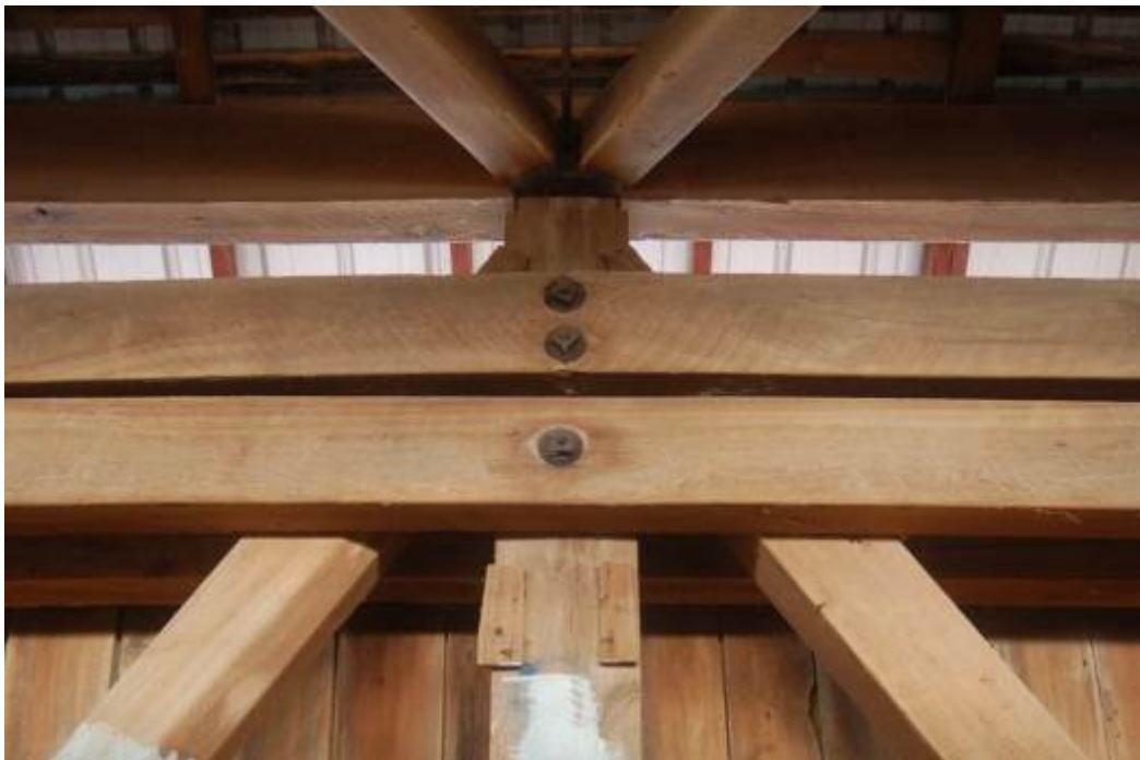
WEST UNION BRIDGE. Detail of arch-truss connection. Photograph by Lola Bennett, 2015.
