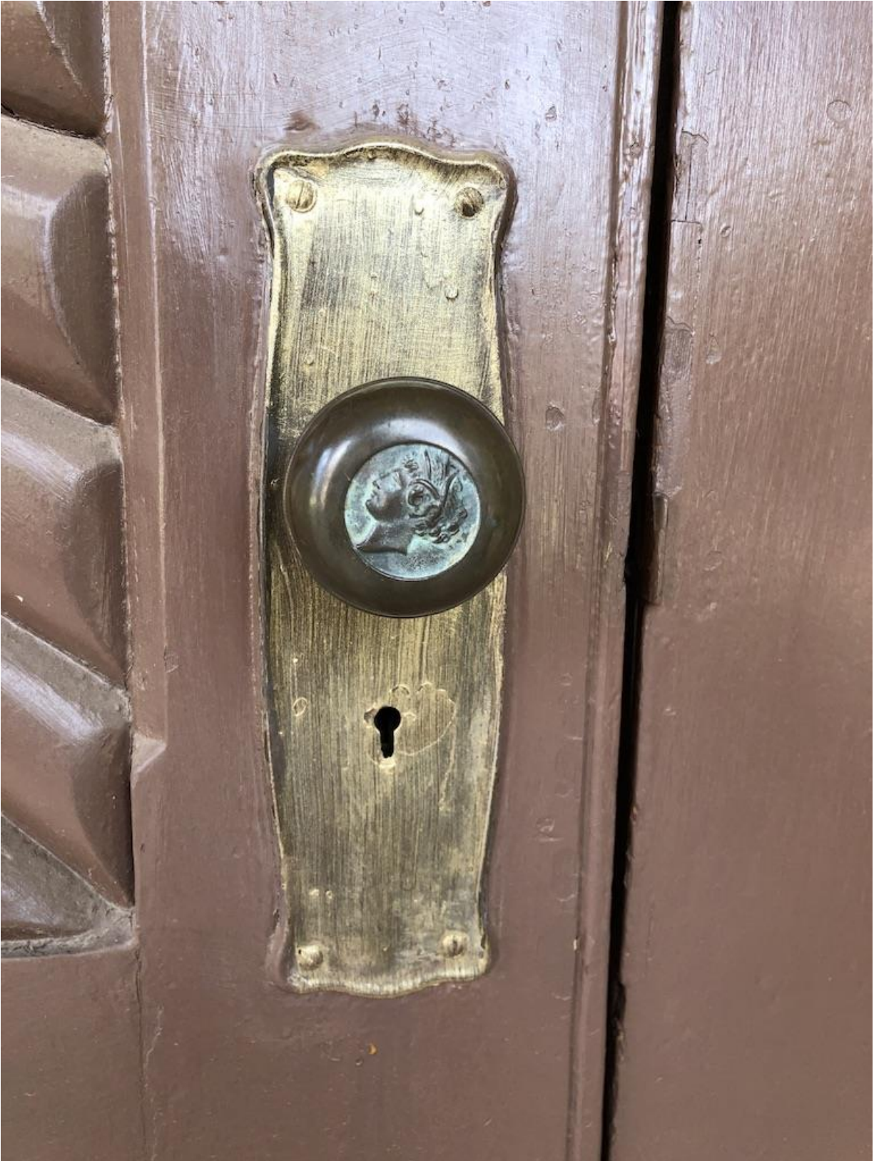
Photo 12 of 39. Temple Aaron, detail of doorknob with cast Liberty head on paired wood entrance doors, east (main) façade.
