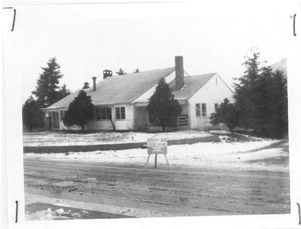
Figure 10. Officers' Club, Building 205, view is north, 1963.
