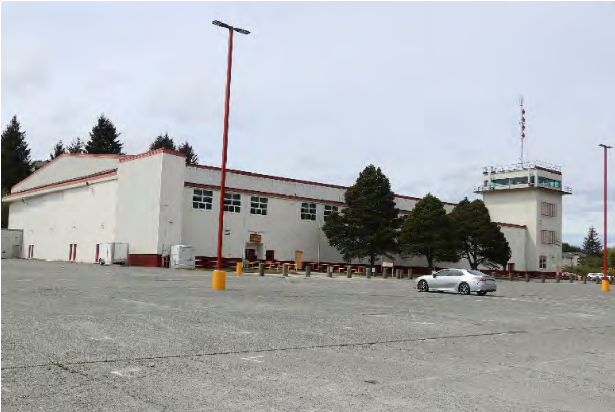
Photo 17 of 43. Seaplane Hangar No. 1, Building 331, view is northwest, May 2022.
