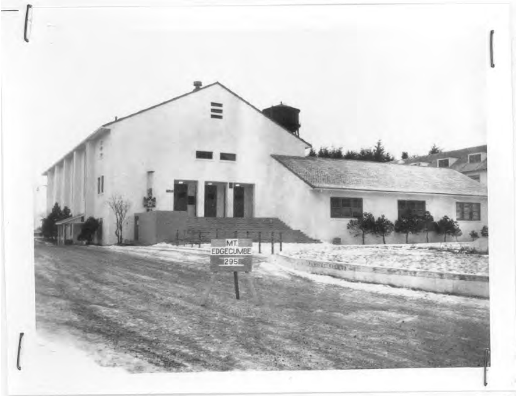
Figure 14. Enlisted Men's Recreation Facility, Building 295, view is south, 1963.
