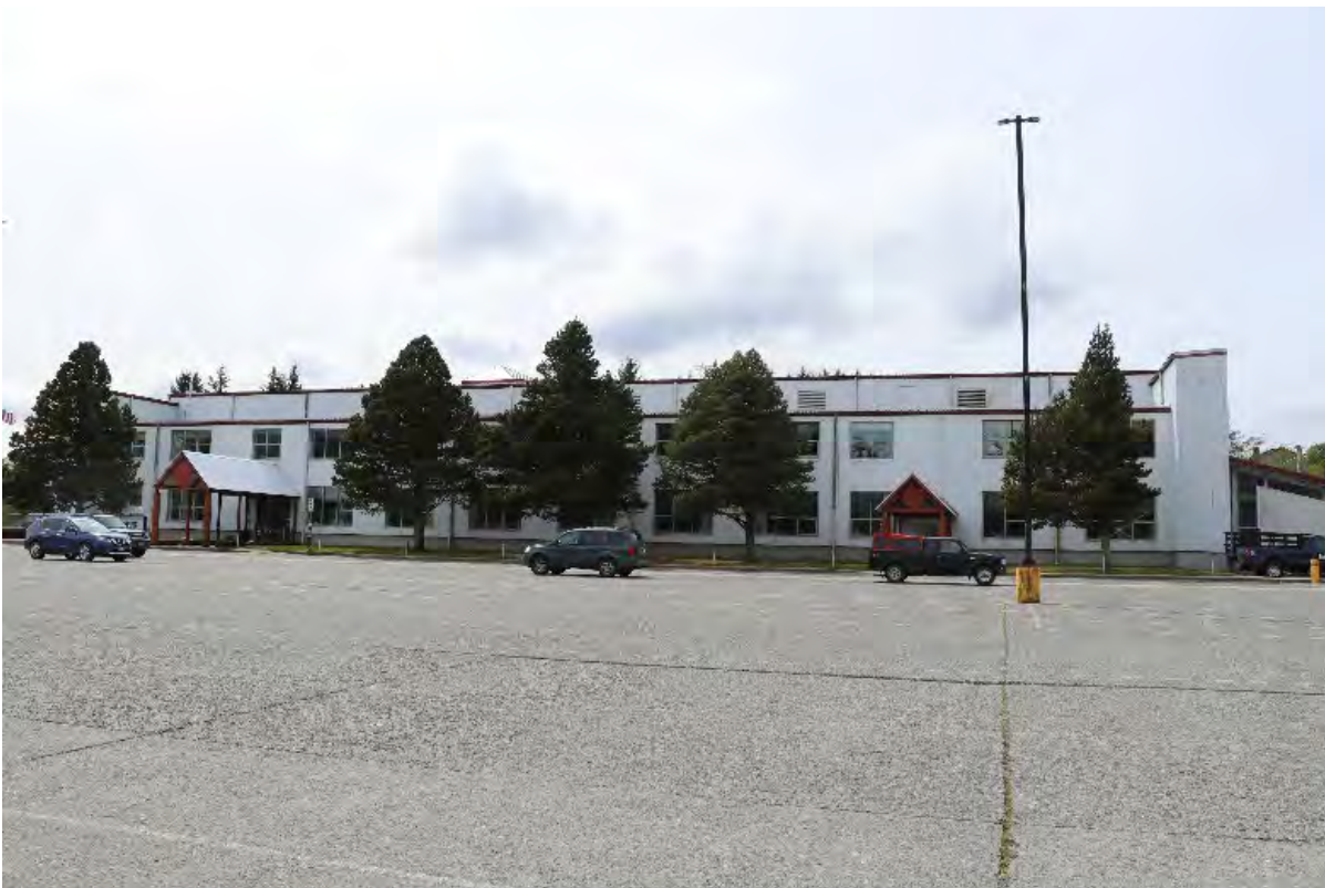
Photo 16 of 43. Seaplane Hangar No. 2, Building 332, view is southwest, May 2022.
