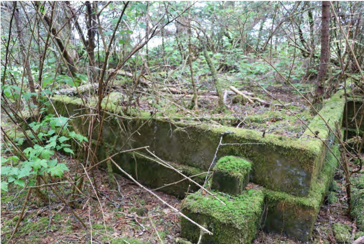
Photo 37 of 43. Foundation on Kirushkin Island, view is southwest, May 2022.
