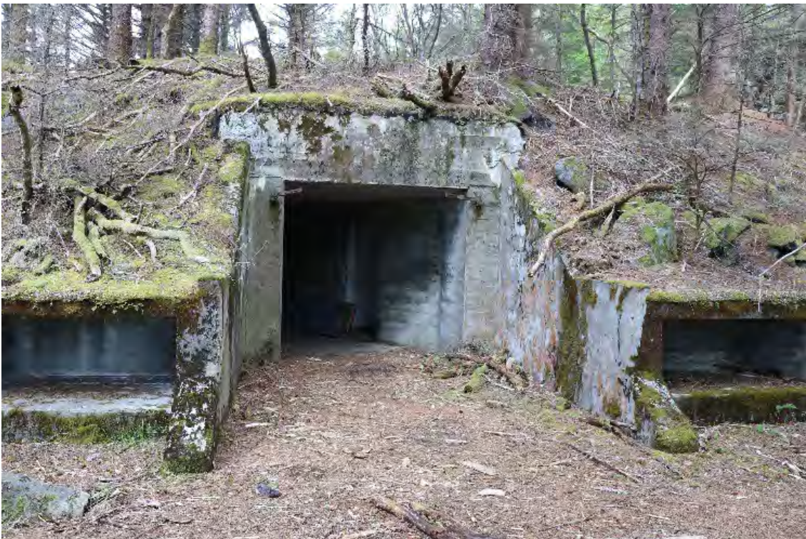
Photo 39 of 43. Battery Emplacement No. 292 Bunker, entrance, view is southwest, May 2022.
