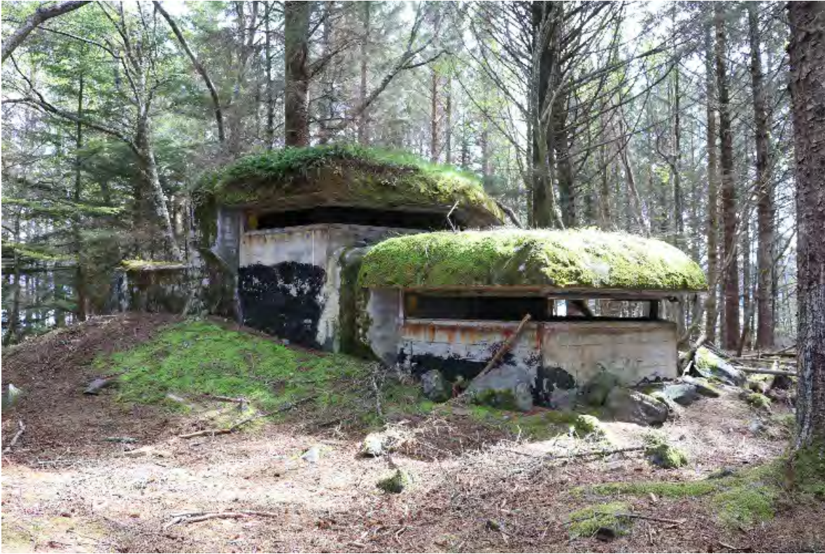
Photo 40 of 43. Battery Emplacement No. 292 Bunker, Command Post, view is east, May 2022.
