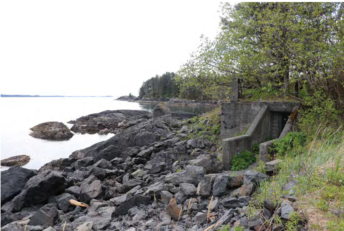
Photo 35 of 43. Meteorological Station (MET) on south side of Sasedni Island, view is south, May 2022.
