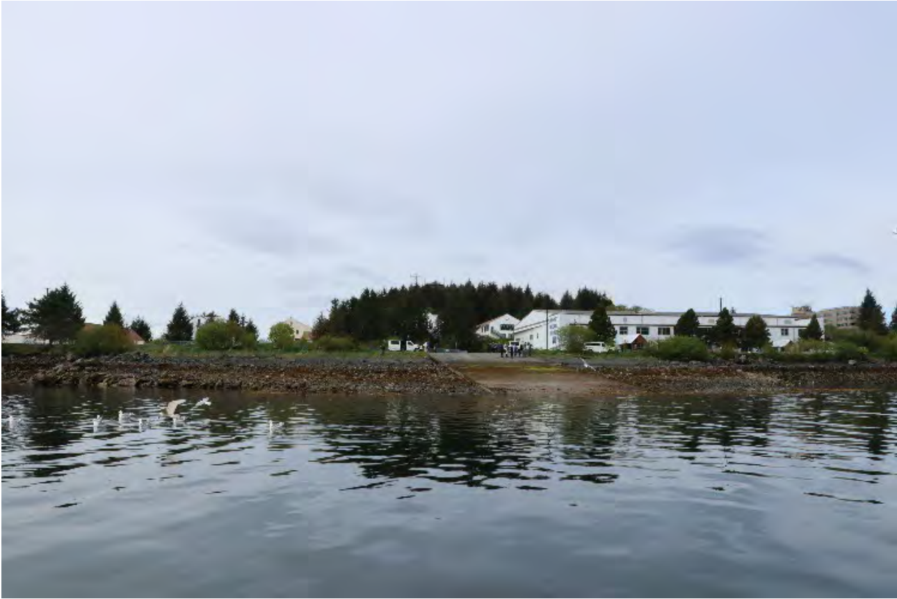
Photo 19 of 43. Seaplane Ramp No. 2 with Seaplane Hangar No. 2 in the background, view is southwest, May 2022.
