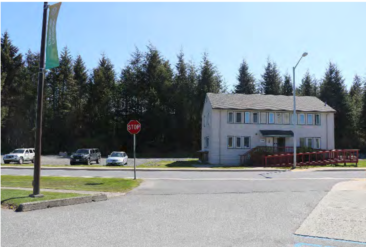
Photo 2 of 43. Typical Married Officers' Quarters duplex, Building 210, view is south, May 2022.
