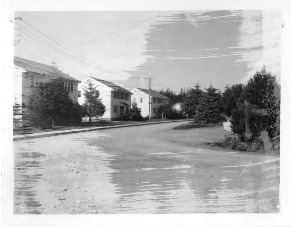
Figure 6. Married Officers' Quarters, Buildings 210, 209 and 208, view is west, 1963.
