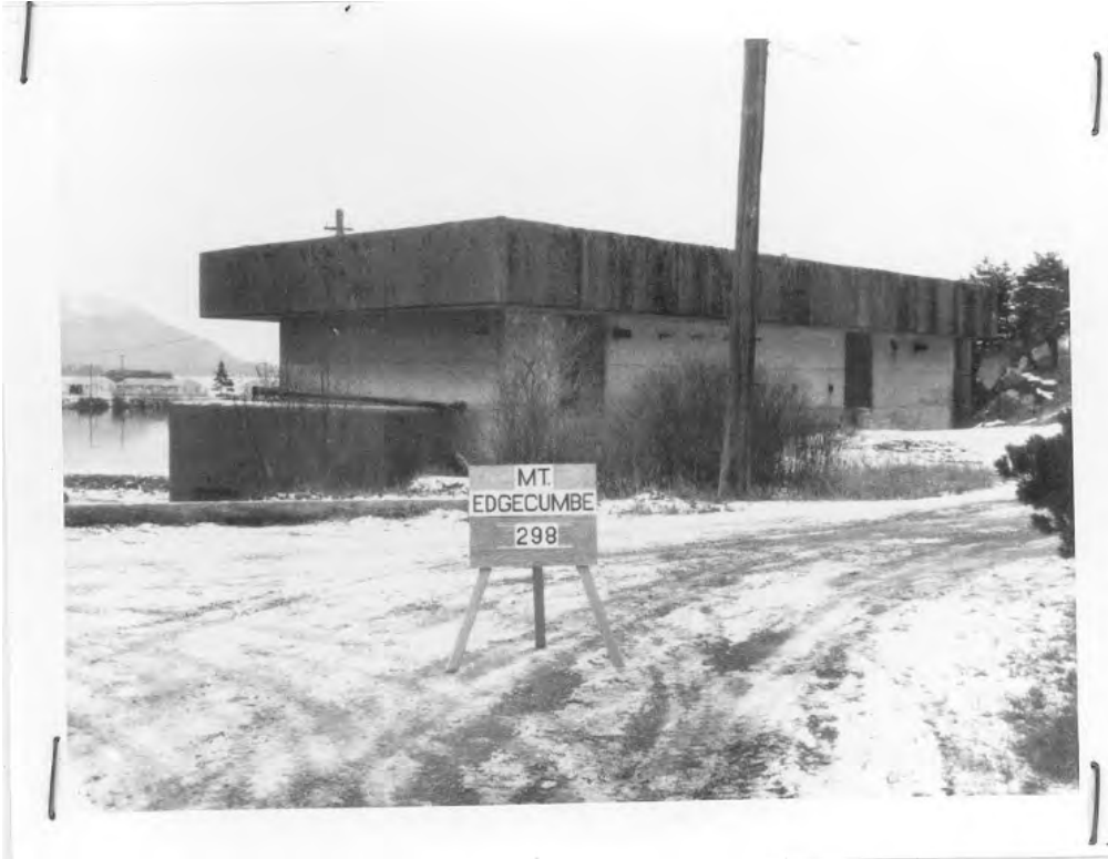
Figure 18. Bomb Proof Communications Center, Building 298, view is southwest, 1963.
