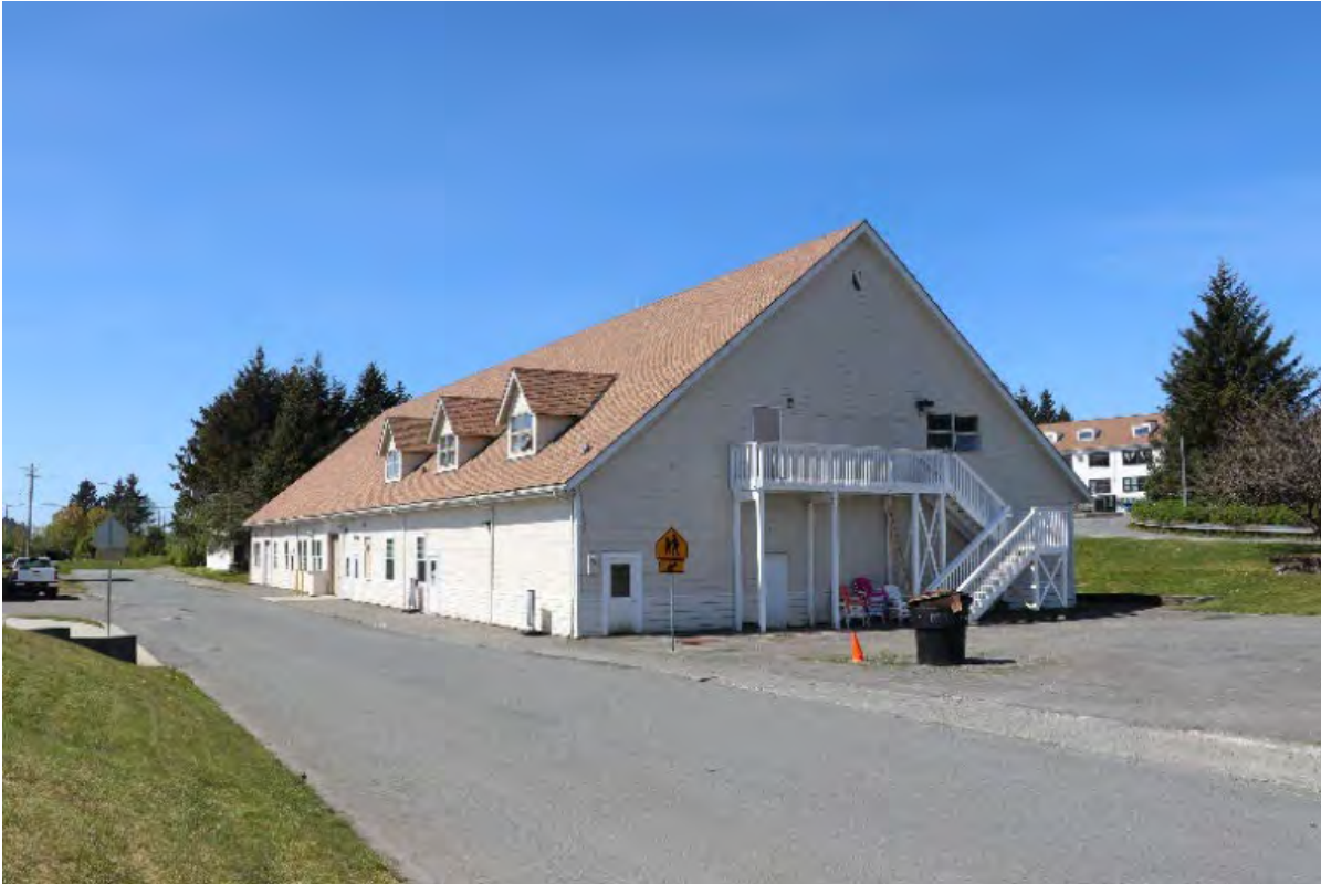
Photo 11 of 43. Commissary, Cold Storage, and Laundry Building, Building 299, view is southwest, May 2022.
