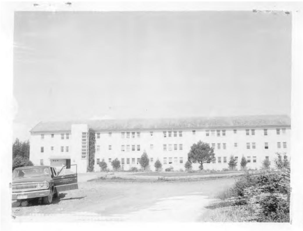
Figure 11. Bachelor Officers' Quarters, Building 212, view is northwest, 1963.
