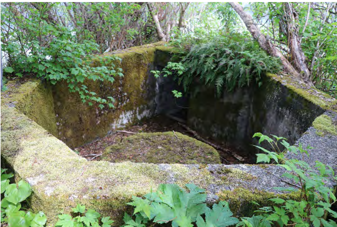
Photo 31 of 43. Mount on top of the Gold Island Bunker, view is east, May 2022. Note that the shape and size of the structure is likely to be an instrument mount rather than a gun emplacement.
