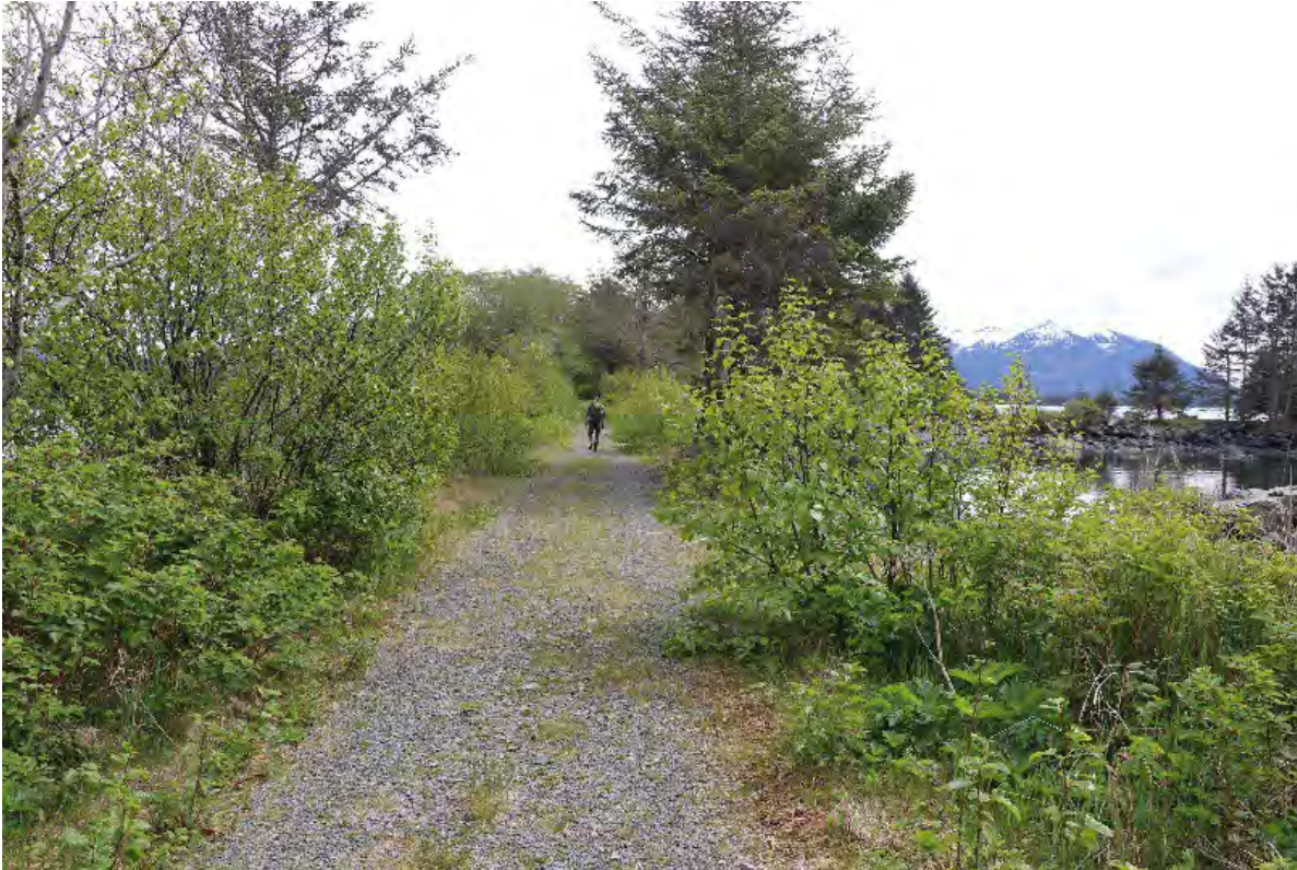
Photo 23 of 43. Causeway between Gold Island and Virublennoi Island, view is southeast, May 2022. Note gravel placed over armor rock on causeway as part of stabilization and rehabilitation efforts.
