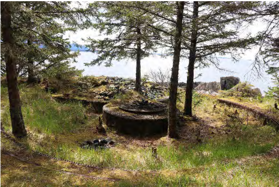
Photo 41 of 43. One of the two 155mm gun emplacements (Panama Mount) that are a part of Battery Emplacement No. 292 Bunker, view is southwest, May 2022.
