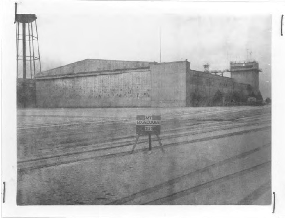
Figure 20. Seaplane Hangar 1, Building 331, view is northwest, 1963.
