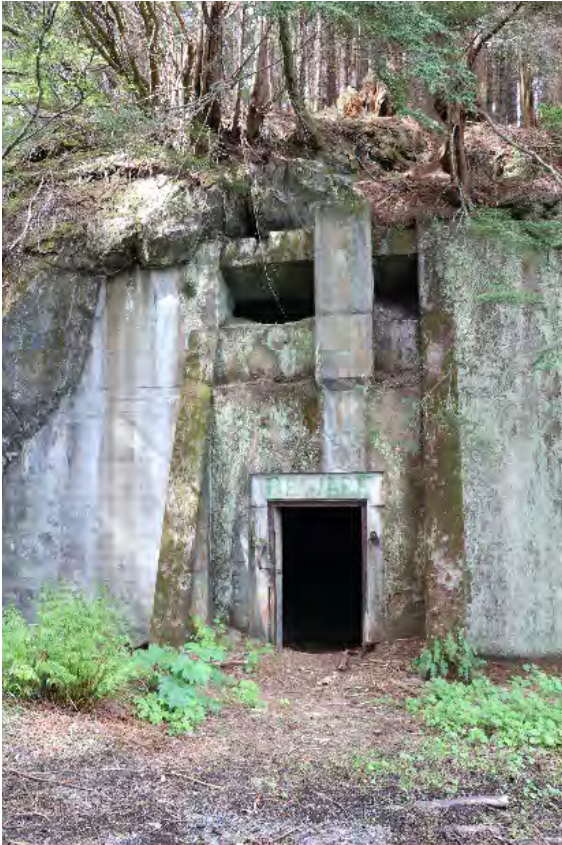
Photo 42 of 43. Entrance to Ammunition Bunker, view is northwest, May 2022.
