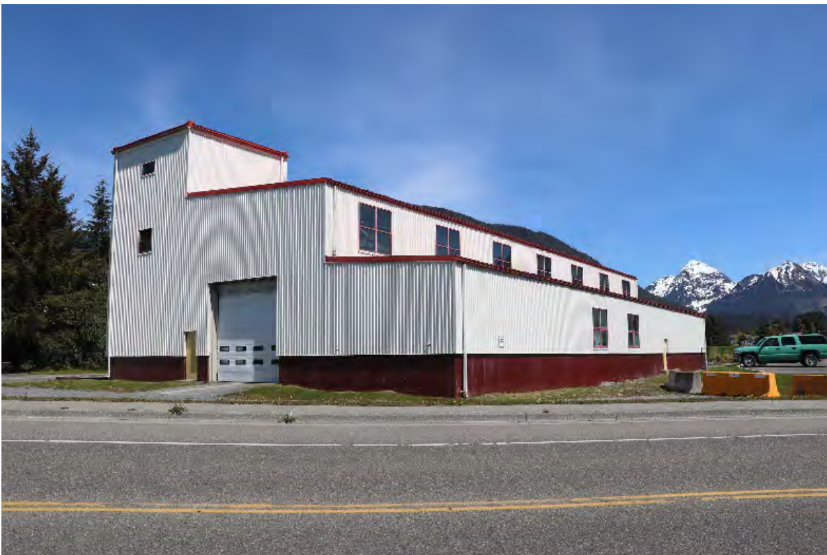
Photo 12 of 43. Torpedo Shed, Garage and Shop, Building 301, view is northeast, May 2022.
