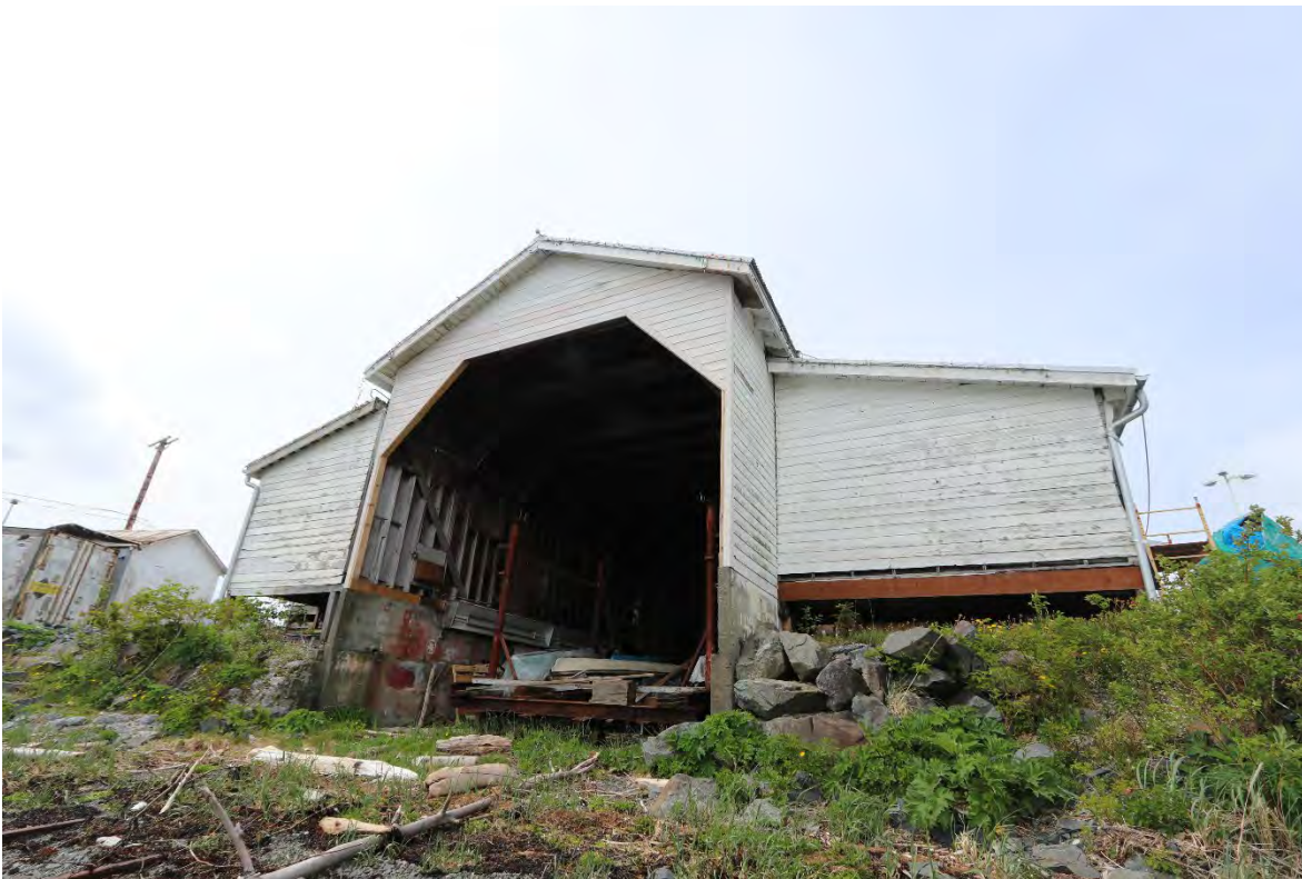
Photo 14 of 43. Boathouse, Building 309, view is southwest towards the opening, May 2022.
