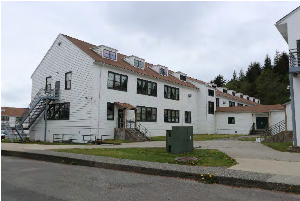
Photo 8 of 43. Enlisted Men’s Barracks, Building 293, view is southwest, May 2022.
