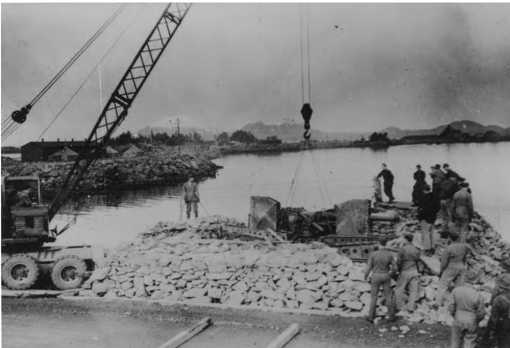
Figure 27. Crane lowering a 3-inch AA gun into its emplacement on Nevski Island. Note that the causeway is in the background, ca. 1942, view is west.
