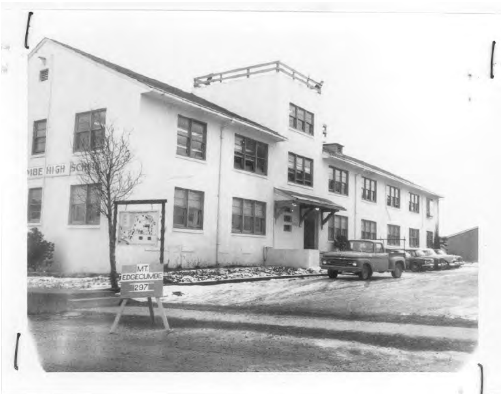
Figure 15. Administration and Operations Building, Building 297, view is southwest, 1963.
