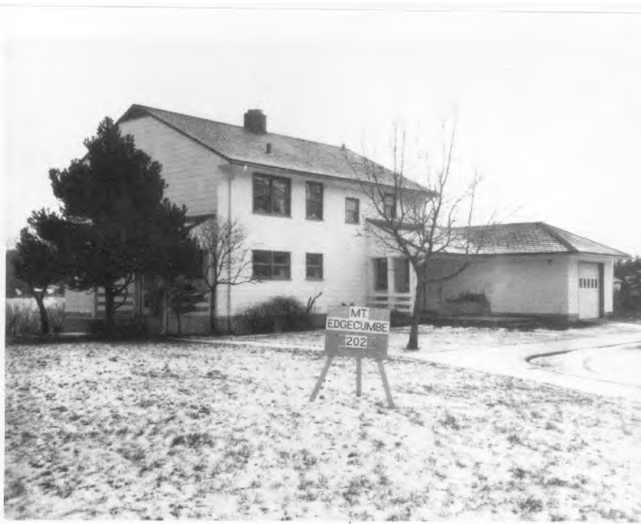
Figure 9. Commanding Officers' Quarters, Building 202, view is northeast, 1963.
