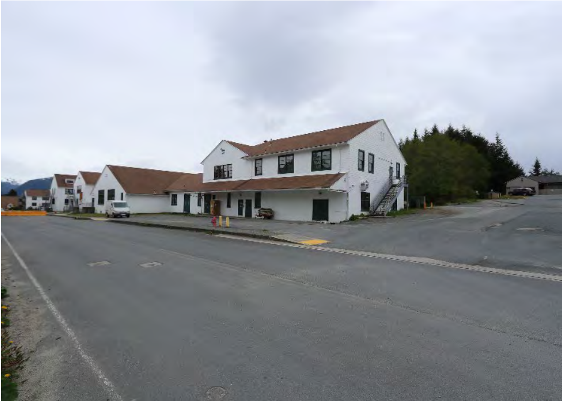
Photo 7 of 43. Mess Hall and Bakery (right), Enlisted Men’s Barracks (center and left), Buildings 290, 292 and 293, respectively. View is southwest, May 2022.
