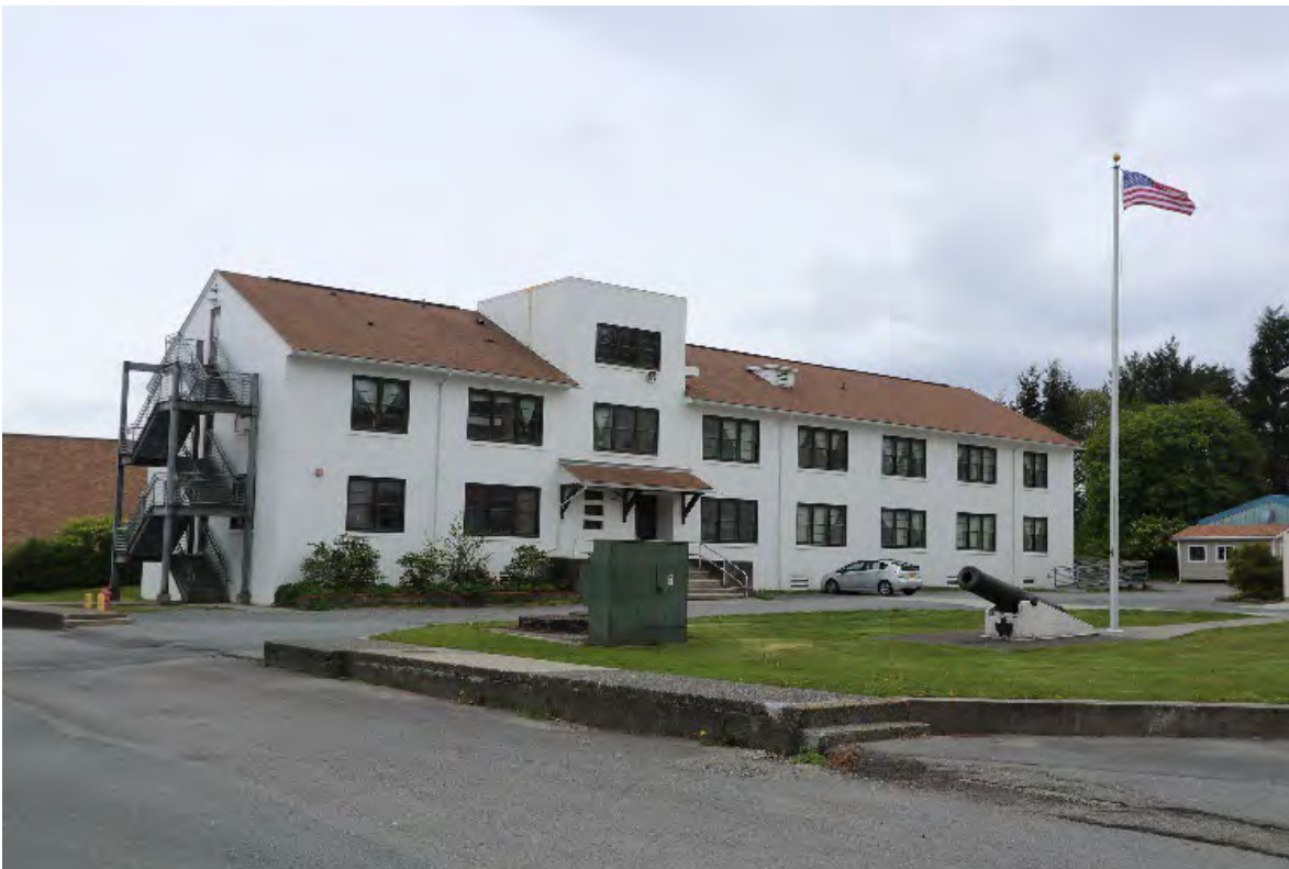
Photo 10 of 43. Administration and Operations Building, Building 297, view is southeast, May 2022.
