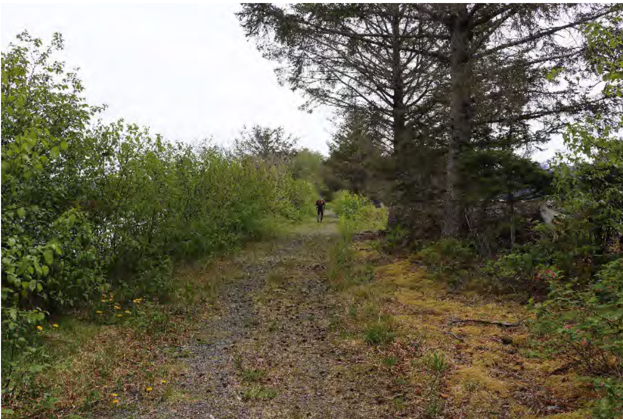
Photo 24 of 43. Causeway between Sasedni Island and Virublennoi Island, view is southeast, May 2022. Note gravel placed over armor rock on causeway as part of stabilization and rehabilitation efforts.
