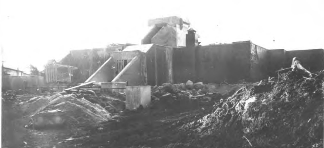
Figure 29. Battery Emplacement No. 292 (Fort Rousseau) under construction, ca. 1942. Rear of battery, entrance in center, Command Post on top, view is south.
