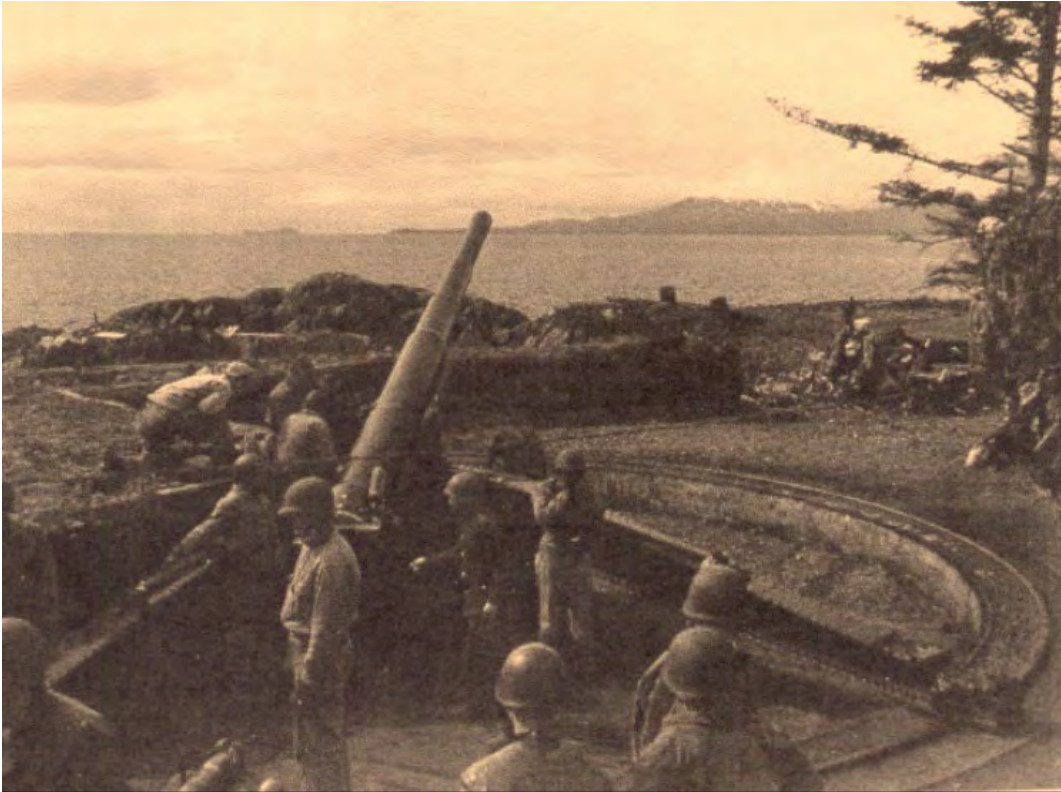
Figure 31. Battery Emplacement No. 292, with 155 mm gun, ca. 1942. View is southwest.
