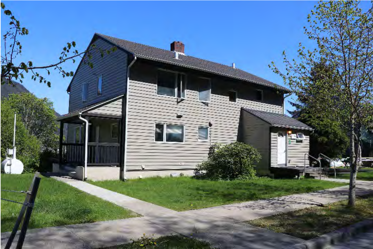
Photo 3 of 43. Typical Senior Officer's Quarters single family home, Building 203, view is north, May 2022.
