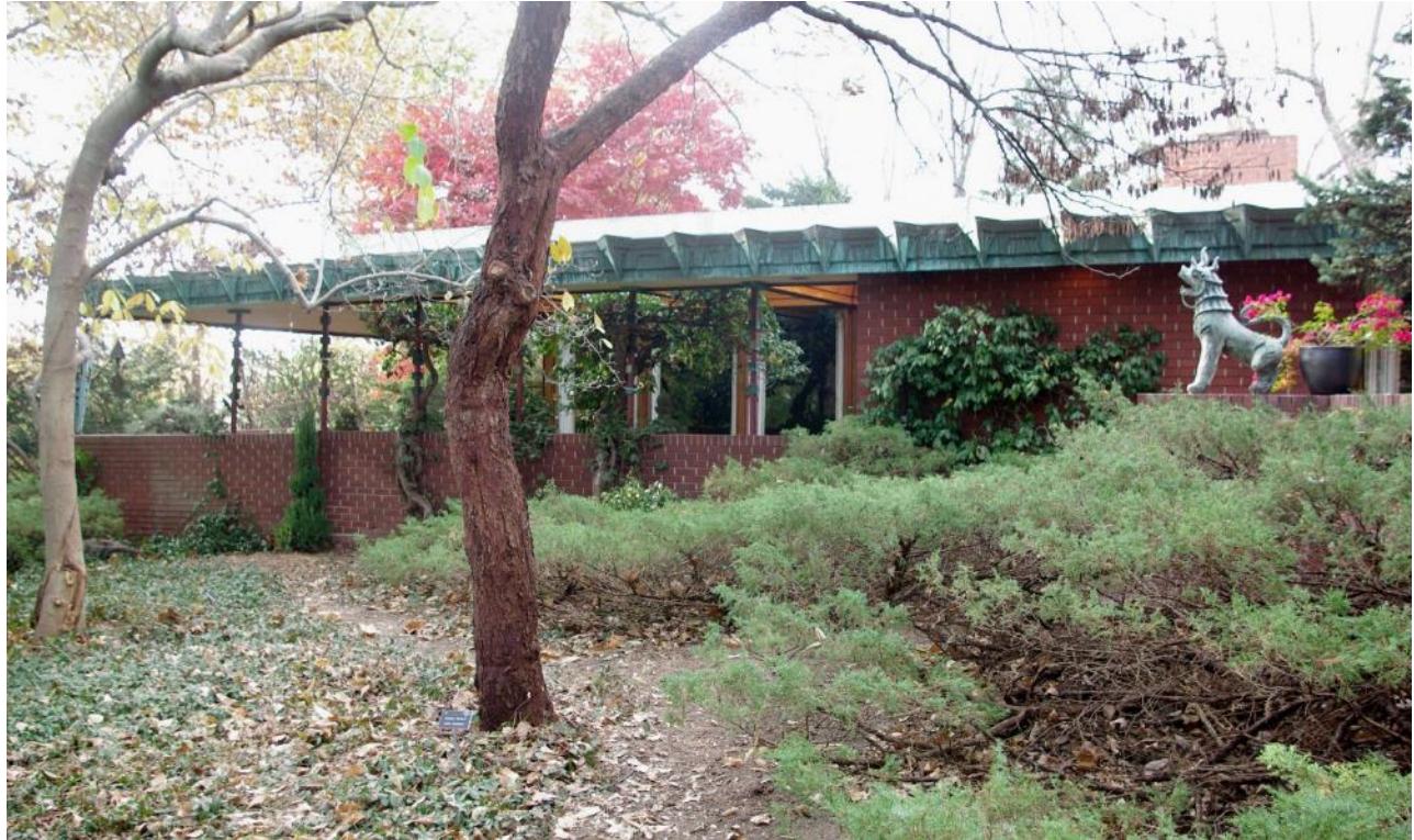
Fig. 2 East, northeast elevation, Camille B. Fife, Photographer 2011.
