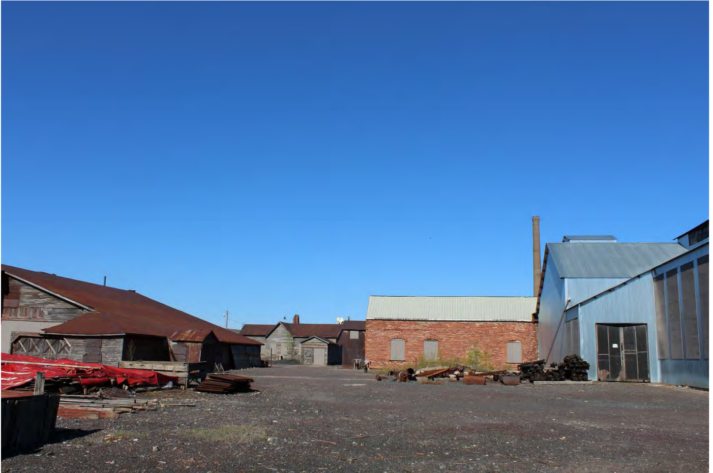
Quincy Smelting Works Landscape Character Area 4. Left to right: Dockside Warehouse (MAP ID# 178), Assay Office (MAP ID# 176), Scale House (MAP ID# 177), and Casting Plant (MAP ID# 171).
