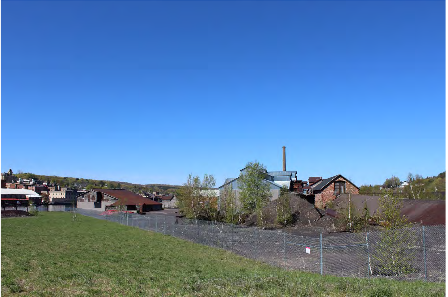
Quincy Smelting Works Landscape Character Area 4. Left to right: Dockside Warehouse (MAP ID# 178), Assay Office (MAP ID# 176), Scale House (MAP ID# 177), Casting Plant (MAP ID# 171), East Slag Pile and Steel Trestle, and Mineral House (MAP ID# 169). Boiler Stack (MAP ID# 156) in background.
