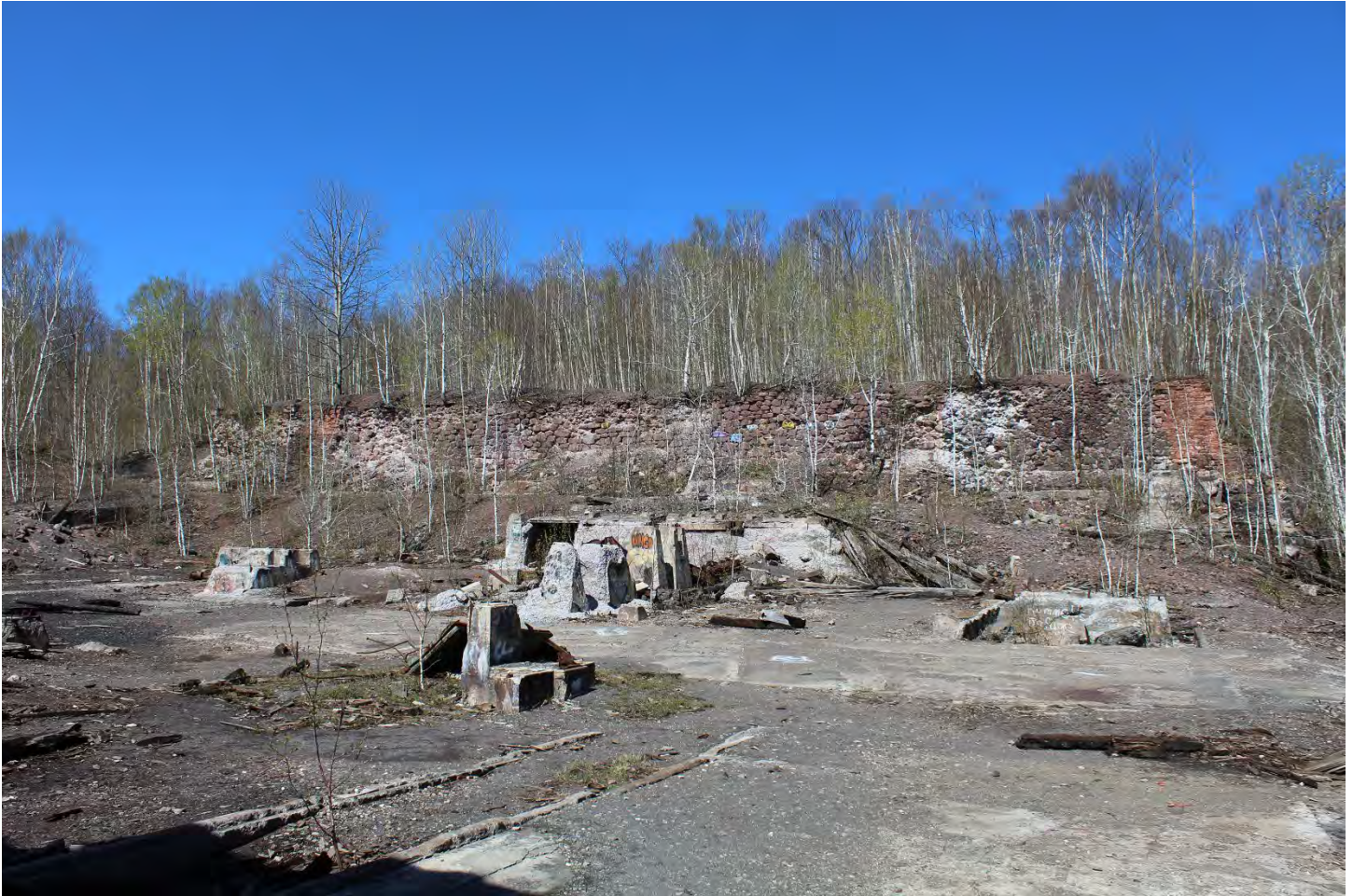
Quincy Stamp Mill, Landscape Character Area 7. Steam Turbine Building Ruin (MAP ID# 202).
