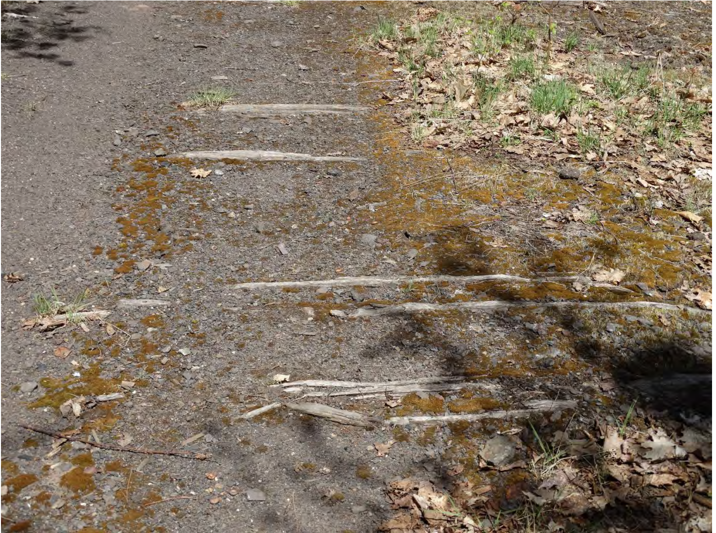
Quincy and Torch Lake Railroad Corridor, Landscape Character Area 6. Detail of the railroad tie remnants.
