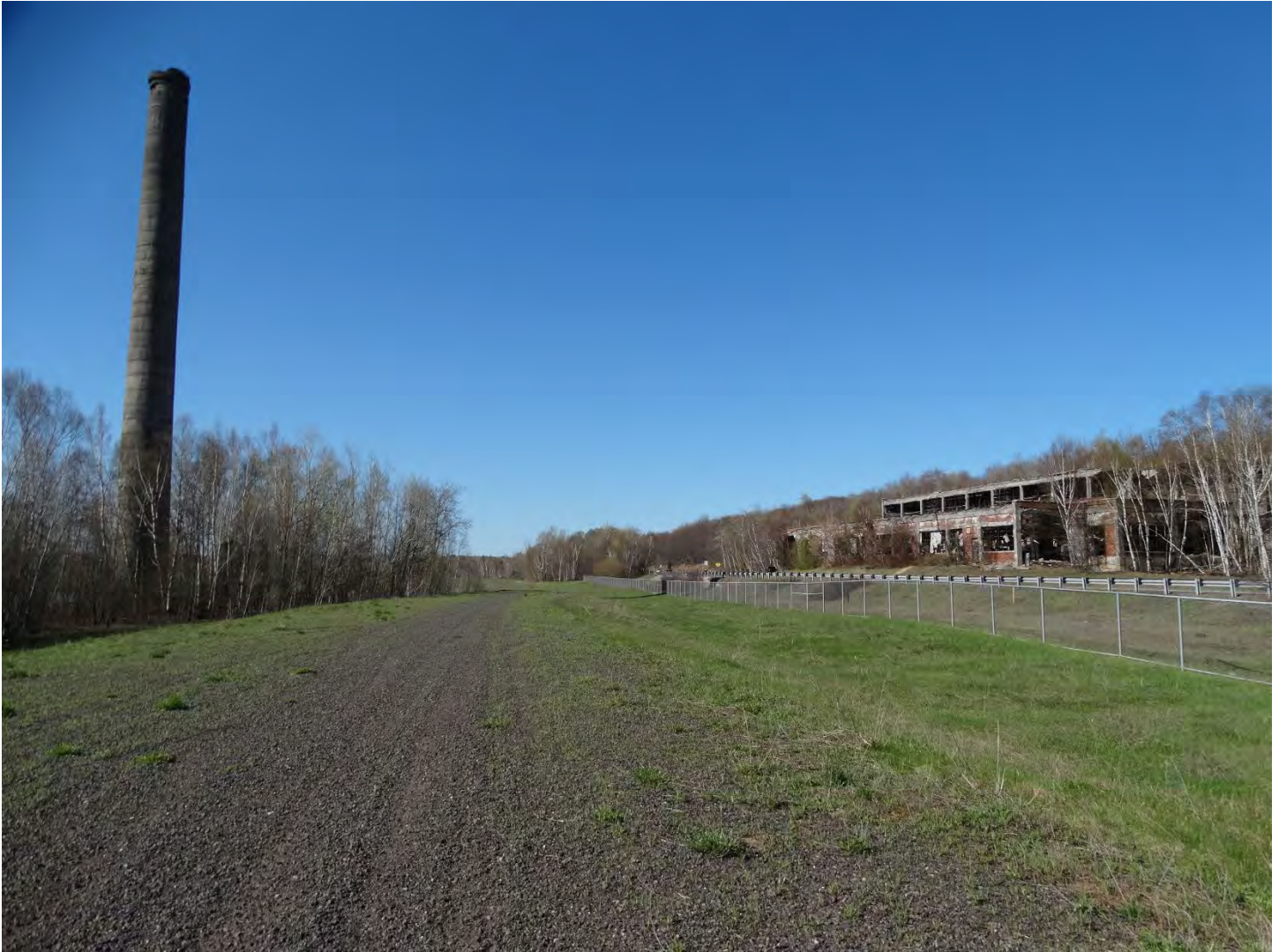
Quincy Stamp Mill, Landscape Character Area 7. Quincy Stamp Mill No. 1 (MAP ID# 203) area along the Quincy and Torch Lake Railroad Corridor; the Boilerhouse Smokestack for Stamp Mill No. 1 (MAP ID# 204) on the left.
