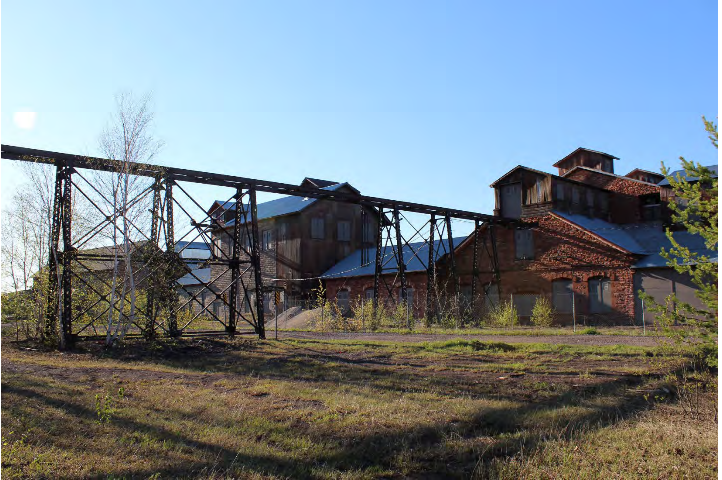
Quincy Smelting Works Landscape Character Area 4. Steel Trestle (MAP ID# 151) in foreground; right to left: Cupola Furnace Building (MAP ID# 159), Pump House Addition (MAP ID# 162), Crushing Plant (MAP ID# 163), Briquetting Plant (MAP ID# 165) and Mineral House (MAP ID# 169).
