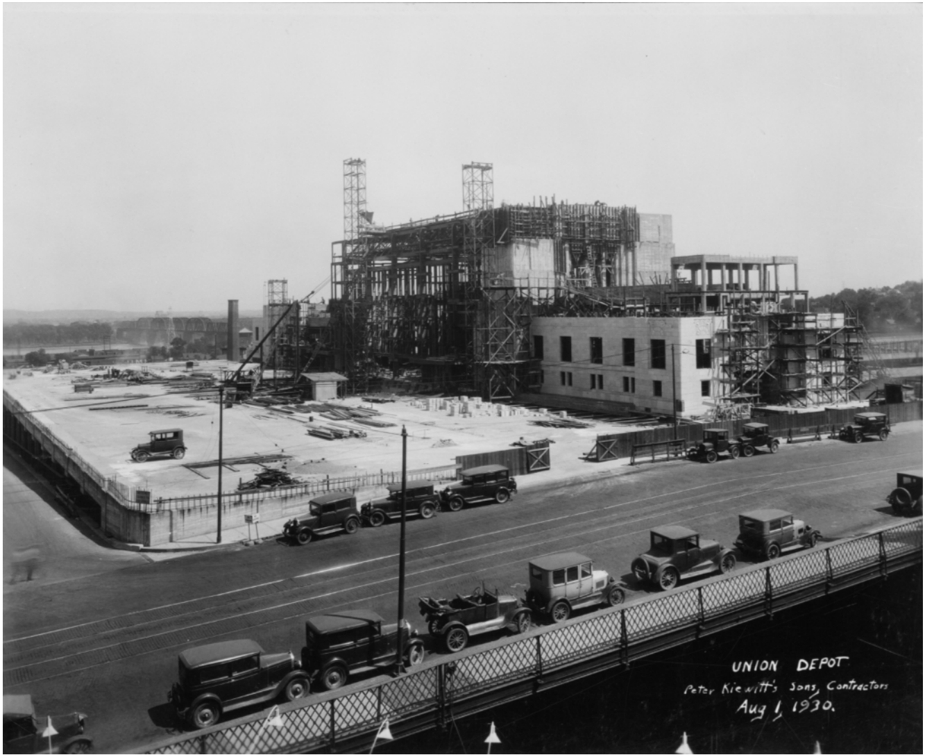
THE 1931 OMAHA UNION STATION UNDER CONSTRUCTION, AUGUST 1, 1930
