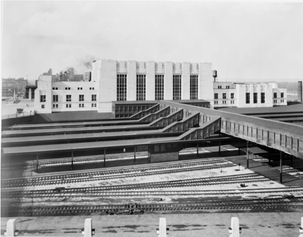
OMAHA UNION STATION, SOUTH WALL AND CONCOURSE, Aug. 18, 1932
