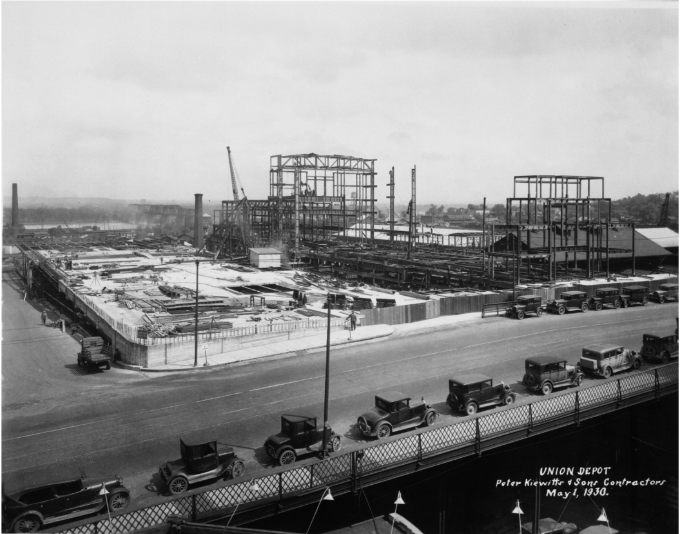
THE 1931 OMAHA UNION STATION UNDER CONSTRUCTION, MAY 1, 1930
