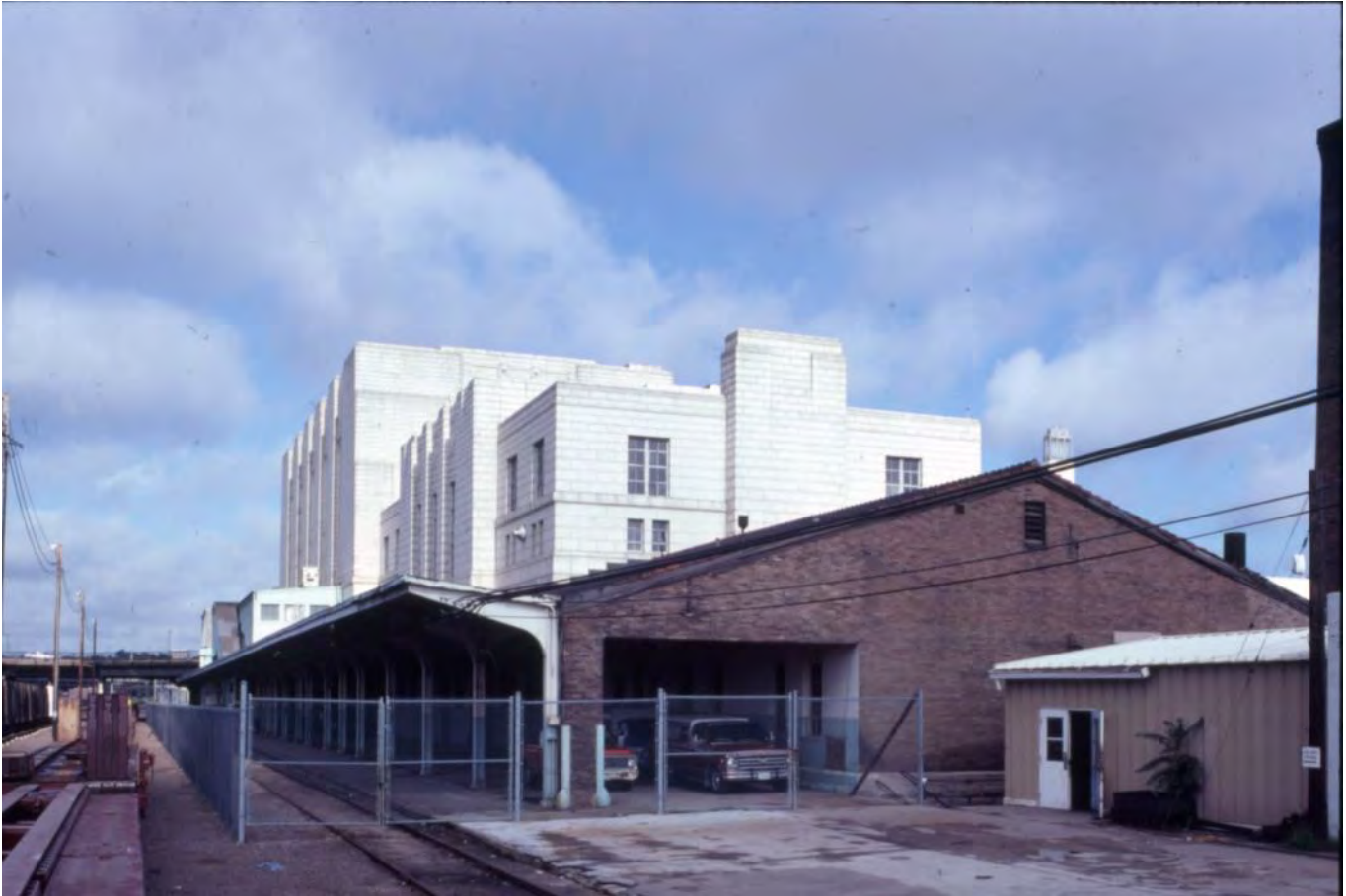
OMAHA UNION STATION, EAST WALL OF MAIN BUILDING AND 1899 BRICK BOILER HOUSE, ca. 1975
