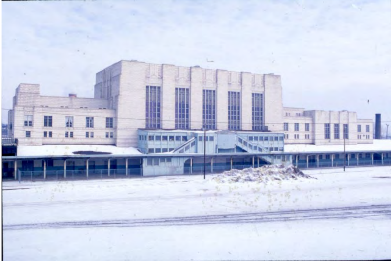
OMAHA UNION STATION, SOUTH WALL, ca. 1975
